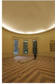
M2Hi\_j0007 8/18/2005 1445. Oval Office Restoration. Sanding and vacuuming the floor.
