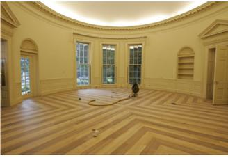
M2Hi\_j0003 8/18/2005 1445. Oval Office Restoration. Sanding and vacuuming the floor.
