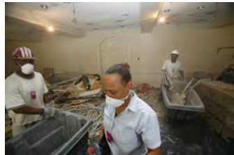
F081506PM-0004 [2018-0227-F_M1Hi_j0140_2.JPG] 8/15/2006 Press Briefing Room Renovations
