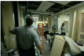
F062707CG-0045 [2018-0227-F_M1Hi_j0037_3.JPG] 6/27/2007 Work continues on the press briefing room
