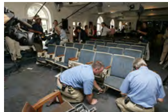
F080306PM-0015 [2018-0227-F_M1Hi_j0107.JPG] 8/3/2006 Clearing out Press Briefing room for renovations.
