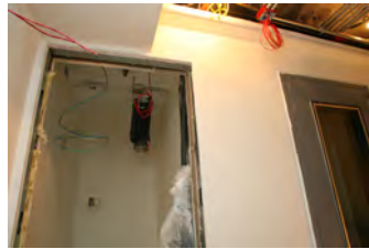
F051607SC-0119 [2018-0227-F_M1Hi_j0068_1.JPG] 5/16/2007 Press Briefing Room Renovations
