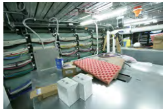
F062007CG-0011 [2018-0227-F_M2Hi_j0192.JPG] 6/20/2007 Work continues on the press briefing room
