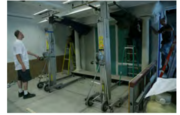
F062007CG-0041 [2018-0227-F_M2Hi_j0252.JPG] 6/20/2007 Work continues on the press briefing room
