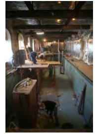
F120206PM-0032 [2018-0227-F_M1Hi_j0206_3.JPG] 12/2/2006 Press Briefing room renovations.
