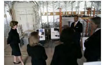
P040207SC-0049 [2018-0227-F_M1Hi_j0214_4.JPG] 4/2/2007 LB. The Brady Press Room During Renovations.
