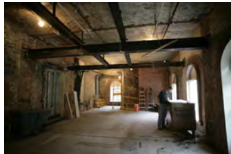
F101906PM-004 [2018-0227-F_M1Hi_j0207_1.JPG] 10/19/2006 Renovations to the Press Briefing room
