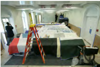
F062707CG-0001 [2018-0227-F_M1Hi_j0097_2.JPG] 6/27/2007 Work continues on the press briefing room
