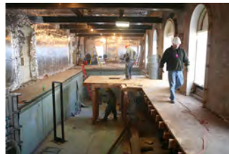
F120206PM-0003 [2018-0227-F_M1Hi_j0148_4.JPG] 12/2/2006 Press Briefing room renovations.
