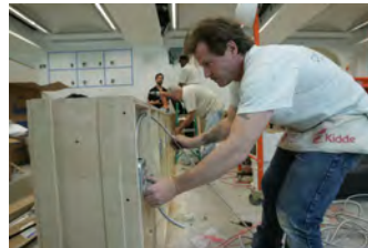
F061507CG-0012 [2018-0227-F_M2Hi_j0179.JPG] 6/15/2007 The Press Briefing Room nears completion
