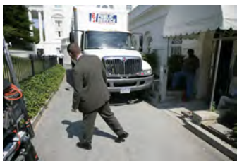
P062107ED-0329 [2018-0227-F_M1Hi_j0030_6.JPG] 6/21/2007 Press Briefing Room Renovations. West Wing.
