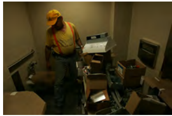
F061507CG-0046 [2018-0227-F_M2Hi_j0247.JPG] 6/15/2007 The Press Briefing Room nears completion
