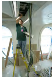
F061507CG-0011 [2018-0227-F_M2Hi_j0177.JPG] 6/15/2007 The Press Briefing Room nears completion
