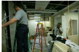
F062707CG-0043 [2018-0227-F_M1Hi_j0029_2.JPG] 6/27/2007 Work continues on the press briefing room
