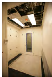
F061207DB-0001 [2018-0227-F_M1Hi_j0007_2.JPG] 6/12/2007 Brady Press Briefing Room Renovations
