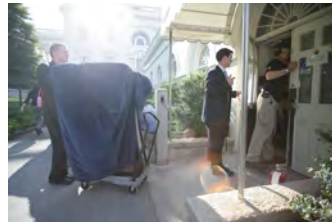
P062207ED-0026 [2018-0227-F_M1Hi_j0039_3.JPG] 6/22/2007 Press Briefing Room rennovations
