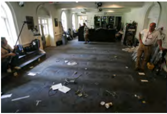
F080306PM-0180 [2018-0227-F_M1Hi_j0182.JPG] 8/3/2006 Clearing out Press Briefing room for renovations.
