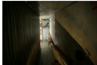
F121506PM-0020 [2018-0227-F_M1Hi_j0143_1.JPG] 12/15/2006 Press Briefing room renovations
