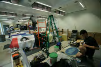
F062907CG-0033 [2018-0227-F_M1Hi_j0036_5.JPG] 6/29/2007 Work nears completion on the press briefing room, Friday June 29, 2007.
