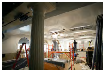
P062107ED-0227 [2018-0227-F_M1Hi_j0081_4.JPG] 6/21/2007 Press Briefing Room Renovations. West Wing.
