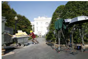
F081506PM-0049 [2018-0227-F_M1Hi_j0230_1.JPG] 8/15/2006 Press Briefing Room Renovations
