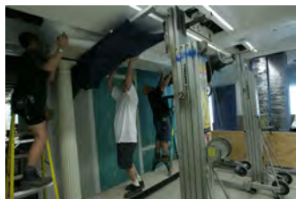
F062007CG-0031 [2018-0227-F_M2Hi_j0232.JPG] 6/20/2007 Work continues on the press briefing room
