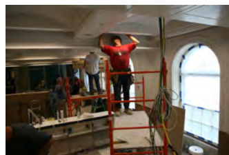
P061907DG-0206 [2018-0227-F_M1Hi_j0171_2.JPG] 6/19/2007 James S. Brady Press Briefing Room renovation
