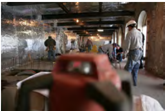
F010907PM-0015 [2018-0227-F_M1Hi_j0144_4.JPG] 1/9/2007 Press Briefing Room Renovations
