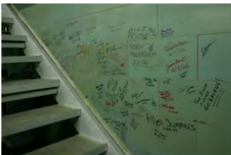
F062007CG-0006 [2018-0227-F_M2Hi_j0182.JPG] 6/20/2007 Work continues on the press briefing room
