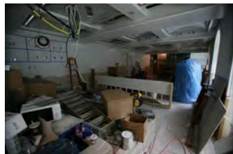
F061207DB-0010 [2018-0227-F_M1Hi_j0077_1.JPG] 6/12/2007 Brady Press Briefing Room Renovations
