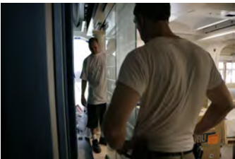
P062107ED-0261 [2018-0227-F_M1Hi_j0149_6.JPG] 6/21/2007 Press Briefing Room Renovations. West Wing.
