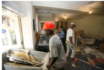
F081506PM-0045 [2018-0227-F_M1Hi_j0222_1.JPG] 8/15/2006 Press Briefing Room Renovations
