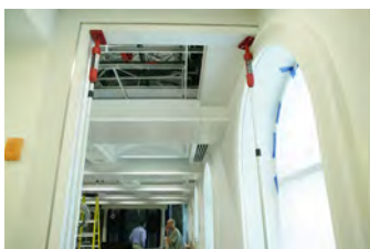
F062207CG-0018 [2018-0227-F_M1Hi_j0076_7.JPG] 6/22/2007 Work continues on the press briefing room
