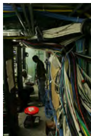
F062807CG-0036 [2018-0227-F_M1Hi_j0149_3.JPG] 6/28/2007 Work continues on the press briefing room
