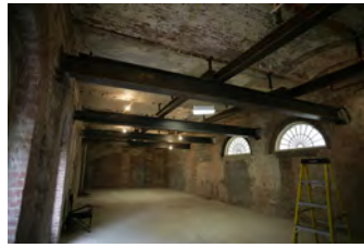
F101906PM-016 [2018-0227-F_M1Hi_j0255_1.JPG] 10/19/2006 Renovations to the Press Briefing room
