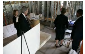
P040207SC-0057 [2018-0227-F_M1Hi_j0007_1.JPG] 4/2/2007 LB. The Brady Press Room During Renovations.
