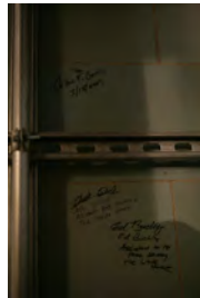
F051607SC-0015 [2018-0227-F_M1Hi_j0062_1.JPG] 5/16/2007 Press Briefing Room Renovations
