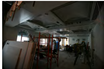
F061207DB-0029 [2018-0227-F_M1Hi_j0198_5.JPG] 6/12/2007 Brady Press Briefing Room Renovations
