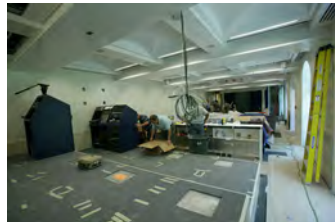
F062707CG-0022 [2018-0227-F_M1Hi_j0187_3.JPG] 6/27/2007 Work continues on the press briefing room
