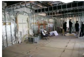
P040207SC-0032 [2018-0227-F_M1Hi_j0084_1.JPG] 4/2/2007 LB. The Brady Press Room During Renovations.
