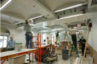
F061507CG-0006 [2018-0227-F_M2Hi_j0167.JPG] 6/15/2007 The Press Briefing Room nears completion
