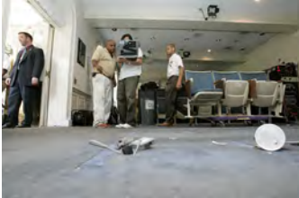
F080306PM-0164 [2018-0227-F_M1Hi_j0150.JPG] 8/3/2006 Clearing out Press Briefing room for renovations.
