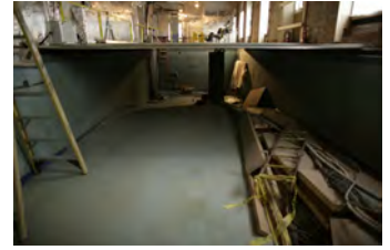
F121506PM-0013 [2018-0227-F_M1Hi_j0129_1.JPG] 12/15/2006 Press Briefing room renovations
