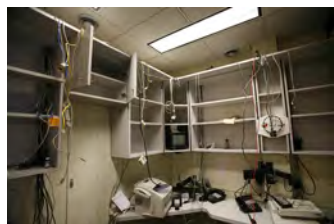
F080406PM-0039 [2018-0227-F_M1Hi_j0214.JPG] 8/4/2006 Clearing out Press Briefing room for renovations.
