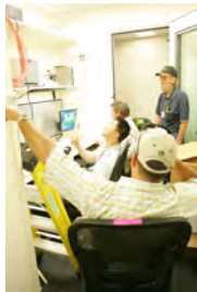
F070207CG-0018 [2018-0227-F_M1Hi_j0115_4.JPG] 7/2/2007 Work nears completion on the press briefing room
