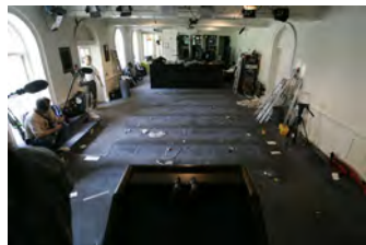
F080306PM-0189 [2018-0227-F_M1Hi_j0200.JPG] 8/3/2006 Clearing out Press Briefing room for renovations.
