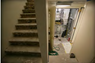
F061207DB-0044 [2018-0227-F_M1Hi_j0040_3.JPG] 6/12/2007 Brady Press Briefing Room Renovations
