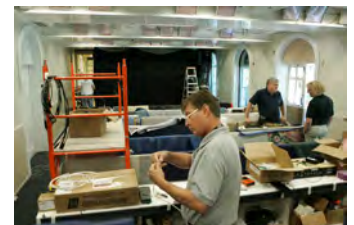
F070207CG-0003 [2018-0227-F_M1Hi_j0029_3.JPG] 7/2/2007 Work nears completion on the press briefing room
