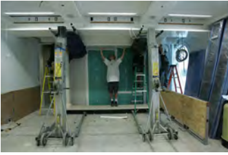
F062007CG-0038 [2018-0227-F_M2Hi_j0246.JPG] 6/20/2007 Work continues on the press briefing room
