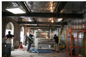
F012507PM-0031 [2018-0227-F_M1Hi_j0075.JPG] 1/25/2007 Press Briefing room renovations.
