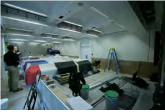
F062707CG-0053 [2018-0227-F_M1Hi_j0069_2.JPG] 6/27/2007 Work continues on the press briefing room
