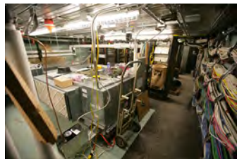
F061207DB-0037 [2018-0227-F_M1Hi_j0253_3.JPG] 6/12/2007 Brady Press Briefing Room Renovations
