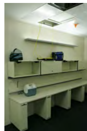
F062907CG-0007 [2018-0227-F_M1Hi_j0239_5.JPG] 6/29/2007 Work nears completion on the press briefing room, Friday June 29, 2007.
