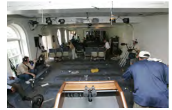
F080306PM-0163 [2018-0227-F_M1Hi_j0148.JPG] 8/3/2006 Clearing out Press Briefing room for renovations.
