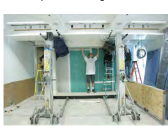
F062007CG-0036 [2018-0227-F_M2Hi_j0242.JPG] 6/20/2007 Work continues on the press briefing room
