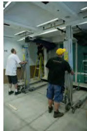
F062007CG-0043 [2018-0227-F_M2Hi_j0001.JPG] 6/20/2007 Work continues on the press briefing room
