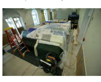
F062707CG-0007 [2018-0227-F_M1Hi_j0121_3.JPG] 6/27/2007 Work continues on the press briefing room
