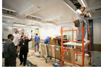
P062107ED-0214 [2018-0227-F_M1Hi_j0055_4.JPG] 6/21/2007 Press Briefing Room Renovations. West Wing.
