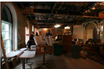
F051607SC-0086 [2018-0227-F_M1Hi_j0002_2.JPG] 5/16/2007 Press Briefing Room Renovations
