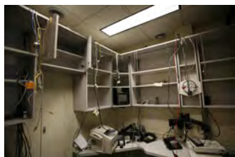
F080406PM-0038 [2018-0227-F_M1Hi_j0212.JPG] 8/4/2006 Clearing out Press Briefing room for renovations.
