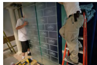
P062107ED-0288 [2018-0227-F_M1Hi_j0203_9.JPG] 6/21/2007 Press Briefing Room Renovations. West Wing.
