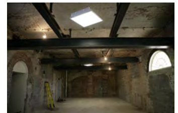
F101806KH-0002 [2018-0227-F_M1Hi_j0148_3.JPG] 10/18/2006 Press Room Renovations
