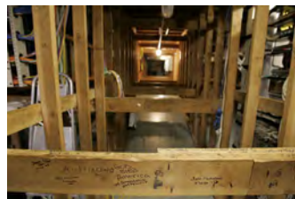
F080306PM-0074 [2018-0227-F_M1Hi_j0225.JPG] 8/3/2006 Clearing out Press Briefing room for renovations.
