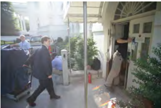
P062207ED-0024 [2018-0227-F_M1Hi_j0069_1.JPG] 6/22/2007 Press Briefing Room rennovations
