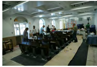
F062207CG-0075 [2018-0227-F_M1Hi_j0190_6.JPG] 6/22/2007 Work continues on the press briefing room
