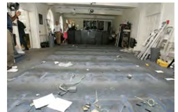
F080306PM-0179 [2018-0227-F_M1Hi_j0180.JPG] 8/3/2006 Clearing out Press Briefing room for renovations.
