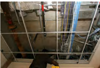
F051607SC-0126 [2018-0227-F_M1Hi_j0082_2.JPG] 5/16/2007 Press Briefing Room Renovations
