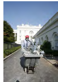
F081506PM-0055 [2018-0227-F_M1Hi_j0242_1.JPG] 8/15/2006 Press Briefing Room Renovations
