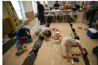
P062107ED-0299 [2018-0227-F_M1Hi_j0225_6.JPG] 6/21/2007 Press Briefing Room Renovations. West Wing.
