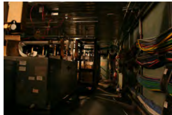
F051607SC-0019 [2018-0227-F_M1Hi_j0082_1.JPG] 5/16/2007 Press Briefing Room Renovations
