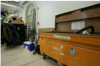
F062007CG-0066 [2018-0227-F_M2Hi_j0047.JPG] 6/20/2007 Work continues on the press briefing room
