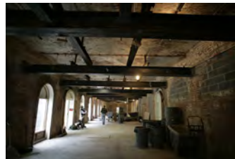
F101906PM-009 [2018-0227-F_M1Hi_j0234_2.JPG] 10/19/2006 Renovations to the Press Briefing room
