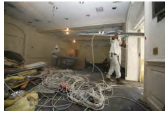
F081506PM-0018 [2018-0227-F_M1Hi_j0168_2.JPG] 8/15/2006 Press Briefing Room Renovations
