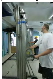
F062007CG-0028 [2018-0227-F_M2Hi_j0226.JPG] 6/20/2007 Work continues on the press briefing room
