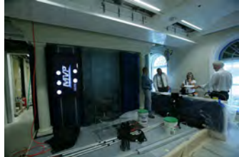
F062707CG-0038 [2018-0227-F_M1Hi_j0009.JPG] 6/27/2007 Work continues on the press briefing room
