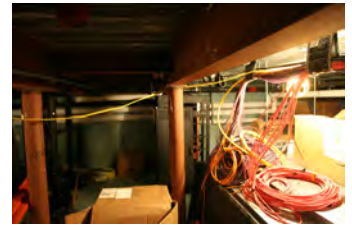
F051607SC-0013 [2018-0227-F_M1Hi_j0054_2.JPG] 5/16/2007 Press Briefing Room Renovations
