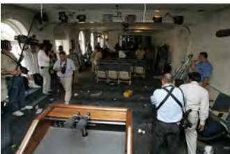
F080306PM-0156 [2018-0227-F_M1Hi_j0134.JPG] 8/3/2006 Clearing out Press Briefing room for renovations.
