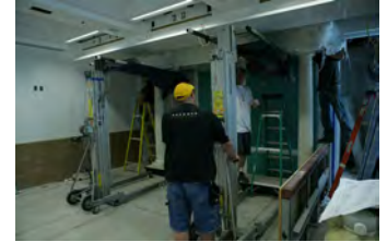
F062007CG-0045 [2018-0227-F_M2Hi_j0005.JPG] 6/20/2007 Work continues on the press briefing room
