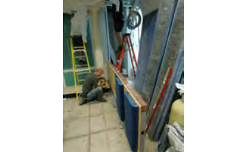
F062007CG-0077 [2018-0227-F_M2Hi_j0069.JPG] 6/20/2007 Work continues on the press briefing room
