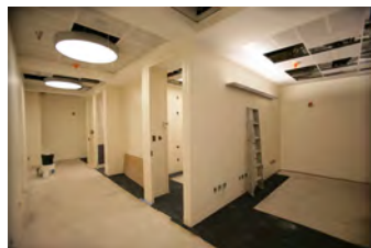
F061207DB-0006 [2018-0227-F_M1Hi_j0044_2.JPG] 6/12/2007 Brady Press Briefing Room Renovations
