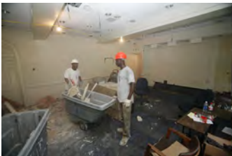
F081506PM-0007 [2018-0227-F_M1Hi_j0146_2.JPG] 8/15/2006 Press Briefing Room Renovations
