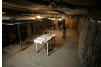
F101906PM-021 [2018-0227-F_M1Hi_j0010_1.JPG] 10/19/2006 Renovations to the Press Briefing room
