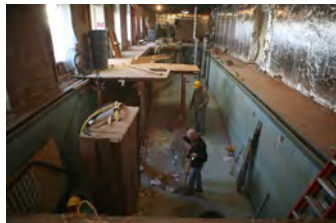
F120206PM-0021 [2018-0227-F_M1Hi_j0184_4.JPG] 12/2/2006 Press Briefing room renovations.
