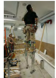
F061507CG-0032 [2018-0227-F_M2Hi_j0219.JPG] 6/15/2007 The Press Briefing Room nears completion
