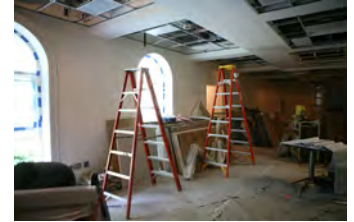
F053107LS-0003 [2018-0227-F_M1Hi_j0062_3.JPG] 5/31/2007 renovation progress of James S. Brady Press Briefing Room
