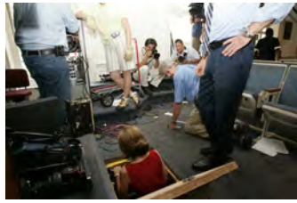
F080306PM-0041 [2018-0227-F_M1Hi_j0159.JPG] 8/3/2006 Clearing out Press Briefing room for renovations.
