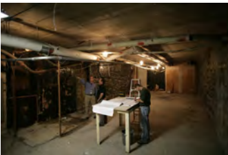
F101906PM-027 [2018-0227-F_M1Hi_j0022_1.JPG] 10/19/2006 Renovations to the Press Briefing room
