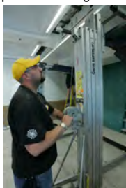
F062007CG-0026 [2018-0227-F_M2Hi_j0222.JPG] 6/20/2007 Work continues on the press briefing room
