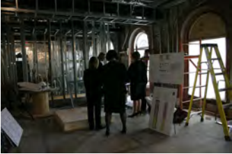
P040207SC-0002 [2018-0227-F_M1Hi_j0180_5.JPG] 4/2/2007 LB. The Brady Press Room During Renovations.
