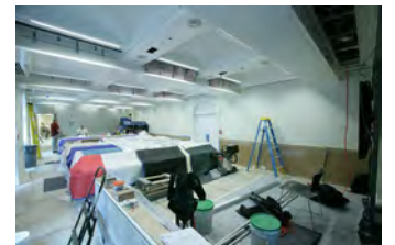
F062707CG-0052 [2018-0227-F_M1Hi_j0065_3.JPG] 6/27/2007 Work continues on the press briefing room
