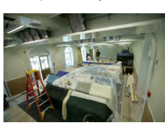
F062707CG-0006 [2018-0227-F_M1Hi_j0117_3.JPG] 6/27/2007 Work continues on the press briefing room
