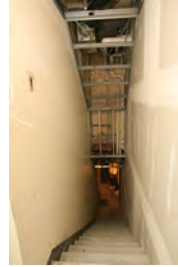
F051607SC-0116 [2018-0227-F_M1Hi_j0062_2.JPG] 5/16/2007 Press Briefing Room Renovations
