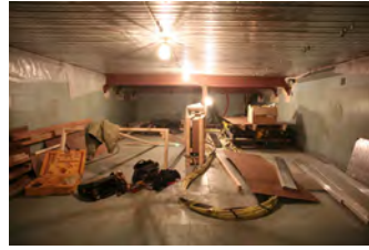
F012507PM-0016 [2018-0227-F_M1Hi_j0045.JPG] 1/25/2007 Press Briefing room renovations.
