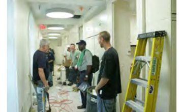
F062807CG-0062 [2018-0227-F_M1Hi_j0201_2.JPG] 6/28/2007 Work continues on the press briefing room
