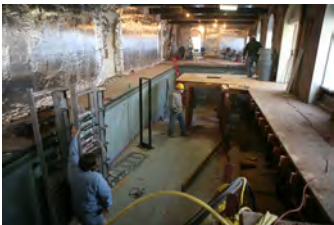
F120206PM-0001 [2018-0227-F_M1Hi_j0144_3.JPG] 12/2/2006 Press Briefing room renovations.
