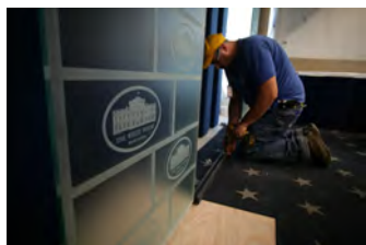
P062107ED-0358 [2018-0227-F_M1Hi_j0088_6.JPG] 6/21/2007 Press Briefing Room Renovations. West Wing.
