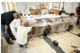
P062107ED-0273 [2018-0227-F_M1Hi_j0173_8.JPG] 6/21/2007 Press Briefing Room Renovations. West Wing.
