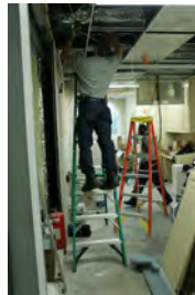
F062707CG-0039 [2018-0227-F_M1Hi_j0013_5.JPG] 6/27/2007 Work continues on the press briefing room
