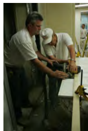
F062907CG-0046 [2018-0227-F_M1Hi_j0183_5.JPG] 6/29/2007 Work nears completion on the press briefing room, Friday June 29, 2007.
