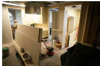
P062107ED-0222 [2018-0227-F_M1Hi_j0071_3.JPG] 6/21/2007 Press Briefing Room Renovations. West Wing.
