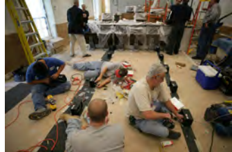
P062107ED-0294 [2018-0227-F_M1Hi_j0215_5.JPG] 6/21/2007 Press Briefing Room Renovations. West Wing.
