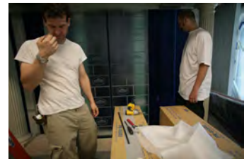
P062107ED-0264 [2018-0227-F_M1Hi_j0155_7.JPG] 6/21/2007 Press Briefing Room Renovations. West Wing.
