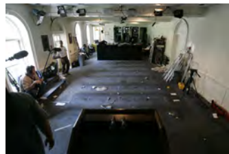
F080306PM-0190 [2018-0227-F_M1Hi_j0202.JPG] 8/3/2006 Clearing out Press Briefing room for renovations.
