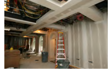
F051607SC-0097 [2018-0227-F_M1Hi_j0024_3.JPG] 5/16/2007 Press Briefing Room Renovations
