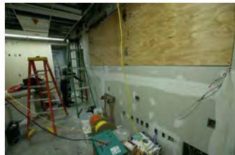
F062707CG-0047 [2018-0227-F_M1Hi_j0045_3.JPG] 6/27/2007 Work continues on the press briefing room
