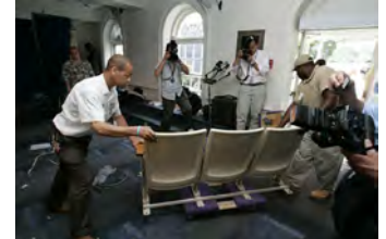
F080306PM-0147 [2018-0227-F_M1Hi_j0116.JPG] 8/3/2006 Clearing out Press Briefing room for renovations.
