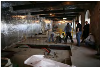
F010907PM-0011 [2018-0227-F_M1Hi_j0136_2.JPG] 1/9/2007 Press Briefing Room Renovations
