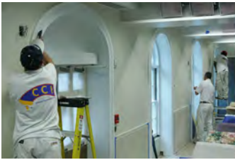
F062807CG-0055 [2018-0227-F_M1Hi_j0187_4.JPG] 6/28/2007 Work continues on the press briefing room
