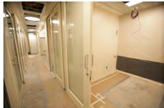
F061207DB-0049 [2018-0227-F_M1Hi_j0070_4.JPG] 6/12/2007 Brady Press Briefing Room Renovations
