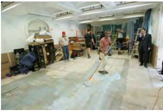
F062007CG-0098 [2018-0227-F_M2Hi_j0111.JPG] 6/20/2007 Work continues on the press briefing room
