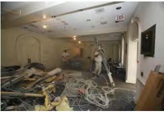
F081506PM-0016 [2018-0227-F_M1Hi_j0164_2.JPG] 8/15/2006 Press Briefing Room Renovations
