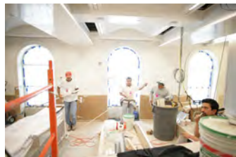
P062107ED-0246 [2018-0227-F_M1Hi_j0119_7.JPG] 6/21/2007 Press Briefing Room Renovations. West Wing.
