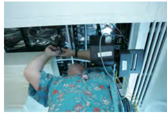
F062907CG-0051 [2018-0227-F_M1Hi_j0193_5.JPG] 6/29/2007 Work nears completion on the press briefing room, Friday June 29, 2007.
