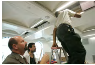
F061507CG-0066 [2018-0227-F_M2Hi_j0032.JPG] 6/15/2007 The Press Briefing Room nears completion
