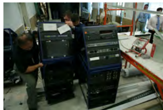
F062207CG-0055 [2018-0227-F_M1Hi_j0150_10.JPG] 6/22/2007 Work continues on the press briefing room
