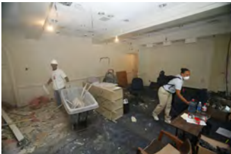
F081506PM-0003 [2018-0227-F_M1Hi_j0138_2.JPG] 8/15/2006 Press Briefing Room Renovations
