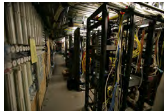
F061207DB-0038 [2018-0227-F_M1Hi_j0004_3.JPG] 6/12/2007 Brady Press Briefing Room Renovations
