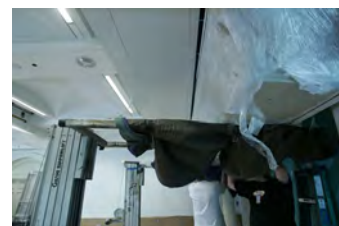
F062007CG-0025 [2018-0227-F_M2Hi_j0220.JPG] 6/20/2007 Work continues on the press briefing room
