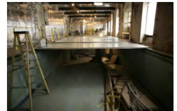
F121506PM-0005 [2018-0227-F_M1Hi_j0113_1.JPG] 12/15/2006 Press Briefing room renovations
