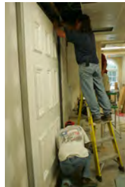
F062807CG-0025 [2018-0227-F_M1Hi_j0127_2.JPG] 6/28/2007 Work continues on the press briefing room
