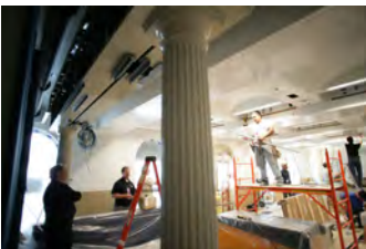
P062107ED-0225 [2018-0227-F_M1Hi_j0077_3.JPG] 6/21/2007 Press Briefing Room Renovations. West Wing.
