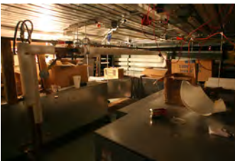
F051607SC-0026 [2018-0227-F_M1Hi_j0120_3.JPG] 5/16/2007 Press Briefing Room Renovations
