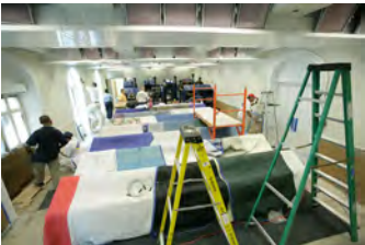
F062807CG-0023 [2018-0227-F_M1Hi_j0123_3.JPG] 6/28/2007 Work continues on the press briefing room
