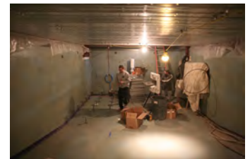
F012507PM-0013 [2018-0227-F_M1Hi_j0039.JPG] 1/25/2007 Press Briefing room renovations.
