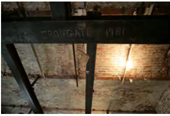
F101906PM-035 [2018-0227-F_M1Hi_j0038_1.JPG] 10/19/2006 Renovations to the Press Briefing room
