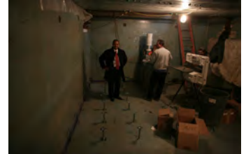
F012507PM-0021 [2018-0227-F_M1Hi_j0055.JPG] 1/25/2007 Press Briefing room renovations.
