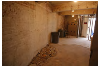
F110106PM-0005 [2018-0227-F_M1Hi_j0023.JPG] 11/1/2006 Press Briefing room renovations
