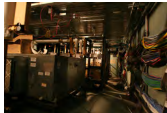
F051607SC-0024 [2018-0227-F_M1Hi_j0112_1.JPG] 5/16/2007 Press Briefing Room Renovations
