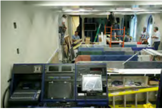
F062907CG-0029 [2018-0227-F_M1Hi_j0028_4.JPG] 6/29/2007 Work nears completion on the press briefing room, Friday June 29, 2007.
