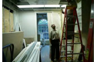
F062007CG-0004 [2018-0227-F_M2Hi_j0178.JPG] 6/20/2007 Work continues on the press briefing room
