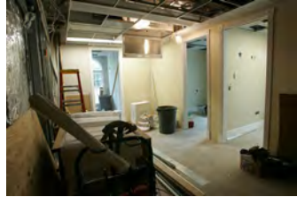
F061507CG-0030 [2018-0227-F_M2Hi_j0215.JPG] 6/15/2007 The Press Briefing Room nears completion
