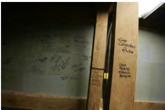
F080306PM-0092 [2018-0227-F_M1Hi_j0006.JPG] 8/3/2006 Clearing out Press Briefing room for renovations.
