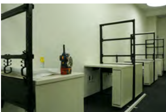
F062907CG-0005 [2018-0227-F_M1Hi_j0235_4.JPG] 6/29/2007 Work nears completion on the press briefing room, Friday June 29, 2007.
