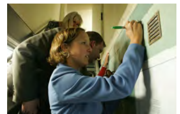
F070207CG-0007 [2018-0227-F_M1Hi_j0045_4.JPG] 7/2/2007 Work nears completion on the press briefing room
