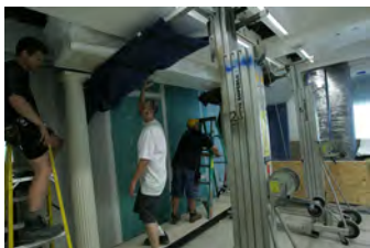
F062007CG-0030 [2018-0227-F_M2Hi_j0230.JPG] 6/20/2007 Work continues on the press briefing room
