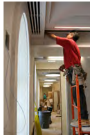
P061907DG-0241 [2018-0227-F_M1Hi_j0241_3.JPG] 6/19/2007 James S. Brady Press Briefing Room renovation
