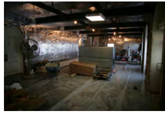
F010907PM-0005 [2018-0227-F_M1Hi_j0124_1.JPG] 1/9/2007 Press Briefing Room Renovations
