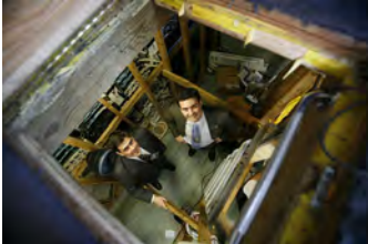
F080406PM-0053 [2018-0227-F_M1Hi_j0242.JPG] 8/4/2006 Clearing out Press Briefing room for renovations.
