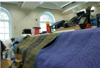
F062807CG-0031 [2018-0227-F_M1Hi_j0139_2.JPG] 6/28/2007 Work continues on the press briefing room
