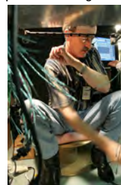
F062807CG-0042 [2018-0227-F_M1Hi_j0161_2.JPG] 6/28/2007 Work continues on the press briefing room
