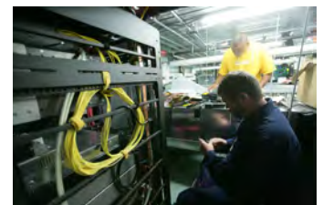
F062007CG-0017 [2018-0227-F_M2Hi_j0204.JPG] 6/20/2007 Work continues on the press briefing room
