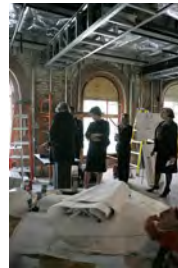
P040207SC-0024 [2018-0227-F_M1Hi_j0036_2.JPG] 4/2/2007 LB. The Brady Press Room During Renovations.
