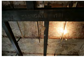
F101906PM-036 [2018-0227-F_M1Hi_j0040_1.JPG] 10/19/2006 Renovations to the Press Briefing room
