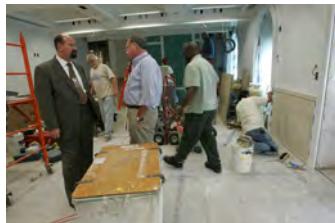
F061507CG-0058 [2018-0227-F_M2Hi_j0016.JPG] 6/15/2007 The Press Briefing Room nears completion
