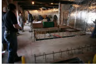
F010907PM-0008 [2018-0227-F_M1Hi_j0130_1.JPG] 1/9/2007 Press Briefing Room Renovations
