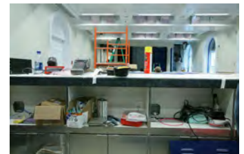
F062807CG-0066 [2018-0227-F_M1Hi_j0209_5.JPG] 6/28/2007 Work continues on the press briefing room
