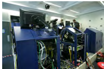
F070207CG-0029 [2018-0227-F_M1Hi_j0091_2.JPG] 7/2/2007 Work nears completion on the press briefing room
