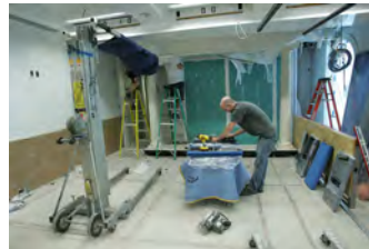
F062007CG-0048 [2018-0227-F_M2Hi_j0011.JPG] 6/20/2007 Work continues on the press briefing room
