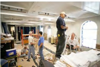
P062107ED-0245 [2018-0227-F_M1Hi_j0117_7.JPG] 6/21/2007 Press Briefing Room Renovations. West Wing.
