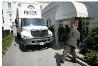
P062107ED-0327 [2018-0227-F_M1Hi_j0026_6.JPG] 6/21/2007 Press Briefing Room Renovations. West Wing.
