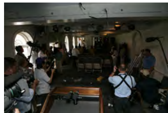
F080306PM-0158 [2018-0227-F_M1Hi_j0138.JPG] 8/3/2006 Clearing out Press Briefing room for renovations.
