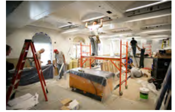
P062107ED-0232 [2018-0227-F_M1Hi_j0091_4.JPG] 6/21/2007 Press Briefing Room Renovations. West Wing.
