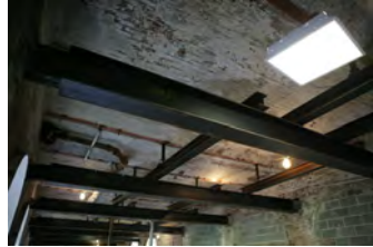
F101806KH-0016 [2018-0227-F_M1Hi_j0176_3.JPG] 10/18/2006 Press Room Renovations
