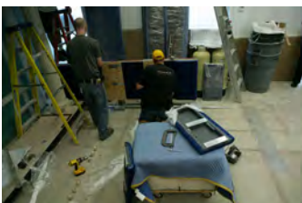
F062007CG-0094 [2018-0227-F_M2Hi_j0103.JPG] 6/20/2007 Work continues on the press briefing room
