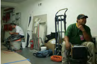
F062907CG-0013 [2018-0227-F_M1Hi_j0251_5.JPG] 6/29/2007 Work nears completion on the press briefing room, Friday June 29, 2007.
