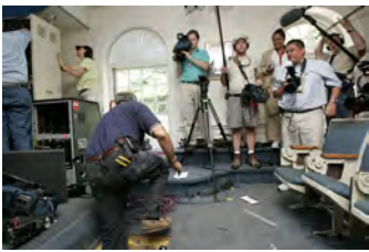
F080306PM-0021 [2018-0227-F_M1Hi_j0119.JPG] 8/3/2006 Clearing out Press Briefing room for renovations.
