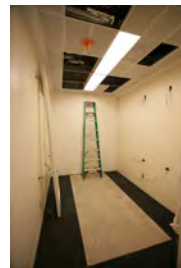
F061207DB-0007 [2018-0227-F_M1Hi_j0050_3.JPG] 6/12/2007 Brady Press Briefing Room Renovations
