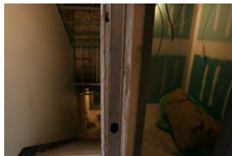
F051607SC-0107 [2018-0227-F_M1Hi_j0044_1.JPG] 5/16/2007 Press Briefing Room Renovations
