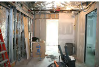
F053107LS-0012 [2018-0227-F_M1Hi_j0080_2.JPG] 5/31/2007 renovation progress of James S. Brady Press Briefing Room
