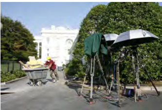
F081506PM-0048 [2018-0227-F_M1Hi_j0228_1.JPG] 8/15/2006 Press Briefing Room Renovations
