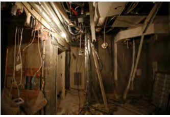
F081506PM-0036 [2018-0227-F_M1Hi_j0204_2.JPG] 8/15/2006 Press Briefing Room Renovations
