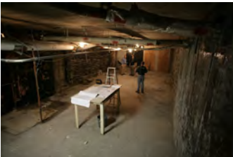
F101906PM-023 [2018-0227-F_M1Hi_j0014_1.JPG] 10/19/2006 Renovations to the Press Briefing room
