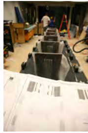
F062107DG-0014 [2018-0227-F_M1Hi_j0114_4.JPG] 6/21/2007 White House Press Briefing Room renovations Thursday, June 21, 2007. White House photo by Debra Gulbas
