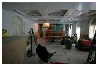
F061207DB-0014 [2018-0227-F_M1Hi_j0101_2.JPG] 6/12/2007 Brady Press Briefing Room Renovations
