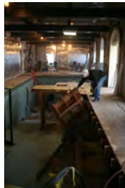
F120206PM-0014 [2018-0227-F_M1Hi_j0170_4.JPG] 12/2/2006 Press Briefing room renovations.
