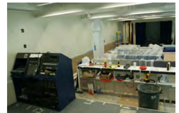
F062707CG-0012 [2018-0227-F_M1Hi_j0147_3.JPG] 6/27/2007 Work continues on the press briefing room
