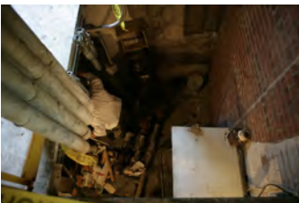
F101806KH-0027 [2018-0227-F_M1Hi_j0198_3.JPG] 10/18/2006 Press Room Renovations
