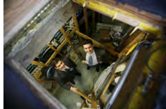
F080406PM-0054 [2018-0227-F_M1Hi_j0244.JPG] 8/4/2006 Clearing out Press Briefing room for renovations.
