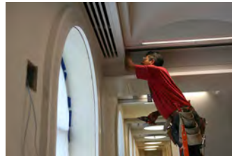
P061907DG-0238 [2018-0227-F_M1Hi_j0235_2.JPG] 6/19/2007 James S. Brady Press Briefing Room renovation
