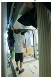
F062007CG-0034 [2018-0227-F_M2Hi_j0238.JPG] 6/20/2007 Work continues on the press briefing room
