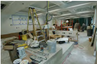
F061507CG-0053 [2018-0227-F_M2Hi_j0006.JPG] 6/15/2007 The Press Briefing Room nears completion
