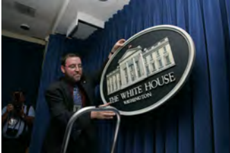
F080306PM-0064 [2018-0227-F_M1Hi_j0205.JPG] 8/3/2006 Clearing out Press Briefing room for renovations.
