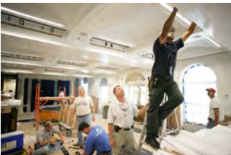
P062107ED-0241 [2018-0227-F_M1Hi_j0109_8.JPG] 6/21/2007 Press Briefing Room Renovations. West Wing.
