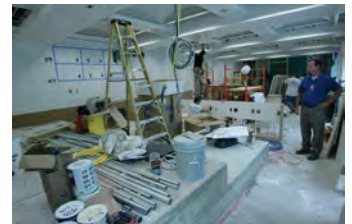
F061507CG-0052 [2018-0227-F_M2Hi_j0004.JPG] 6/15/2007 The Press Briefing Room nears completion
