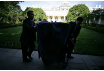
P062207ED-0018 [2018-0227-F_M1Hi_j0049_2.JPG] 6/22/2007 Press Briefing Room rennovations
