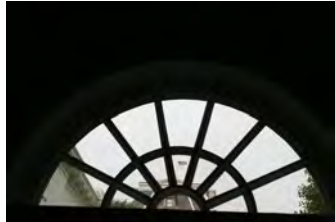
F051607SC-0059 [2018-0227-F_M1Hi_j0203_2.JPG] 5/16/2007 Press Briefing Room Renovations
