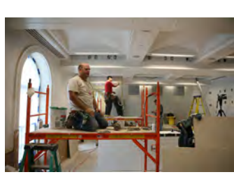
P061907DG-0221 [2018-0227-F_M1Hi_j0200_6.JPG] 6/19/2007 James S. Brady Press Briefing Room renovation
