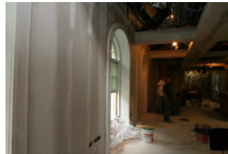
F051607SC-0100 [2018-0227-F_M1Hi_j0030_3.JPG] 5/16/2007 Press Briefing Room Renovations
