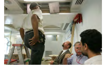
F061507CG-0072 [2018-0227-F_M2Hi_j0044.JPG] 6/15/2007 The Press Briefing Room nears completion
