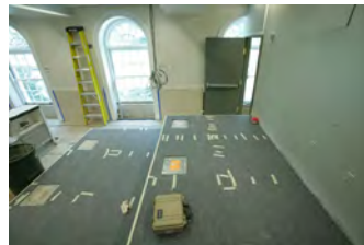
F062707CG-0019 [2018-0227-F_M1Hi_j0175_3.JPG] 6/27/2007 Work continues on the press briefing room
