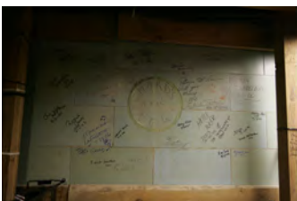
F080306PM-0076 [2018-0227-F_M1Hi_j0229.JPG] 8/3/2006 Clearing out Press Briefing room for renovations.
