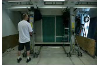
F062007CG-0040 [2018-0227-F_M2Hi_j0250.JPG] 6/20/2007 Work continues on the press briefing room
