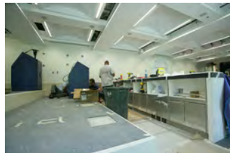
F062707CG-0026 [2018-0227-F_M1Hi_j0203_4.JPG] 6/27/2007 Work continues on the press briefing room
