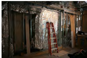
F053107LS-0009 [2018-0227-F_M1Hi_j0074_2.JPG] 5/31/2007 renovation progress of James S. Brady Press Briefing Room
