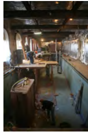
F120206PM-0031 [2018-0227-F_M1Hi_j0204_4.JPG] 12/2/2006 Press Briefing room renovations.
