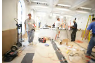
P062107ED-0235 [2018-0227-F_M1Hi_j0097_5.JPG] 6/21/2007 Press Briefing Room Renovations. West Wing.
