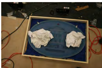
F062107DG-0026 [2018-0227-F_M1Hi_j0126_4.JPG] 6/21/2007 White House Press Briefing Room renovations Thursday, June 21, 2007. White House photo by Debra Gulbas
