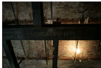
F101906PM-032 [2018-0227-F_M1Hi_j0032_1.JPG] 10/19/2006 Renovations to the Press Briefing room
