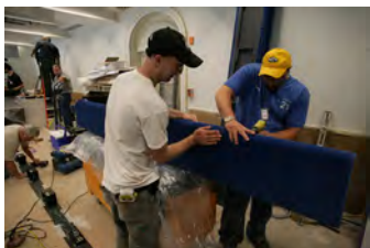
P062107ED-0281 [2018-0227-F_M1Hi_j0189_7.JPG] 6/21/2007 Press Briefing Room Renovations. West Wing.
