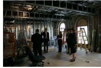
P040207SC-0040 [2018-0227-F_M1Hi_j0132_2.JPG] 4/2/2007 LB. The Brady Press Room During Renovations.
