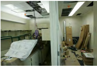
F062007CG-0058 [2018-0227-F_M2Hi_j0031.JPG] 6/20/2007 Work continues on the press briefing room
