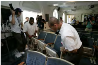
F080306PM-0108 [2018-0227-F_M1Hi_j0038.JPG] 8/3/2006 Clearing out Press Briefing room for renovations.
