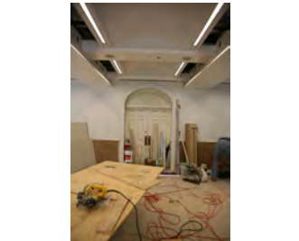
P061907DG-0220 [2018-0227-F_M1Hi_j0199_3.JPG] 6/19/2007 James S. Brady Press Briefing Room renovation
