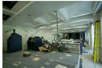
F062707CG-0023 [2018-0227-F_M1Hi_j0191_3.JPG] 6/27/2007 Work continues on the press briefing room
