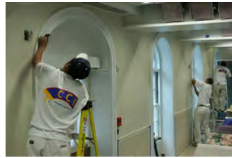
F062807CG-0057 [2018-0227-F_M1Hi_j0191_4.JPG] 6/28/2007 Work continues on the press briefing room
