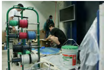
F062907CG-0038 [2018-0227-F_M1Hi_j0046_4.JPG] 6/29/2007 Work nears completion on the press briefing room, Friday June 29, 2007.
