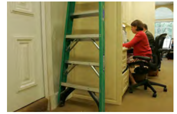
F070207CG-0011 [2018-0227-F_M1Hi_j0087_1.JPG] 7/2/2007 Work nears completion on the press briefing room
