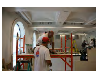
P061907DG-0222 [2018-0227-F_M1Hi_j0203_3.JPG] 6/19/2007 James S. Brady Press Briefing Room renovation
