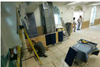
F062007CG-0074 [2018-0227-F_M2Hi_j0063.JPG] 6/20/2007 Work continues on the press briefing room
