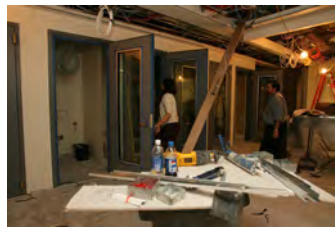
F051607SC-0127 [2018-0227-F_M1Hi_j0084_2.JPG] 5/16/2007 Press Briefing Room Renovations
