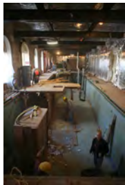
F120206PM-0025 [2018-0227-F_M1Hi_j0192_4.JPG] 12/2/2006 Press Briefing room renovations.
