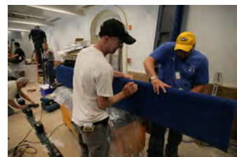
P062107ED-0280 [2018-0227-F_M1Hi_j0187_8.JPG] 6/21/2007 Press Briefing Room Renovations. West Wing.
