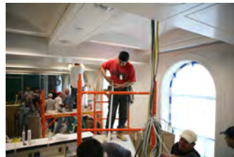
P061907DG-0202 [2018-0227-F_M1Hi_j0163_2.JPG] 6/19/2007 James S. Brady Press Briefing Room renovation
