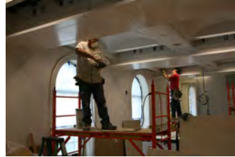
P061907DG-0234 [2018-0227-F_M1Hi_j0227_2.JPG] 6/19/2007 James S. Brady Press Briefing Room renovation
