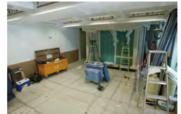
F062007CG-0069 [2018-0227-F_M2Hi_j0053.JPG] 6/20/2007 Work continues on the press briefing room
