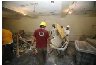
F081506PM-0046 [2018-0227-F_M1Hi_j0224_1.JPG] 8/15/2006 Press Briefing Room Renovations
