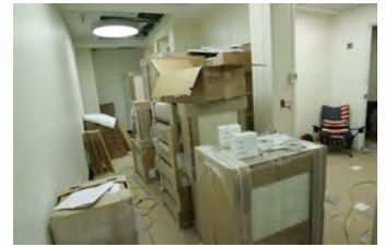
F061507CG-0048 [2018-0227-F_M2Hi_j0251.JPG] 6/15/2007 The Press Briefing Room nears completion
