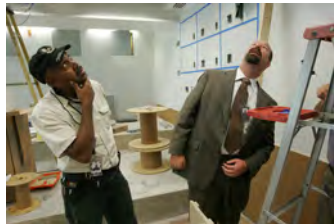
F061507CG-0074 [2018-0227-F_M2Hi_j0048.JPG] 6/15/2007 The Press Briefing Room nears completion
