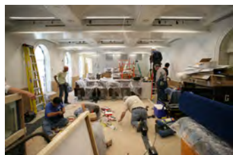
P062107ED-0279 [2018-0227-F_M1Hi_j0185_7.JPG] 6/21/2007 Press Briefing Room Renovations. West Wing.
