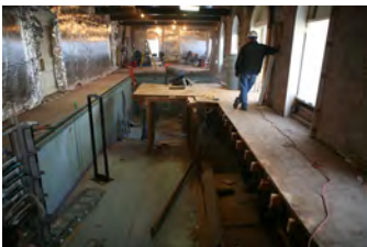
F120206PM-0005 [2018-0227-F_M1Hi_j0152_4.JPG] 12/2/2006 Press Briefing room renovations.
