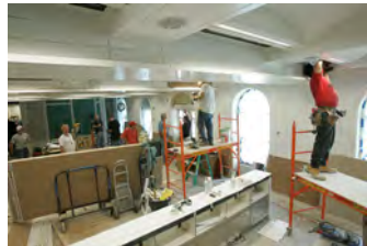
F061907CG-0002 [2018-0227-F_M2Hi_j0181_1.JPG] 6/19/2007 Work continues on the Brady Briefing Room
