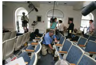
F080306PM-0054 [2018-0227-F_M1Hi_j0185.JPG] 8/3/2006 Clearing out Press Briefing room for renovations.
