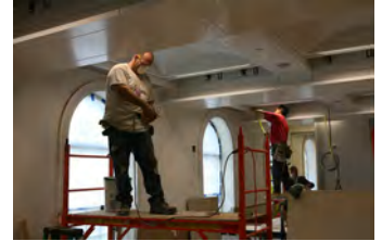
P061907DG-0235 [2018-0227-F_M1Hi_j0229_3.JPG] 6/19/2007 James S. Brady Press Briefing Room renovation
