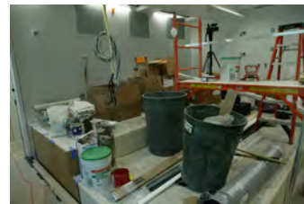
F062207CG-0032 [2018-0227-F_M1Hi_j0104_4.JPG] 6/22/2007 Work continues on the press briefing room
