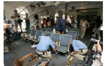
F080306PM-0016 [2018-0227-F_M1Hi_j0109.JPG] 8/3/2006 Clearing out Press Briefing room for renovations.
