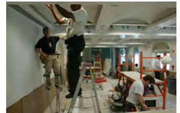
F061507CG-0056 [2018-0227-F_M2Hi_j0012.JPG] 6/15/2007 The Press Briefing Room nears completion
