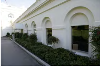
F101806KH-0035 [2018-0227-F_M1Hi_j0214_2.JPG] 10/18/2006 Press Room Renovations
