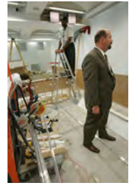
F061507CG-0068 [2018-0227-F_M2Hi_j0036.JPG] 6/15/2007 The Press Briefing Room nears completion
