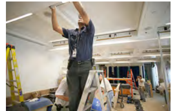
P062107ED-0240 [2018-0227-F_M1Hi_j0107_7.JPG] 6/21/2007 Press Briefing Room Renovations. West Wing.
