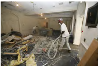
F081506PM-0011 [2018-0227-F_M1Hi_j0154_2.JPG] 8/15/2006 Press Briefing Room Renovations
