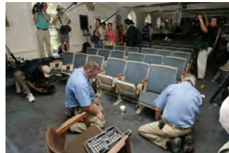
F080306PM-0011 [2018-0227-F_M1Hi_j0099.JPG] 8/3/2006 Clearing out Press Briefing room for renovations.
