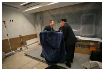
P062207ED-0041 [2018-0227-F_M1Hi_j0153_3.JPG] 6/22/2007 Press Briefing Room rennovations
