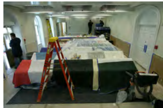
F062707CG-0002 [2018-0227-F_M1Hi_j0101_4.JPG] 6/27/2007 Work continues on the press briefing room
