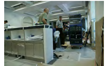
F062207CG-0044 [2018-0227-F_M1Hi_j0128_5.JPG] 6/22/2007 Work continues on the press briefing room
