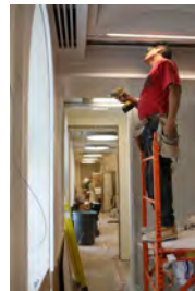
P061907DG-0246 [2018-0227-F_M1Hi_j0251_3.JPG] 6/19/2007 James S. Brady Press Briefing Room renovation
