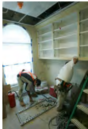
F061907CG-0005 [2018-0227-F_M2Hi_j0187_1.JPG] 6/19/2007 Work continues on the Brady Briefing Room
