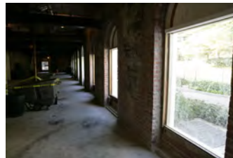
F101806KH-0025 [2018-0227-F_M1Hi_j0194_3.JPG] 10/18/2006 Press Room Renovations
