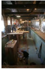
F120206PM-0030 [2018-0227-F_M1Hi_j0202_4.JPG] 12/2/2006 Press Briefing room renovations.
