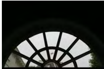
F051607SC-0063 [2018-0227-F_M1Hi_j0211_2.JPG] 5/16/2007 Press Briefing Room Renovations
