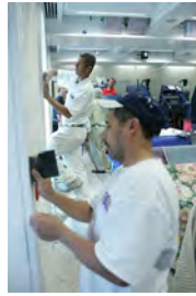
F062807CG-0017 [2018-0227-F_M1Hi_j0111_3.JPG] 6/28/2007 Work continues on the press briefing room
