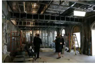
P040207SC-0039 [2018-0227-F_M1Hi_j0126_2.JPG] 4/2/2007 LB. The Brady Press Room During Renovations.
