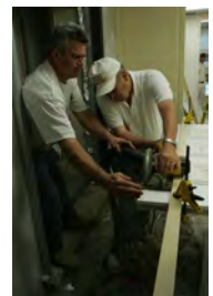
F062907CG-0048 [2018-0227-F_M1Hi_j0187_5.JPG] 6/29/2007 Work nears completion on the press briefing room, Friday June 29, 2007.
