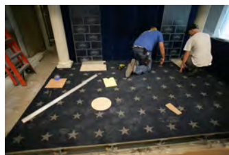
P062107ED-0351 [2018-0227-F_M1Hi_j0074_4.JPG] 6/21/2007 Press Briefing Room Renovations. West Wing.
