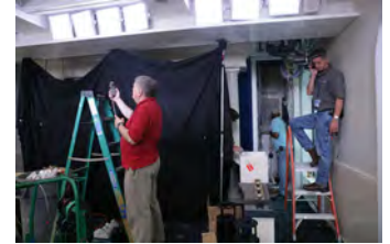
F070507CG-0055 [2018-0227-F_M1Hi_J0211_6.JPG] 7/5/2007 Work nears completion on the press briefing room and the Lower Press office.
