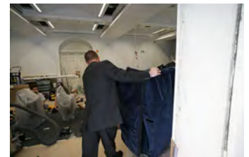
P062207ED-0035 [2018-0227-F_M1Hi_j0162_6.JPG] 6/22/2007 Press Briefing Room rennovations
