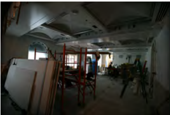
F061207DB-0028 [2018-0227-F_M1Hi_j0192_6.JPG] 6/12/2007 Brady Press Briefing Room Renovations
