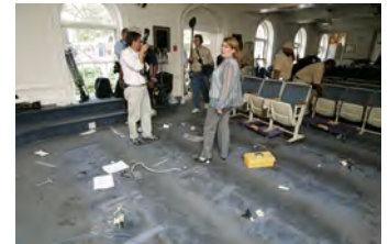
F080306PM-0151 [2018-0227-F_M1Hi_j0124.JPG] 8/3/2006 Clearing out Press Briefing room for renovations.
