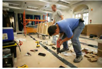
P062107ED-0251 [2018-0227-F_M1Hi_j0129_5.JPG] 6/21/2007 Press Briefing Room Renovations. West Wing.
