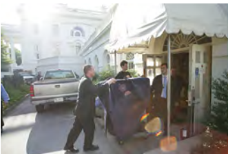
P062207ED-0032 [2018-0227-F_M1Hi_j0023_4.JPG] 6/22/2007 Press Briefing Room rennovations
