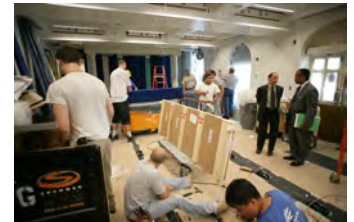
P062107ED-0200 [2018-0227-F_M1Hi_j0027_2.JPG] 6/21/2007 Press Briefing Room Renovations. West Wing.
