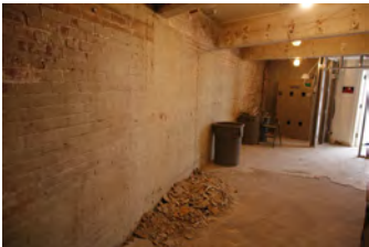
F110106PM-0004 [2018-0227-F_M1Hi_j0021.JPG] 11/1/2006 Press Briefing room renovations
