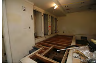
F081506PM-0021 [2018-0227-F_M1Hi_j0174_2.JPG] 8/15/2006 Press Briefing Room Renovations
