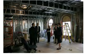
P040207SC-0041 [2018-0227-F_M1Hi_j0138_4.JPG] 4/2/2007 LB. The Brady Press Room During Renovations.
