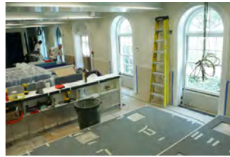
F062707CG-0015 [2018-0227-F_M1Hi_j0159_2.JPG] 6/27/2007 Work continues on the press briefing room
