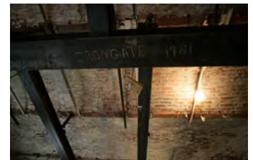
F101906PM-034 [2018-0227-F_M1Hi_j0036_1.JPG] 10/19/2006 Renovations to the Press Briefing room
