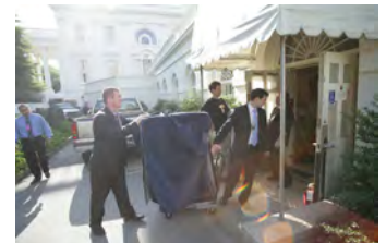
P062207ED-0031 [2018-0227-F_M1Hi_j0010_5.JPG] 6/22/2007 Press Briefing Room rennovations
