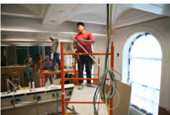
P061907DG-0204 [2018-0227-F_M1Hi_j0167_2.JPG] 6/19/2007 James S. Brady Press Briefing Room renovation
