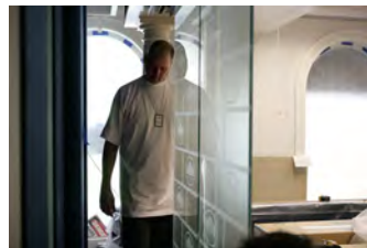
P062107ED-0267 [2018-0227-F_M1Hi_j0161_5.JPG] 6/21/2007 Press Briefing Room Renovations. West Wing.
