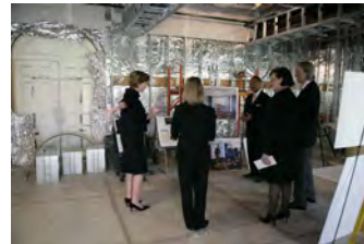
P040207SC-0048 [2018-0227-F_M1Hi_j0208_4.JPG] 4/2/2007 LB. The Brady Press Room During Renovations.
