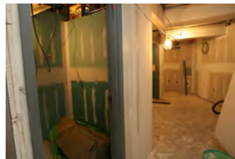
F051607SC-0108 [2018-0227-F_M1Hi_j0046_2.JPG] 5/16/2007 Press Briefing Room Renovations
