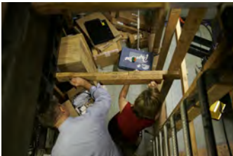
F080306PM-0048 [2018-0227-F_M1Hi_j0173.JPG] 8/3/2006 Clearing out Press Briefing room for renovations.
