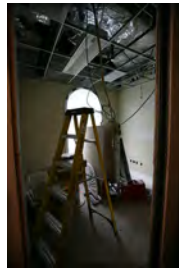
F061207DB-0025 [2018-0227-F_M1Hi_j0174_5.JPG] 6/12/2007 Brady Press Briefing Room Renovations
