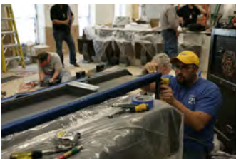
P062107ED-0305 [2018-0227-F_M1Hi_j0237_4.JPG] 6/21/2007 Press Briefing Room Renovations. West Wing.
