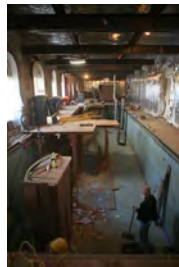
F120206PM-0027 [2018-0227-F_M1Hi_j0196_4.JPG] 12/2/2006 Press Briefing room renovations.
