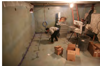
F012507PM-0007 [2018-0227-F_M1Hi_j0027.JPG] 1/25/2007 Press Briefing room renovations.
