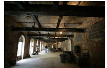
F101906PM-010 [2018-0227-F_M1Hi_j0238_2.JPG] 10/19/2006 Renovations to the Press Briefing room
