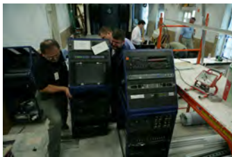
F062207CG-0053 [2018-0227-F_M1Hi_j0146_9.JPG] 6/22/2007 Work continues on the press briefing room
