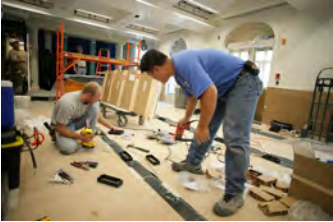
P062107ED-0253 [2018-0227-F_M1Hi_j0133_7.JPG] 6/21/2007 Press Briefing Room Renovations. West Wing.
