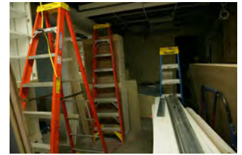
F062007CG-0001 [2018-0227-F_M2Hi_j0172.JPG] 6/20/2007 Work continues on the press briefing room
