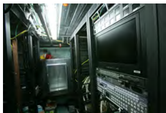
F062007CG-0019 [2018-0227-F_M2Hi_j0208.JPG] 6/20/2007 Work continues on the press briefing room
