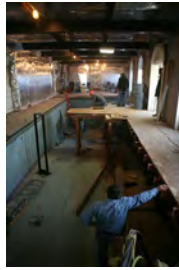
F120206PM-0010 [2018-0227-F_M1Hi_j0162_3.JPG] 12/2/2006 Press Briefing room renovations.
