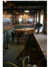
F120206PM-0016 [2018-0227-F_M1Hi_j0174_4.JPG] 12/2/2006 Press Briefing room renovations.
