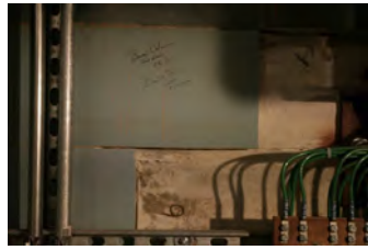
F051607SC-0011 [2018-0227-F_M1Hi_j0046_1.JPG] 5/16/2007 Press Briefing Room Renovations
