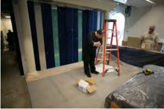
P062107ED-0233 [2018-0227-F_M1Hi_j0093_3.JPG] 6/21/2007 Press Briefing Room Renovations. West Wing.
