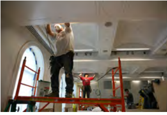
P061907DG-0228 [2018-0227-F_M1Hi_j0215_2.JPG] 6/19/2007 James S. Brady Press Briefing Room renovation
