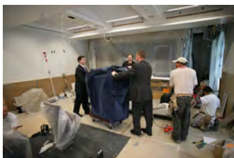
P062207ED-0036 [2018-0227-F_M1Hi_j0195_4.JPG] 6/22/2007 Press Briefing Room rennovations
