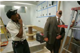
F061507CG-0077 [2018-0227-F_M2Hi_j0054.JPG] 6/15/2007 The Press Briefing Room nears completion
