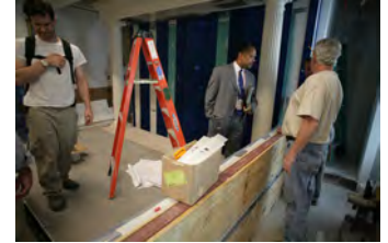
P062107ED-0216 [2018-0227-F_M1Hi_j0059_2.JPG] 6/21/2007 Press Briefing Room Renovations. West Wing.
