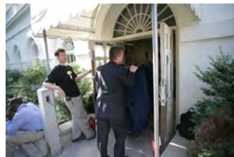
P062207ED-0034 [2018-0227-F_M1Hi_j0182_6.JPG] 6/22/2007 Press Briefing Room rennovations
