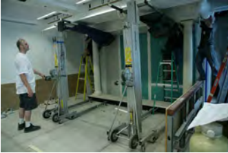
F062007CG-0042 [2018-0227-F_M2Hi_j0254.JPG] 6/20/2007 Work continues on the press briefing room
