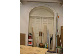
P061907DG-0218 [2018-0227-F_M1Hi_j0195_3.JPG] 6/19/2007 James S. Brady Press Briefing Room renovation
