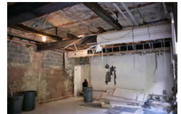
F091806PM-006 [2018-0227-F_M1Hi_j0122_1.JPG] 9/18/2006 Renovations of the Press Briefing Room
