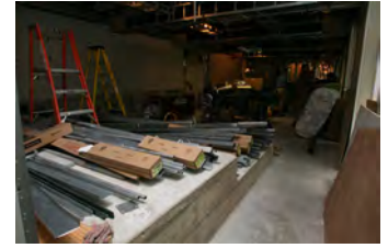
F051607SC-0153 [2018-0227-F_M1Hi_j0136_4.JPG] 5/16/2007 Press Briefing Room Renovations
