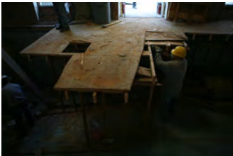
F120206PM-0037 [2018-0227-F_M1Hi_j0216_3.JPG] 12/2/2006 Press Briefing room renovations.
