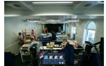
F070207CG-0027 [2018-0227-F_M1Hi_j0087_2.JPG] 7/2/2007 Work nears completion on the press briefing room
