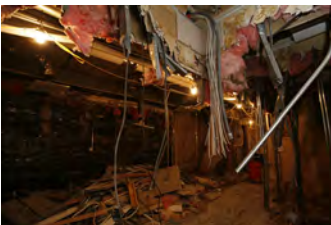
F081506PM-0032 [2018-0227-F_M1Hi_j0196_2.JPG] 8/15/2006 Press Briefing Room Renovations
