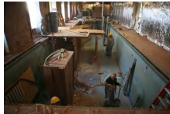
F120206PM-0019 [2018-0227-F_M1Hi_j0180_4.JPG] 12/2/2006 Press Briefing room renovations.
