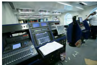
F062807CG-0064 [2018-0227-F_M1Hi_j0205_3.JPG] 6/28/2007 Work continues on the press briefing room
