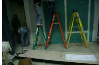
F062007CG-0003 [2018-0227-F_M2Hi_j0176.JPG] 6/20/2007 Work continues on the press briefing room
