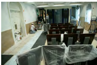
F062207CG-0005 [2018-0227-F_M1Hi_j0050_5.JPG] 6/22/2007 Work continues on the press briefing room
