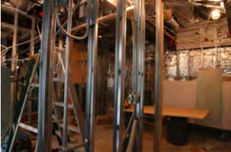
F051607SC-0074 [2018-0227-F_M1Hi_j0233_2.JPG] 5/16/2007 Press Briefing Room Renovations
