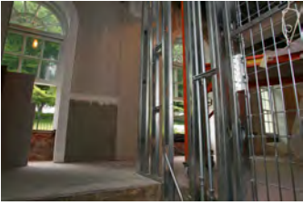
F051607SC-0150 [2018-0227-F_M1Hi_j0130_2.JPG] 5/16/2007 Press Briefing Room Renovations
