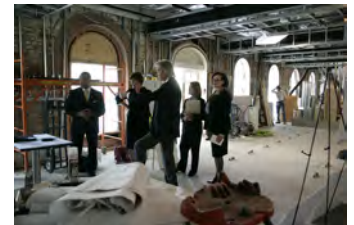
P040207SC-0013 [2018-0227-F_M1Hi_j0229_1.JPG] 4/2/2007 LB. The Brady Press Room During Renovations.
