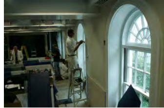
F062807CG-0021 [2018-0227-F_M1Hi_j0119_4.JPG] 6/28/2007 Work continues on the press briefing room
