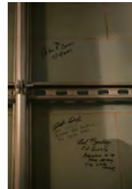
F051607SC-0017 [2018-0227-F_M1Hi_j0070_1.JPG] 5/16/2007 Press Briefing Room Renovations
