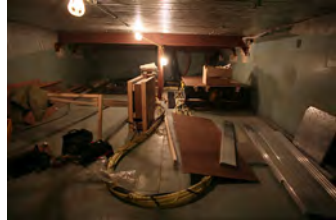
F012507PM-0019 [2018-0227-F_M1Hi_j0051.JPG] 1/25/2007 Press Briefing room renovations.
