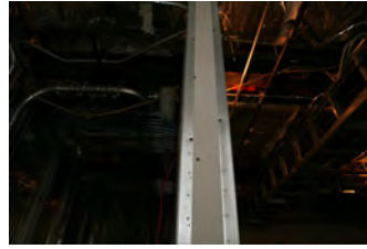
F051607SC-0152 [2018-0227-F_M1Hi_j0134_3.JPG] 5/16/2007 Press Briefing Room Renovations
