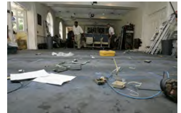
F080306PM-0171 [2018-0227-F_M1Hi_j0164.JPG] 8/3/2006 Clearing out Press Briefing room for renovations.
