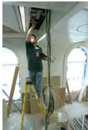
F061507CG-0010 [2018-0227-F_M2Hi_j0175.JPG] 6/15/2007 The Press Briefing Room nears completion
