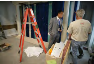
P062107ED-0217 [2018-0227-F_M1Hi_j0061_6.JPG] 6/21/2007 Press Briefing Room Renovations. West Wing.
