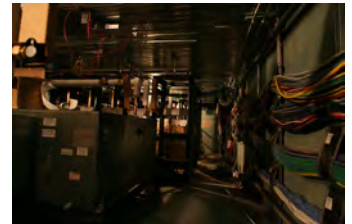
F051607SC-0021 [2018-0227-F_M1Hi_j0094_1.JPG] 5/16/2007 Press Briefing Room Renovations
