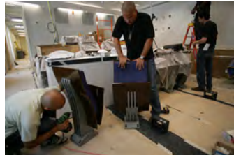
P062107ED-0318 [2018-0227-F_M1Hi_j0008_5.JPG] 6/21/2007 Press Briefing Room Renovations. West Wing.
