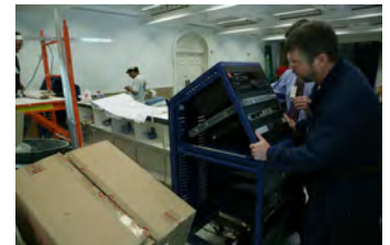
F062207CG-0048 [2018-0227-F_M1Hi_j0136_7.JPG] 6/22/2007 Work continues on the press briefing room
