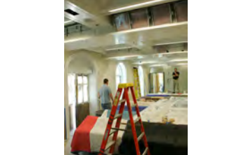
F062707CG-0004 [2018-0227-F_M1Hi_j0109_3.JPG] 6/27/2007 Work continues on the press briefing room
