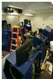
F070507CG-0045 [2018-0227-F_M1Hi_j0191_6.JPG] 7/5/2007 Work nears completion on the press briefing room and the Lower Press office.
