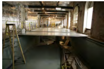
F121506PM-0003 [2018-0227-F_M1Hi_j0109_1.JPG] 12/15/2006 Press Briefing room renovations
