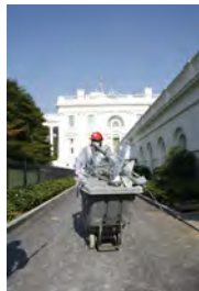
F081506PM-0053 [2018-0227-F_M1Hi_j0238_1.JPG] 8/15/2006 Press Briefing Room Renovations
