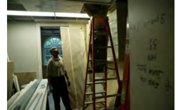
F062007CG-0005 [2018-0227-F_M2Hi_j0180.JPG] 6/20/2007 Work continues on the press briefing room
