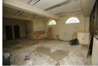
F081506PM-0022 [2018-0227-F_M1Hi_j0176_2.JPG] 8/15/2006 Press Briefing Room Renovations
