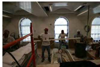
P062107ED-0247 [2018-0227-F_M1Hi_j0121_7.JPG] 6/21/2007 Press Briefing Room Renovations. West Wing.
