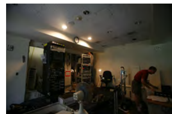
F080406PM-0040 [2018-0227-F_M1Hi_j0216.JPG] 8/4/2006 Clearing out Press Briefing room for renovations.
