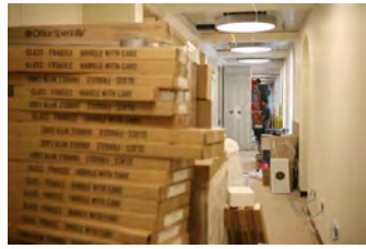
P061907DG-0249 [2018-0227-F_M1Hi_j0002_3.JPG] 6/19/2007 James S. Brady Press Briefing Room renovation
