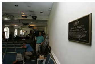
F080306PM-0038 [2018-0227-F_M1Hi_j0153.JPG] 8/3/2006 Clearing out Press Briefing room for renovations.
