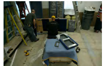
F062007CG-0093 [2018-0227-F_M2Hi_j0101.JPG] 6/20/2007 Work continues on the press briefing room
