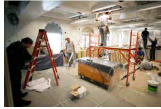
P062107ED-0231 [2018-0227-F_M1Hi_j0089_4.JPG] 6/21/2007 Press Briefing Room Renovations. West Wing.
