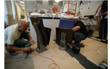
P062107ED-0320 [2018-0227-F_M1Hi_j0012_5.JPG] 6/21/2007 Press Briefing Room Renovations. West Wing.
