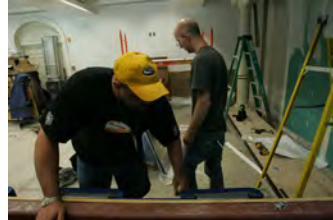
F062007CG-0084 [2018-0227-F_M2Hi_j0083.JPG] 6/20/2007 Work continues on the press briefing room
