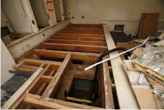
F081506PM-0020 [2018-0227-F_M1Hi_j0172_2.JPG] 8/15/2006 Press Briefing Room Renovations
