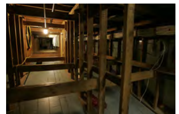
F080306PM-0079 [2018-0227-F_M1Hi_j0235.JPG] 8/3/2006 Clearing out Press Briefing room for renovations.
