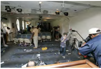
F080306PM-0160 [2018-0227-F_M1Hi_j0142.JPG] 8/3/2006 Clearing out Press Briefing room for renovations.
