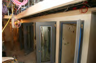
F051607SC-0135 [2018-0227-F_M1Hi_j0100_2.JPG] 5/16/2007 Press Briefing Room Renovations
