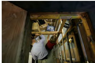
F080306PM-0049 [2018-0227-F_M1Hi_j0175.JPG] 8/3/2006 Clearing out Press Briefing room for renovations.
