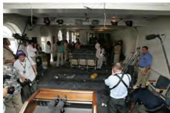
F080306PM-0157 [2018-0227-F_M1Hi_j0136.JPG] 8/3/2006 Clearing out Press Briefing room for renovations.
