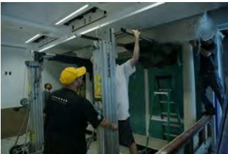
F062007CG-0046 [2018-0227-F_M2Hi_j0007.JPG] 6/20/2007 Work continues on the press briefing room
