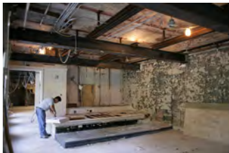
F091806PM-003 [2018-0227-F_M1Hi_j0110_1.JPG] 9/18/2006 Renovations of the Press Briefing Room
