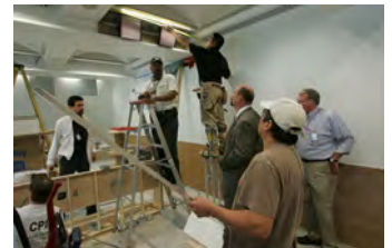
F061507CG-0060 [2018-0227-F_M2Hi_j0020.JPG] 6/15/2007 The Press Briefing Room nears completion
