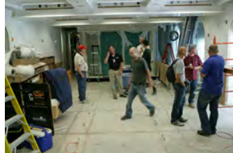
F062007CG-0063 [2018-0227-F_M2Hi_j0041.JPG] 6/20/2007 Work continues on the press briefing room
