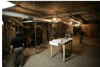
F101906PM-024 [2018-0227-F_M1Hi_j0016_1.JPG] 10/19/2006 Renovations to the Press Briefing room
