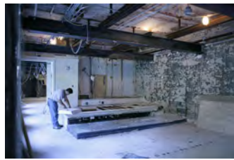
F091806PM-001 [2018-0227-F_M1Hi_j0102_1.JPG] 9/18/2006 Renovations of the Press Briefing Room
