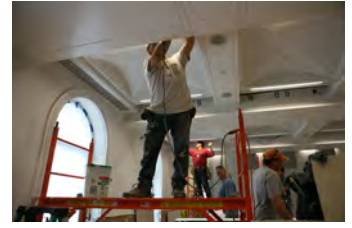
P061907DG-0231 [2018-0227-F_M1Hi_j0221_3.JPG] 6/19/2007 James S. Brady Press Briefing Room renovation
