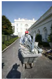
F081506PM-0057 [2018-0227-F_M1Hi_j0246.JPG] 8/15/2006 Press Briefing Room Renovations
