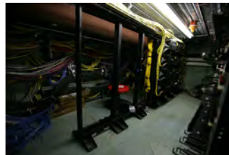
F061207DB-0034 [2018-0227-F_M1Hi_j0228_2.JPG] 6/12/2007 Brady Press Briefing Room Renovations
