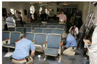
F080306PM-0018 [2018-0227-F_M1Hi_j0113.JPG] 8/3/2006 Clearing out Press Briefing room for renovations.
