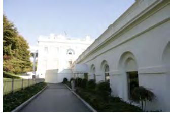
F101806KH-0036 [2018-0227-F_M1Hi_j0216_2.JPG] 10/18/2006 Press Room Renovations
