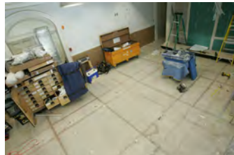
F062007CG-0067 [2018-0227-F_M2Hi_j0049.JPG] 6/20/2007 Work continues on the press briefing room
