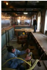
F120206PM-0013 [2018-0227-F_M1Hi_j0168_4.JPG] 12/2/2006 Press Briefing room renovations.
