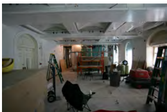
F061207DB-0016 [2018-0227-F_M1Hi_j0113_2.JPG] 6/12/2007 Brady Press Briefing Room Renovations
