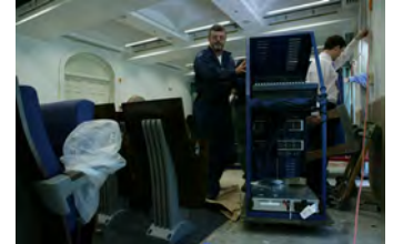
F062207CG-0040 [2018-0227-F_M1Hi_j0120_7.JPG] 6/22/2007 Work continues on the press briefing room
