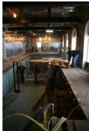
F120206PM-0017 [2018-0227-F_M1Hi_j0176_4.JPG] 12/2/2006 Press Briefing room renovations.
