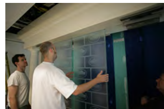
P062107ED-0284 [2018-0227-F_M1Hi_j0195_9.JPG] 6/21/2007 Press Briefing Room Renovations. West Wing.
