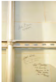
F051607SC-0022 [2018-0227-F_M1Hi_j0100_1.JPG] 5/16/2007 Press Briefing Room Renovations
