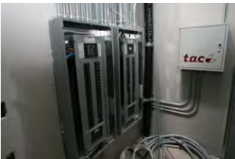
F051607SC-0102 [2018-0227-F_M1Hi_j0034_2.JPG] 5/16/2007 Press Briefing Room Renovations
