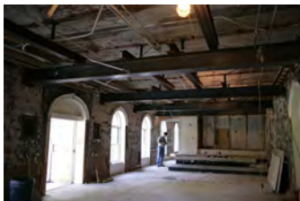
F091806PM-007 [2018-0227-F_M1Hi_j0131_1.JPG] 9/18/2006 Renovations of the Press Briefing Room
