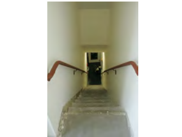
F070207CG-0021 [2018-0227-F_M1Hi_j0127_3.JPG] 7/2/2007 Work nears completion on the press briefing room
