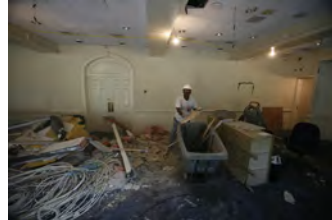
F081506PM-0001 [2018-0227-F_M1Hi_j0134_1.JPG] 8/15/2006 Press Briefing Room Renovations
