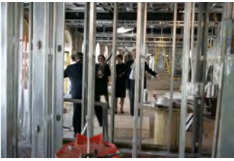
P040207SC-0018 [2018-0227-F_M1Hi_j0001.JPG] 4/2/2007 LB. The Brady Press Room During Renovations.
