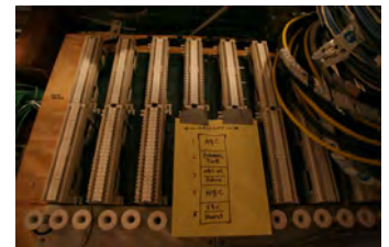
F051607SC-0049 [2018-0227-F_M1Hi_j0183_1.JPG] 5/16/2007 Press Briefing Room Renovations
