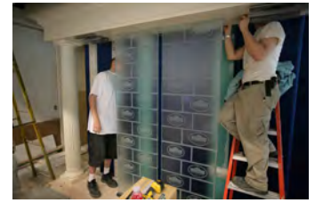
P062107ED-0292 [2018-0227-F_M1Hi_j0211_7.JPG] 6/21/2007 Press Briefing Room Renovations. West Wing.
