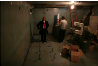
F012507PM-0022 [2018-0227-F_M1Hi_j0057.JPG] 1/25/2007 Press Briefing room renovations.
