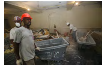
F081506PM-0006 [2018-0227-F_M1Hi_j0144_2.JPG] 8/15/2006 Press Briefing Room Renovations
