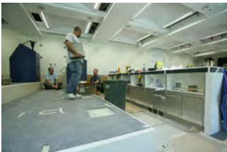
F062707CG-0025 [2018-0227-F_M1Hi_j0199_4.JPG] 6/27/2007 Work continues on the press briefing room
