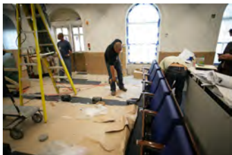
P062107ED-0337 [2018-0227-F_M1Hi_j0046_6.JPG] 6/21/2007 Press Briefing Room Renovations. West Wing.
