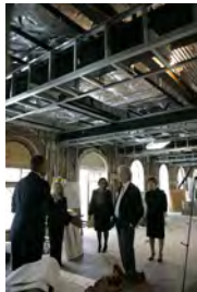
P040207SC-0022 [2018-0227-F_M1Hi_j0024_2.JPG] 4/2/2007 LB. The Brady Press Room During Renovations.
