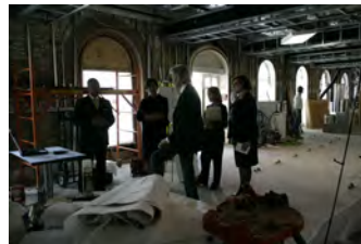
P040207SC-0012 [2018-0227-F_M1Hi_j0225_1.JPG] 4/2/2007 LB. The Brady Press Room During Renovations.
