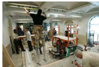
F061507CG-0035 [2018-0227-F_M2Hi_j0225.JPG] 6/15/2007 The Press Briefing Room nears completion
