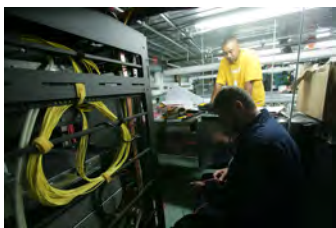
F062007CG-0018 [2018-0227-F_M2Hi_j0206.JPG] 6/20/2007 Work continues on the press briefing room
