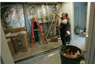
F061507CG-0018 [2018-0227-F_M2Hi_j0191.JPG] 6/15/2007 The Press Briefing Room nears completion
