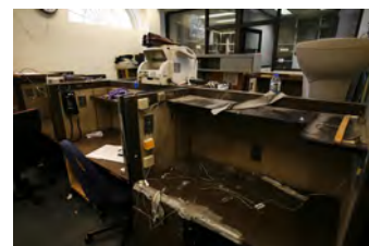
F080406PM-0036 [2018-0227-F_M1Hi_j0208.JPG] 8/4/2006 Clearing out Press Briefing room for renovations.
