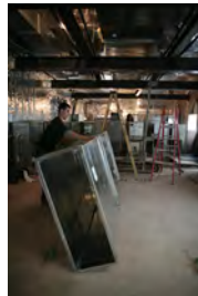
F012507PM-0003 [2018-0227-F_M1Hi_j0019_1.JPG] 1/25/2007 Press Briefing room renovations.
