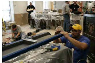
P062107ED-0303 [2018-0227-F_M1Hi_j0233_7.JPG] 6/21/2007 Press Briefing Room Renovations. West Wing.
