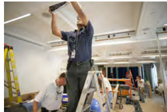
P062107ED-0239 [2018-0227-F_M1Hi_j0105_8.JPG] 6/21/2007 Press Briefing Room Renovations. West Wing.
