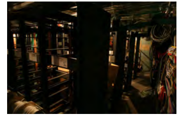
F051607SC-0033 [2018-0227-F_M1Hi_j0147_2.JPG] 5/16/2007 Press Briefing Room Renovations
