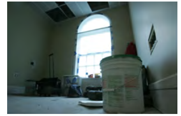
F061507CG-0025 [2018-0227-F_M2Hi_j0205.JPG] 6/15/2007 The Press Briefing Room nears completion
