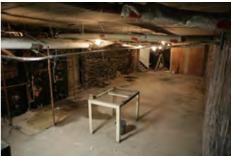
F101806KH-0019 [2018-0227-F_M1Hi_j0182_3.JPG] 10/18/2006 Press Room Renovations
