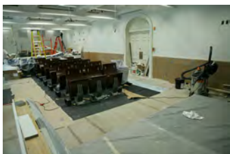
F062207CG-0013 [2018-0227-F_M1Hi_j0066_6.JPG] 6/22/2007 Work continues on the press briefing room
