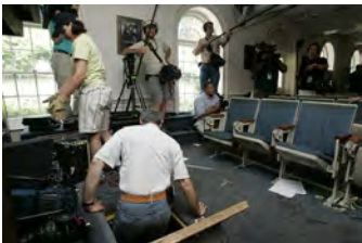
F080306PM-0025 [2018-0227-F_M1Hi_j0127.JPG] 8/3/2006 Clearing out Press Briefing room for renovations.
