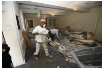
F081506PM-0008 [2018-0227-F_M1Hi_j0148_2.JPG] 8/15/2006 Press Briefing Room Renovations
