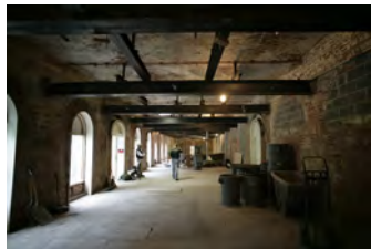
F101906PM-008 [2018-0227-F_M1Hi_j0230_2.JPG] 10/19/2006 Renovations to the Press Briefing room
