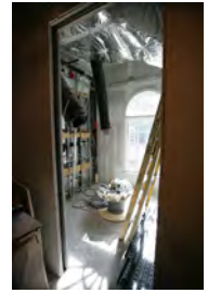
F061207DB-0023 [2018-0227-F_M1Hi_j0162_5.JPG] 6/12/2007 Brady Press Briefing Room Renovations
