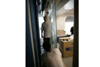
P062107ED-0263 [2018-0227-F_M1Hi_j0153_7.JPG] 6/21/2007 Press Briefing Room Renovations. West Wing.
