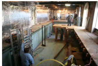
F120206PM-0002 [2018-0227-F_M1Hi_j0146_4.JPG] 12/2/2006 Press Briefing room renovations.
