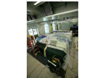
F062707CG-0008 [2018-0227-F_M1Hi_j0125_5.JPG] 6/27/2007 Work continues on the press briefing room
