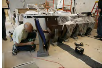
P062107ED-0314 [2018-0227-F_M1Hi_j0255_7.JPG] 6/21/2007 Press Briefing Room Renovations. West Wing.
