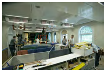
F062907CG-0026 [2018-0227-F_M1Hi_j0022_6.JPG] 6/29/2007 Work nears completion on the press briefing room, Friday June 29, 2007.
