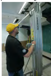
F062007CG-0027 [2018-0227-F_M2Hi_j0224.JPG] 6/20/2007 Work continues on the press briefing room
