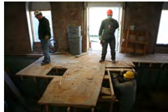
F120206PM-0039 [2018-0227-F_M1Hi_j0220_2.JPG] 12/2/2006 Press Briefing room renovations.
