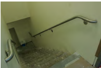
F062807CG-0063 [2018-0227-F_M1Hi_j0203_5.JPG] 6/28/2007 Work continues on the press briefing room
