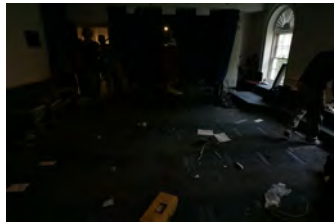
F080306PM-0149 [2018-0227-F_M1Hi_j0120.JPG] 8/3/2006 Clearing out Press Briefing room for renovations.
