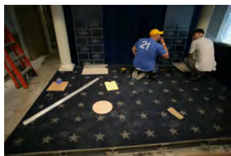
P062107ED-0350 [2018-0227-F_M1Hi_j0072_5.JPG] 6/21/2007 Press Briefing Room Renovations. West Wing.
