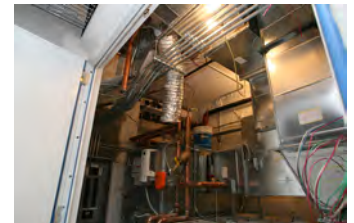
F051607SC-0145 [2018-0227-F_M1Hi_j0120_4.JPG] 5/16/2007 Press Briefing Room Renovations
