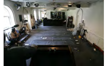
F080306PM-0187 [2018-0227-F_M1Hi_j0196.JPG] 8/3/2006 Clearing out Press Briefing room for renovations.
