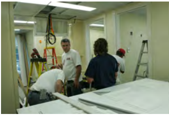
F062907CG-0049 [2018-0227-F_M1Hi_j0189_5.JPG] 6/29/2007 Work nears completion on the press briefing room, Friday June 29, 2007.
