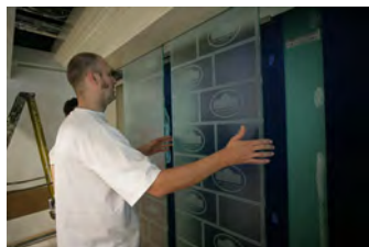
P062107ED-0282 [2018-0227-F_M1Hi_j0191_7.JPG] 6/21/2007 Press Briefing Room Renovations. West Wing.
