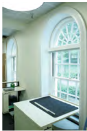
F062907CG-0009 [2018-0227-F_M1Hi_j0243_4.JPG] 6/29/2007 Work nears completion on the press briefing room, Friday June 29, 2007.
