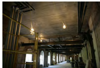
F101806KH-0029 [2018-0227-F_M1Hi_j0202_3.JPG] 10/18/2006 Press Room Renovations
