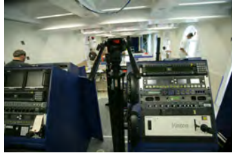
F062807CG-0020 [2018-0227-F_M1Hi_j0117_4.JPG] 6/28/2007 Work continues on the press briefing room
