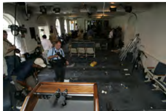
F080306PM-0153 [2018-0227-F_M1Hi_j0128.JPG] 8/3/2006 Clearing out Press Briefing room for renovations.
