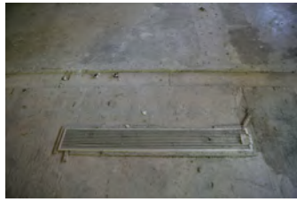
F101806KH-0032 [2018-0227-F_M1Hi_j0208_2.JPG] 10/18/2006 Press Room Renovations
