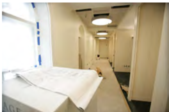
F061207DB-0008 [2018-0227-F_M1Hi_j0065_1.JPG] 6/12/2007 Brady Press Briefing Room Renovations
