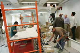
F061507CG-0069 [2018-0227-F_M2Hi_j0038.JPG] 6/15/2007 The Press Briefing Room nears completion
