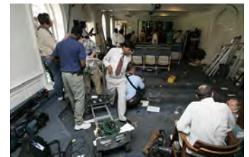
F080306PM-0159 [2018-0227-F_M1Hi_j0140.JPG] 8/3/2006 Clearing out Press Briefing room for renovations.
