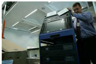
F062207CG-0050 [2018-0227-F_M1Hi_j0140_6.JPG] 6/22/2007 Work continues on the press briefing room
