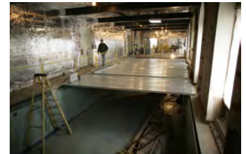
F121506PM-0001 [2018-0227-F_M1Hi_j0105_1.JPG] 12/15/2006 Press Briefing room renovations
