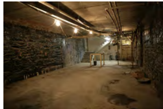
F101806KH-0020 [2018-0227-F_M1Hi_j0184_3.JPG] 10/18/2006 Press Room Renovations
