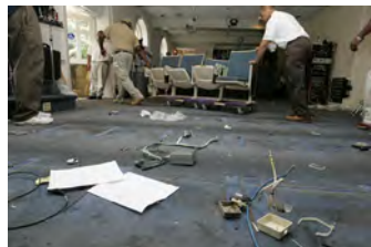
F080306PM-0177 [2018-0227-F_M1Hi_j0176.JPG] 8/3/2006 Clearing out Press Briefing room for renovations.
