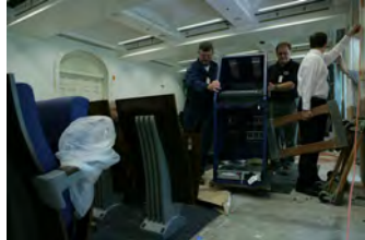
F062207CG-0038 [2018-0227-F_M1Hi_j0116_5.JPG] 6/22/2007 Work continues on the press briefing room
