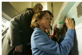
F070207CG-0005 [2018-0227-F_M1Hi_j0037_4.JPG] 7/2/2007 Work nears completion on the press briefing room
