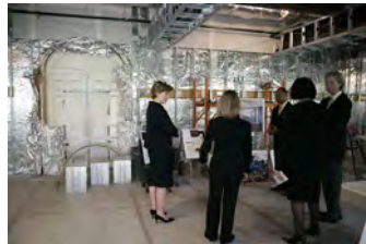
P040207SC-0047 [2018-0227-F_M1Hi_j0202_5.JPG] 4/2/2007 LB. The Brady Press Room During Renovations.
