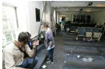
F080306PM-0169 [2018-0227-F_M1Hi_j0160.JPG] 8/3/2006 Clearing out Press Briefing room for renovations.
