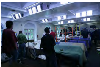
F070507CG-0040 [2018-0227-F_M1Hi_j0181_6.JPG] 7/5/2007 Work nears completion on the press briefing room and the Lower Press office.
