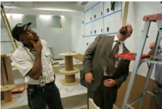
F061507CG-0073 [2018-0227-F_M2Hi_j0046.JPG] 6/15/2007 The Press Briefing Room nears completion
