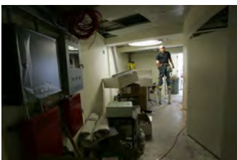
F061507CG-0041 [2018-0227-F_M2Hi_j0237.JPG] 6/15/2007 The Press Briefing Room nears completion
