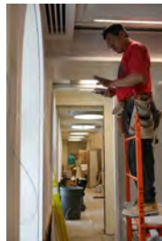
P061907DG-0245 [2018-0227-F_M1Hi_j0249_3.JPG] 6/19/2007 James S. Brady Press Briefing Room renovation
