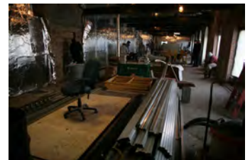
F010907PM-0022 [2018-0227-F_M1Hi_j0158_5.JPG] 1/9/2007 Press Briefing Room Renovations
