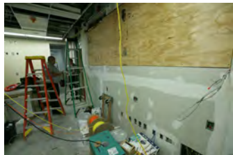
F062707CG-0046 [2018-0227-F_M1Hi_j0041_4.JPG] 6/27/2007 Work continues on the press briefing room
