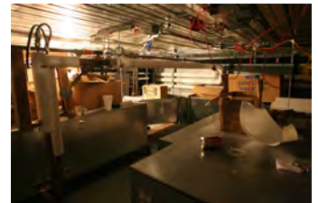
F051607SC-0025 [2018-0227-F_M1Hi_j0116_2.JPG] 5/16/2007 Press Briefing Room Renovations
