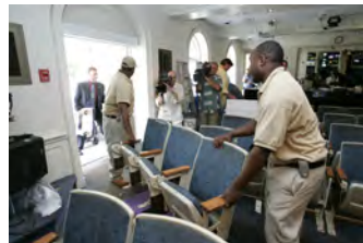
F080306PM-0114 [2018-0227-F_M1Hi_j0050.JPG] 8/3/2006 Clearing out Press Briefing room for renovations.
