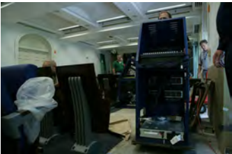
F062207CG-0041 [2018-0227-F_M1Hi_j0122_6.JPG] 6/22/2007 Work continues on the press briefing room
