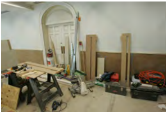
F061907CG-0033 [2018-0227-F_M2Hi_j0243_1.JPG] 6/19/2007 Work continues on the Brady Briefing Room
