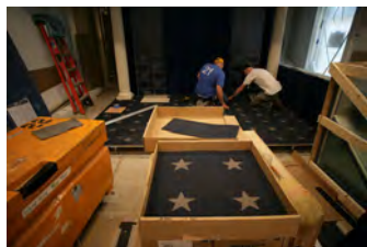
P062107ED-0342 [2018-0227-F_M1Hi_j0056_2.JPG] 6/21/2007 Press Briefing Room Renovations. West Wing.
