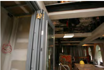
F051607SC-0098 [2018-0227-F_M1Hi_j0026_2.JPG] 5/16/2007 Press Briefing Room Renovations
