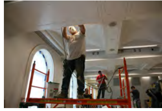
P061907DG-0230 [2018-0227-F_M1Hi_j0219_2.JPG] 6/19/2007 James S. Brady Press Briefing Room renovation
