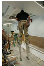
F061507CG-0031 [2018-0227-F_M2Hi_j0217.JPG] 6/15/2007 The Press Briefing Room nears completion
