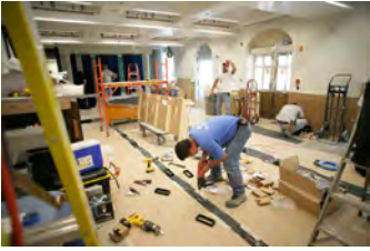
P062107ED-0249 [2018-0227-F_M1Hi_j0125_4.JPG] 6/21/2007 Press Briefing Room Renovations. West Wing.
