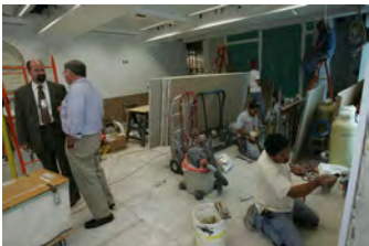
F061507CG-0057 [2018-0227-F_M2Hi_j0014.JPG] 6/15/2007 The Press Briefing Room nears completion
