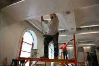
P061907DG-0232 [2018-0227-F_M1Hi_j0223_2.JPG] 6/19/2007 James S. Brady Press Briefing Room renovation
