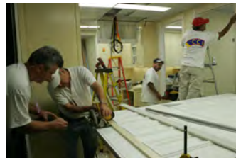
F062907CG-0043 [2018-0227-F_M1Hi_j0177_4.JPG] 6/29/2007 Work nears completion on the press briefing room, Friday June 29, 2007.
