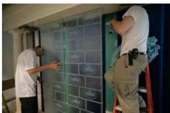
P062107ED-0285 [2018-0227-F_M1Hi_j0197_6.JPG] 6/21/2007 Press Briefing Room Renovations. West Wing.
