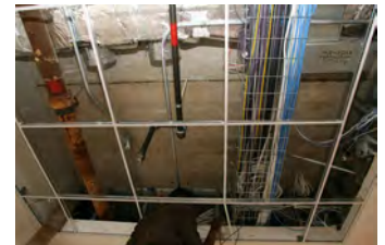
F051607SC-0125 [2018-0227-F_M1Hi_j0080_1.JPG] 5/16/2007 Press Briefing Room Renovations
