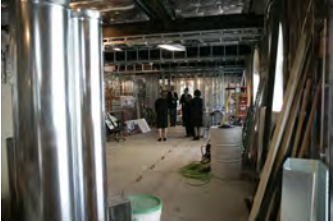
P040207SC-0042 [2018-0227-F_M1Hi_j0142_4.JPG] 4/2/2007 LB. The Brady Press Room During Renovations.
