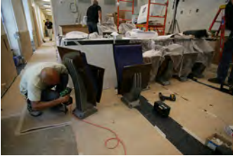
P062107ED-0313 [2018-0227-F_M1Hi_j0253_5.JPG] 6/21/2007 Press Briefing Room Renovations. West Wing.
