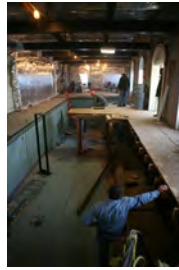
F120206PM-0011 [2018-0227-F_M1Hi_j0164_4.JPG] 12/2/2006 Press Briefing room renovations.
