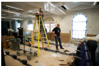
P062107ED-0341 [2018-0227-F_M1Hi_j0054_5.JPG] 6/21/2007 Press Briefing Room Renovations. West Wing.
