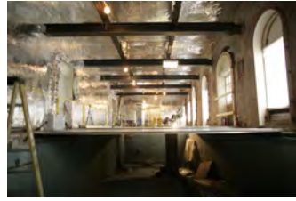
F121506PM-0012 [2018-0227-F_M1Hi_j0127_1.JPG] 12/15/2006 Press Briefing room renovations
