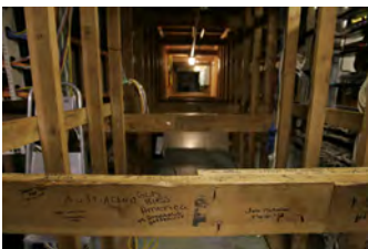
F080306PM-0072 [2018-0227-F_M1Hi_j0221.JPG] 8/3/2006 Clearing out Press Briefing room for renovations.
