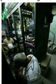
F062807CG-0047 [2018-0227-F_M1Hi_j0171_4.JPG] 6/28/2007 Work continues on the press briefing room
