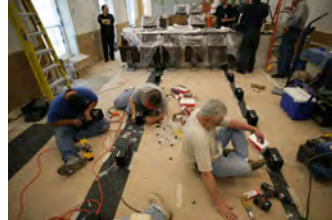
P062107ED-0295 [2018-0227-F_M1Hi_j0217_6.JPG] 6/21/2007 Press Briefing Room Renovations. West Wing.
