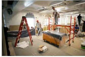
P062107ED-0230 [2018-0227-F_M1Hi_j0087_4.JPG] 6/21/2007 Press Briefing Room Renovations. West Wing.
