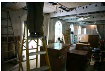
F053107LS-0016 [2018-0227-F_M1Hi_j0088_3.JPG] 5/31/2007 renovation progress of James S. Brady Press Briefing Room
