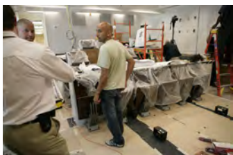
P062107ED-0277 [2018-0227-F_M1Hi_j0181_8.JPG] 6/21/2007 Press Briefing Room Renovations. West Wing.
