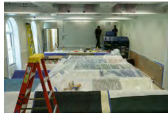
F062707CG-0003 [2018-0227-F_M1Hi_j0105_3.JPG] 6/27/2007 Work continues on the press briefing room
