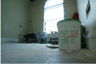
F061507CG-0026 [2018-0227-F_M2Hi_j0207.JPG] 6/15/2007 The Press Briefing Room nears completion
