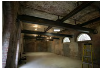
F101906PM-017 [2018-0227-F_M1Hi_j0002_1.JPG] 10/19/2006 Renovations to the Press Briefing room
