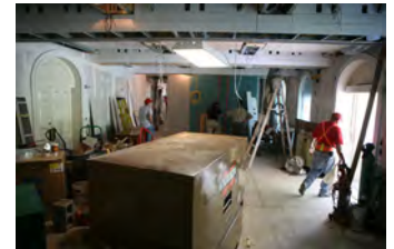
F053107LS-0007 [2018-0227-F_M1Hi_j0070_3.JPG] 5/31/2007 renovation progress of James S. Brady Press Briefing Room
