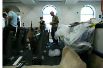
F062207CG-0079 [2018-0227-F_M1Hi_j0198_6.JPG] 6/22/2007 Work continues on the press briefing room
