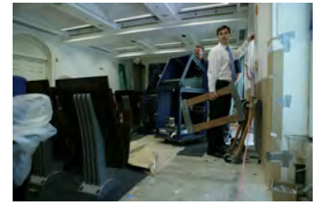
F062207CG-0036 [2018-0227-F_M1Hi_j0112_6.JPG] 6/22/2007 Work continues on the press briefing room
