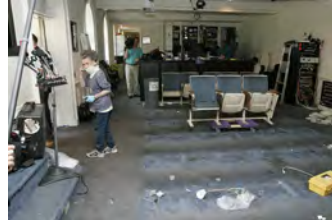
F080306PM-0166 [2018-0227-F_M1Hi_j0154.JPG] 8/3/2006 Clearing out Press Briefing room for renovations.
