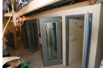
F051607SC-0136 [2018-0227-F_M1Hi_j0102_3.JPG] 5/16/2007 Press Briefing Room Renovations
