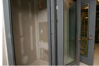
F051607SC-0096 [2018-0227-F_M1Hi_j0022_2.JPG] 5/16/2007 Press Briefing Room Renovations
