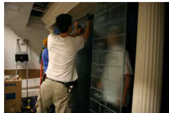
F062107DG-0016 [2018-0227-F_M1Hi_j0116_4.JPG] 6/21/2007 White House Press Briefing Room renovations Thursday, June 21, 2007. White House photo by Debra Gulbas
