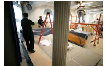
P062107ED-0224 [2018-0227-F_M1Hi_j0075_3.JPG] 6/21/2007 Press Briefing Room Renovations. West Wing.
