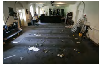
F080306PM-0183 [2018-0227-F_M1Hi_j0188.JPG] 8/3/2006 Clearing out Press Briefing room for renovations.
