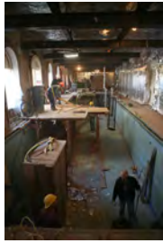
F120206PM-0029 [2018-0227-F_M1Hi_j0200_4.JPG] 12/2/2006 Press Briefing room renovations.
