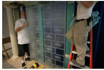
P062107ED-0290 [2018-0227-F_M1Hi_j0207_10.JPG] 6/21/2007 Press Briefing Room Renovations. West Wing.
