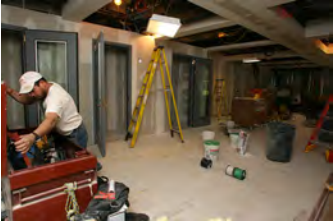
F051607SC-0094 [2018-0227-F_M1Hi_j0018_3.JPG] 5/16/2007 Press Briefing Room Renovations
