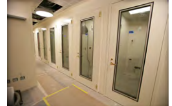
F061207DB-0047 [2018-0227-F_M1Hi_j0058_4.JPG] 6/12/2007 Brady Press Briefing Room Renovations
