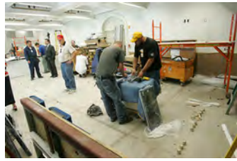
F062007CG-0079 [2018-0227-F_M2Hi_j0073.JPG] 6/20/2007 Work continues on the press briefing room
