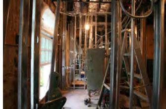
F051607SC-0075 [2018-0227-F_M1Hi_j0235_1.JPG] 5/16/2007 Press Briefing Room Renovations
