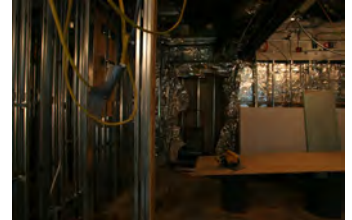
F051607SC-0077 [2018-0227-F_M1Hi_j0239_1.JPG] 5/16/2007 Press Briefing Room Renovations
