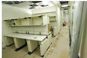
F062007CG-0051 [2018-0227-F_M2Hi_j0017.JPG] 6/20/2007 Work continues on the press briefing room
