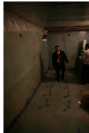
F012507PM-0023 [2018-0227-F_M1Hi_j0059.JPG] 1/25/2007 Press Briefing room renovations.
