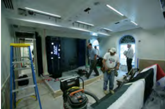
F062707CG-0037 [2018-0227-F_M1Hi_j0247_6.JPG] 6/27/2007 Work continues on the press briefing room
