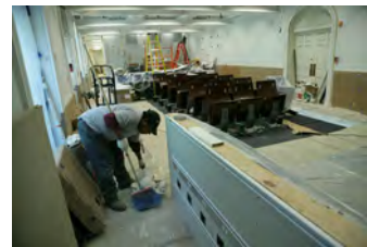
F062207CG-0012 [2018-0227-F_M1Hi_j0064_6.JPG] 6/22/2007 Work continues on the press briefing room
