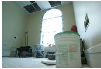
F061507CG-0024 [2018-0227-F_M2Hi_j0203.JPG] 6/15/2007 The Press Briefing Room nears completion
