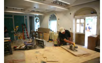
P061907DG-0215 [2018-0227-F_M1Hi_j0189_2.JPG] 6/19/2007 James S. Brady Press Briefing Room renovation
