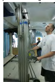
F062007CG-0029 [2018-0227-F_M2Hi_j0228.JPG] 6/20/2007 Work continues on the press briefing room
