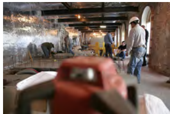
F010907PM-0016 [2018-0227-F_M1Hi_j0146_5.JPG] 1/9/2007 Press Briefing Room Renovations
