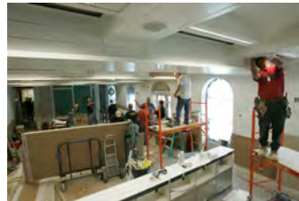
F061907CG-0003 [2018-0227-F_M2Hi_j0183_1.JPG] 6/19/2007 Work continues on the Brady Briefing Room
