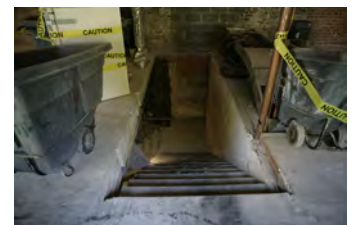
F101806KH-0010 [2018-0227-F_M1Hi_j0164_3.JPG] 10/18/2006 Press Room Renovations
