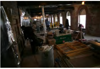
F010907PM-0023 [2018-0227-F_M1Hi_j0160_5.JPG] 1/9/2007 Press Briefing Room Renovations
