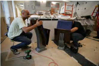
P062107ED-0321 [2018-0227-F_M1Hi_j0014_8.JPG] 6/21/2007 Press Briefing Room Renovations. West Wing.
