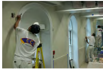
F062807CG-0056 [2018-0227-F_M1Hi_j0189_4.JPG] 6/28/2007 Work continues on the press briefing room
