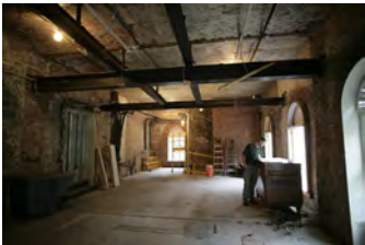
F101906PM-003 [2018-0227-F_M1Hi_j0203_1.JPG] 10/19/2006 Renovations to the Press Briefing room
