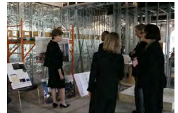
P040207SC-0053 [2018-0227-F_M1Hi_j0238_4.JPG] 4/2/2007 LB. The Brady Press Room During Renovations.
