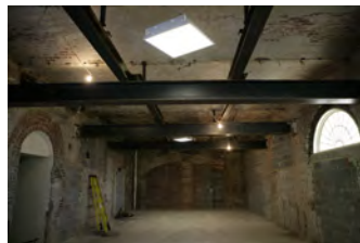
F101806KH-0001 [2018-0227-F_M1Hi_j0146_3.JPG] 10/18/2006 Press Room Renovations
