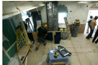
F062007CG-0088 [2018-0227-F_M2Hi_j0091.JPG] 6/20/2007 Work continues on the press briefing room
