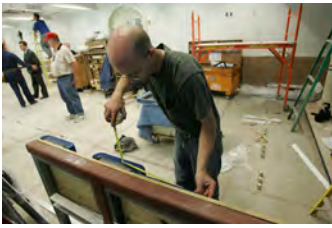
F062007CG-0078 [2018-0227-F_M2Hi_j0071.JPG] 6/20/2007 Work continues on the press briefing room
