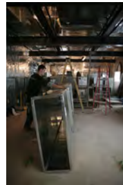
F012507PM-0004 [2018-0227-F_M1Hi_j0021_1.JPG] 1/25/2007 Press Briefing room renovations.
