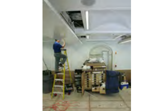
F062007CG-0072 [2018-0227-F_M2Hi_j0059.JPG] 6/20/2007 Work continues on the press briefing room
