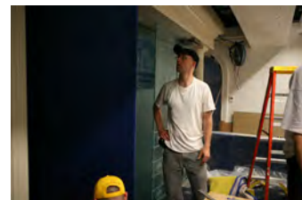
F062107DG-0003 [2018-0227-F_M1Hi_j0103_2.JPG] 6/21/2007 White House Press Briefing Room renovations Thursday, June 21, 2007. White House photo by Debra Gulbas
