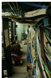
F062807CG-0037 [2018-0227-F_M1Hi_j0151_4.JPG] 6/28/2007 Work continues on the press briefing room
