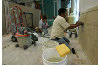
F061507CG-0003 [2018-0227-F_M2Hi_j0161.JPG] 6/15/2007 The Press Briefing Room nears completion
