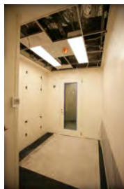
F061207DB-0002 [2018-0227-F_M1Hi_j0017_3.JPG] 6/12/2007 Brady Press Briefing Room Renovations
