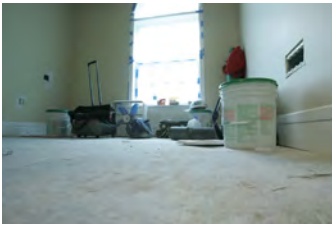
F061507CG-0022 [2018-0227-F_M2Hi_j0199.JPG] 6/15/2007 The Press Briefing Room nears completion
