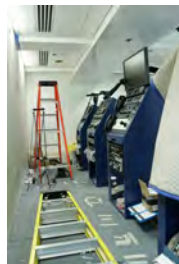
F062907CG-0022 [2018-0227-F_M1Hi_j0014_6.JPG] 6/29/2007 Work nears completion on the press briefing room, Friday June 29, 2007.
