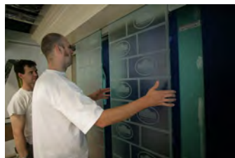
P062107ED-0283 [2018-0227-F_M1Hi_j0193_7.JPG] 6/21/2007 Press Briefing Room Renovations. West Wing.
