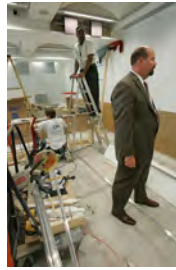
F061507CG-0067 [2018-0227-F_M2Hi_j0034.JPG] 6/15/2007 The Press Briefing Room nears completion
