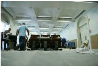
F062207CG-0073 [2018-0227-F_M1Hi_j0186_6.JPG] 6/22/2007 Work continues on the press briefing room
