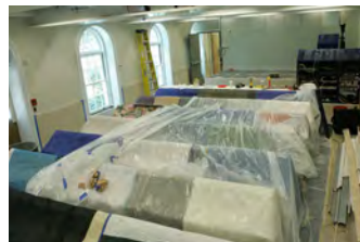
F062707CG-0011 [2018-0227-F_M1Hi_j0137_2.JPG] 6/27/2007 Work continues on the press briefing room
