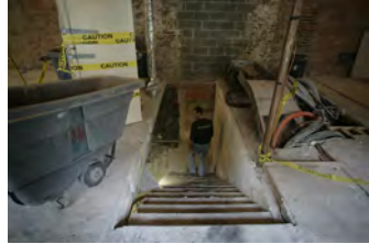
F101906PM-020 [2018-0227-F_M1Hi_j0008_1.JPG] 10/19/2006 Renovations to the Press Briefing room
