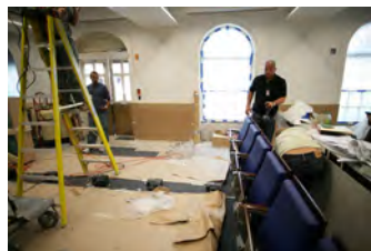
P062107ED-0335 [2018-0227-F_M1Hi_j0042_4.JPG] 6/21/2007 Press Briefing Room Renovations. West Wing.
