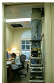
F070507CG-0002 [2018-0227-F_M1Hi_j0105_6.JPG] 7/5/2007 Work nears completion on the press briefing room and Lower Press office.
