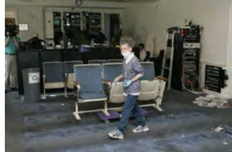
F080306PM-0165 [2018-0227-F_M1Hi_j0152.JPG] 8/3/2006 Clearing out Press Briefing room for renovations.
