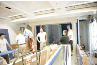
P062107ED-0257 [2018-0227-F_M1Hi_j0141_5.JPG] 6/21/2007 Press Briefing Room Renovations. West Wing.
