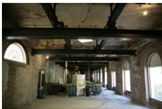
F101806KH-0003 [2018-0227-F_M1Hi_j0150_3.JPG] 10/18/2006 Press Room Renovations
