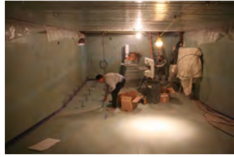
F012507PM-0015 [2018-0227-F_M1Hi_j0043.JPG] 1/25/2007 Press Briefing room renovations.
