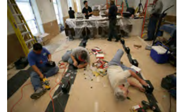
P062107ED-0296 [2018-0227-F_M1Hi_j0219_6.JPG] 6/21/2007 Press Briefing Room Renovations. West Wing.
