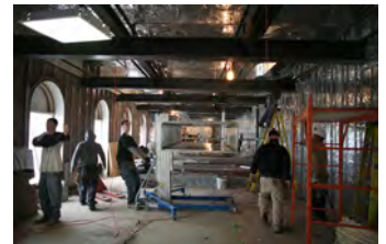
F012507PM-0029 [2018-0227-F_M1Hi_j0071.JPG] 1/25/2007 Press Briefing room renovations.
