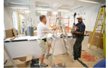
P062107ED-0236 [2018-0227-F_M1Hi_j0099_5.JPG] 6/21/2007 Press Briefing Room Renovations. West Wing.
