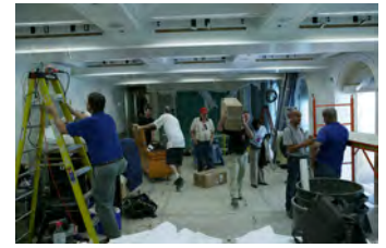
F062007CG-0061 [2018-0227-F_M2Hi_j0037.JPG] 6/20/2007 Work continues on the press briefing room
