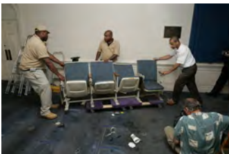
F080306PM-0176 [2018-0227-F_M1Hi_j0174.JPG] 8/3/2006 Clearing out Press Briefing room for renovations.
