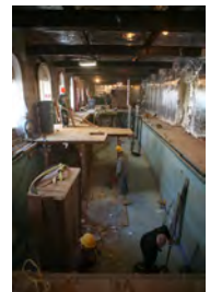
F120206PM-0024 [2018-0227-F_M1Hi_j0190_4.JPG] 12/2/2006 Press Briefing room renovations.
