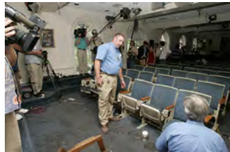
F080306PM-0010 [2018-0227-F_M1Hi_j0097.JPG] 8/3/2006 Clearing out Press Briefing room for renovations.
