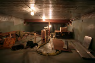
F012507PM-0018 [2018-0227-F_M1Hi_j0049.JPG] 1/25/2007 Press Briefing room renovations.
