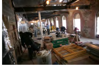
F010907PM-0028 [2018-0227-F_M1Hi_j0170_5.JPG] 1/9/2007 Press Briefing Room Renovations
