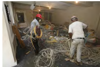
F081506PM-0009 [2018-0227-F_M1Hi_j0150_2.JPG] 8/15/2006 Press Briefing Room Renovations
