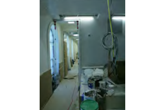
F062207CG-0030 [2018-0227-F_M1Hi_j0100_5.JPG] 6/22/2007 Work continues on the press briefing room
