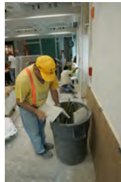
F061507CG-0059 [2018-0227-F_M2Hi_j0018.JPG] 6/15/2007 The Press Briefing Room nears completion
