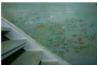
F062007CG-0022 [2018-0227-F_M2Hi_j0214.JPG] 6/20/2007 Work continues on the press briefing room
