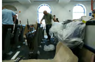
F062207CG-0078 [2018-0227-F_M1Hi_j0196_7.JPG] 6/22/2007 Work continues on the press briefing room
