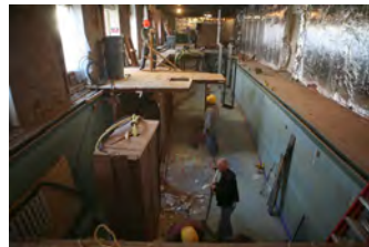
F120206PM-0023 [2018-0227-F_M1Hi_j0188_4.JPG] 12/2/2006 Press Briefing room renovations.
