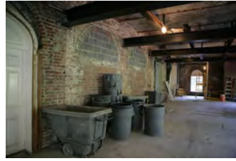
F101806KH-0013 [2018-0227-F_M1Hi_j0170_3.JPG] 10/18/2006 Press Room Renovations
