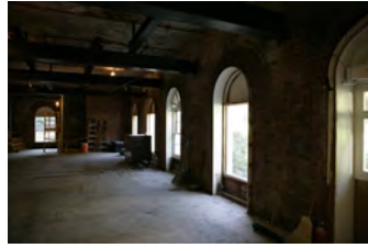
F101806KH-0012 [2018-0227-F_M1Hi_j0168_3.JPG] 10/18/2006 Press Room Renovations
