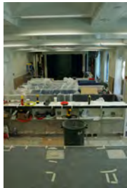
F062707CG-0017 [2018-0227-F_M1Hi_j0167_5.JPG] 6/27/2007 Work continues on the press briefing room
