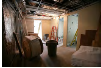
F061207DB-0021 [2018-0227-F_M1Hi_j0150_7.JPG] 6/12/2007 Brady Press Briefing Room Renovations
