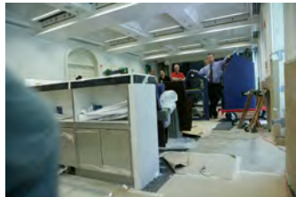
F062207CG-0042 [2018-0227-F_M1Hi_j0124_7.JPG] 6/22/2007 Work continues on the press briefing room
