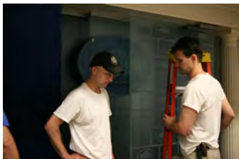
F062107DG-0011 [2018-0227-F_M1Hi_j0111_2.JPG] 6/21/2007 White House Press Briefing Room renovations Thursday, June 21, 2007. White House photo by Debra Gulbas
