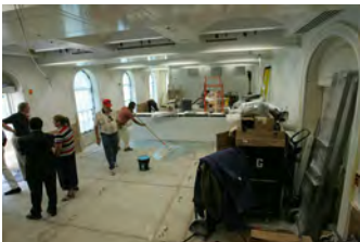
F062007CG-0090 [2018-0227-F_M2Hi_j0095.JPG] 6/20/2007 Work continues on the press briefing room
