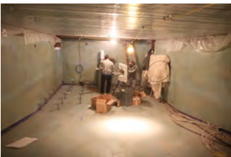
F012507PM-0010 [2018-0227-F_M1Hi_j0033.JPG] 1/25/2007 Press Briefing room renovations.
