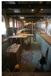
F120206PM-0026 [2018-0227-F_M1Hi_j0194_4.JPG] 12/2/2006 Press Briefing room renovations.
