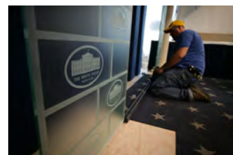
P062107ED-0356 [2018-0227-F_M1Hi_j0084_4.JPG] 6/21/2007 Press Briefing Room Renovations. West Wing.
