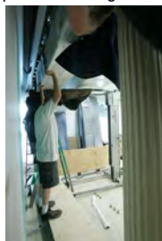
F062007CG-0035 [2018-0227-F_M2Hi_j0240.JPG] 6/20/2007 Work continues on the press briefing room
