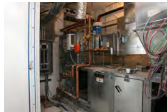
F051607SC-0144 [2018-0227-F_M1Hi_j0118_3.JPG] 5/16/2007 Press Briefing Room Renovations
