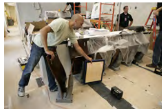
P062107ED-0307 [2018-0227-F_M1Hi_j0241_7.JPG] 6/21/2007 Press Briefing Room Renovations. West Wing.
