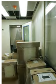
F061507CG-0049 [2018-0227-F_M2Hi_j0253.JPG] 6/15/2007 The Press Briefing Room nears completion
