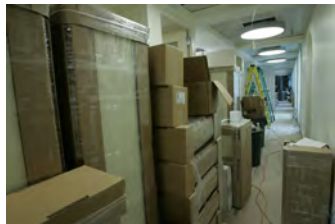
F061507CG-0050 [2018-0227-F_M2Hi_j0255.JPG] 6/15/2007 The Press Briefing Room nears completion
