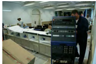
F062207CG-0047 [2018-0227-F_M1Hi_j0134_5.JPG] 6/22/2007 Work continues on the press briefing room
