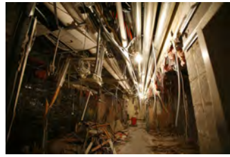
F081506PM-0038 [2018-0227-F_M1Hi_j0208_1.JPG] 8/15/2006 Press Briefing Room Renovations
