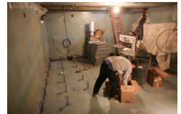
F012507PM-0009 [2018-0227-F_M1Hi_j0031.JPG] 1/25/2007 Press Briefing room renovations.
