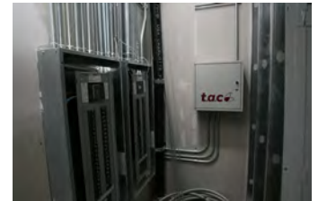
F051607SC-0101 [2018-0227-F_M1Hi_j0032_2.JPG] 5/16/2007 Press Briefing Room Renovations
