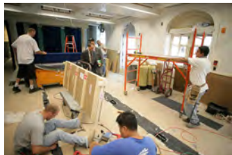
P062107ED-0202 [2018-0227-F_M1Hi_j0031_3.JPG] 6/21/2007 Press Briefing Room Renovations. West Wing.
