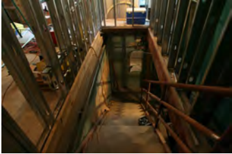
F051607SC-0054 [2018-0227-F_M1Hi_j0193_1.JPG] 5/16/2007 Press Briefing Room Renovations
