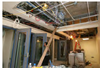
F051607SC-0128 [2018-0227-F_M1Hi_j0086_1.JPG] 5/16/2007 Press Briefing Room Renovations
