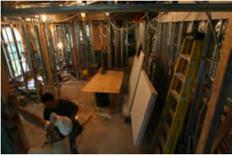
F051607SC-0070 [2018-0227-F_M1Hi_j0225_2.JPG] 5/16/2007 Press Briefing Room Renovations
