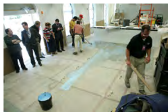
F062007CG-0095 [2018-0227-F_M2Hi_j0105.JPG] 6/20/2007 Work continues on the press briefing room
