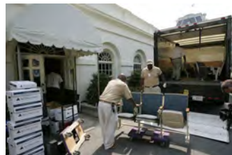
F080306PM-0138 [2018-0227-F_M1Hi_j0098.JPG] 8/3/2006 Clearing out Press Briefing room for renovations.
