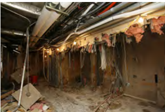
F081506PM-0028 [2018-0227-F_M1Hi_j0188_2.JPG] 8/15/2006 Press Briefing Room Renovations
