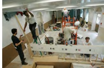
F061507CG-0007 [2018-0227-F_M2Hi_j0169.JPG] 6/15/2007 The Press Briefing Room nears completion
