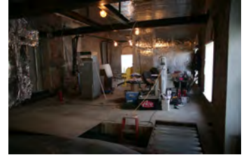
F010907PM-0010 [2018-0227-F_M1Hi_j0134_2.JPG] 1/9/2007 Press Briefing Room Renovations
