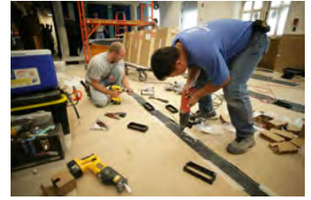
P062107ED-0252 [2018-0227-F_M1Hi_j0131_8.JPG] 6/21/2007 Press Briefing Room Renovations. West Wing.
