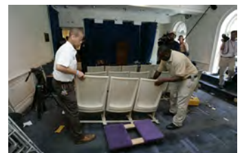
F080306PM-0119 [2018-0227-F_M1Hi_j0060.JPG] 8/3/2006 Clearing out Press Briefing room for renovations.
