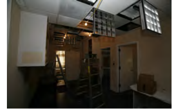
F081506PM-0043 [2018-0227-F_M1Hi_j0218_1.JPG] 8/15/2006 Press Briefing Room Renovations
