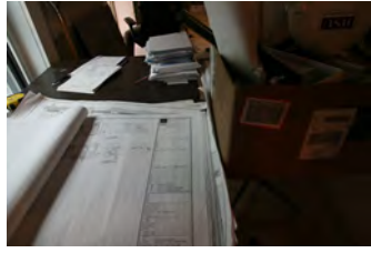
F051607SC-0091 [2018-0227-F_M1Hi_j0012_2.JPG] 5/16/2007 Press Briefing Room Renovations
