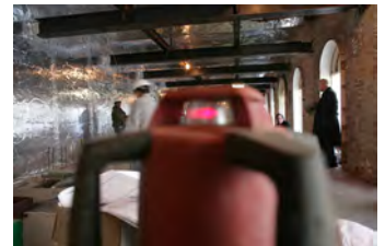
F010907PM-0018 [2018-0227-F_M1Hi_j0150_5.JPG] 1/9/2007 Press Briefing Room Renovations
