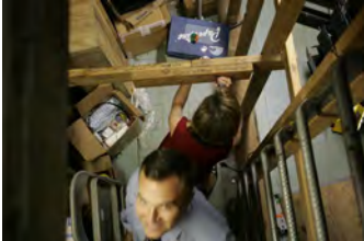
F080306PM-0044 [2018-0227-F_M1Hi_j0165.JPG] 8/3/2006 Clearing out Press Briefing room for renovations.
