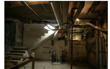
F101806KH-0022 [2018-0227-F_M1Hi_j0188_3.JPG] 10/18/2006 Press Room Renovations
