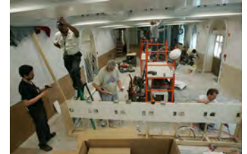
F061507CG-0009 [2018-0227-F_M2Hi_j0173.JPG] 6/15/2007 The Press Briefing Room nears completion
