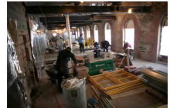
F010907PM-0026 [2018-0227-F_M1Hi_j0166_5.JPG] 1/9/2007 Press Briefing Room Renovations
