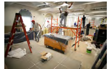
P062107ED-0228 [2018-0227-F_M1Hi_j0083_2.JPG] 6/21/2007 Press Briefing Room Renovations. West Wing.
