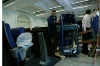
F062207CG-0039 [2018-0227-F_M1Hi_j0118_7.JPG] 6/22/2007 Work continues on the press briefing room
