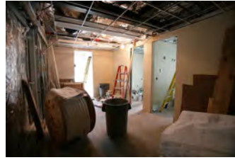
F061207DB-0022 [2018-0227-F_M1Hi_j0156_6.JPG] 6/12/2007 Brady Press Briefing Room Renovations
