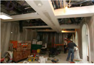
F051607SC-0110 [2018-0227-F_M1Hi_j0050_2.JPG] 5/16/2007 Press Briefing Room Renovations
