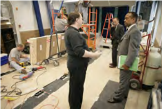
P062107ED-0209 [2018-0227-F_M1Hi_j0045_2.JPG] 6/21/2007 Press Briefing Room Renovations. West Wing.
