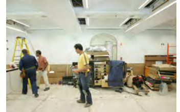
F062007CG-0085 [2018-0227-F_M2Hi_j0085.JPG] 6/20/2007 Work continues on the press briefing room
