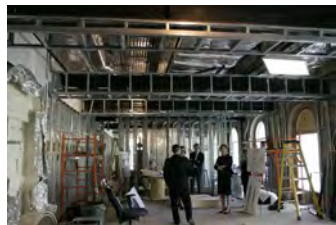
P040207SC-0035 [2018-0227-F_M1Hi_j0102_2.JPG] 4/2/2007 LB. The Brady Press Room During Renovations.
