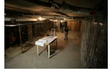
F101906PM-022 [2018-0227-F_M1Hi_j0012_1.JPG] 10/19/2006 Renovations to the Press Briefing room
