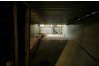
F121506PM-0018 [2018-0227-F_M1Hi_j0139_1.JPG] 12/15/2006 Press Briefing room renovations
