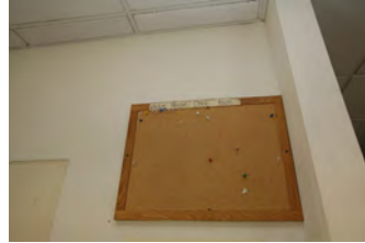
F081506PM-0042 [2018-0227-F_M1Hi_j0216_1.JPG] 8/15/2006 Press Briefing Room Renovations
