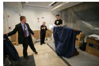
P062207ED-0043 [2018-0227-F_M1Hi_j0166_6.JPG] 6/22/2007 Press Briefing Room rennovations
