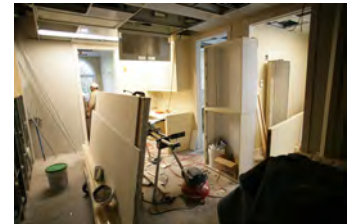
P062107ED-0220 [2018-0227-F_M1Hi_j0067_4.JPG] 6/21/2007 Press Briefing Room Renovations. West Wing.
