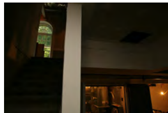
F051607SC-0148 [2018-0227-F_M1Hi_j0126_3.JPG] 5/16/2007 Press Briefing Room Renovations
