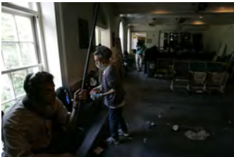
F080306PM-0168 [2018-0227-F_M1Hi_j0158.JPG] 8/3/2006 Clearing out Press Briefing room for renovations.
