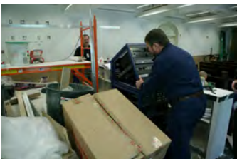
F062207CG-0049 [2018-0227-F_M1Hi_j0138_7.JPG] 6/22/2007 Work continues on the press briefing room
