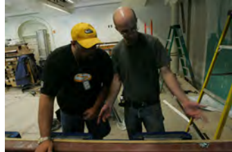
F062007CG-0083 [2018-0227-F_M2Hi_j0081.JPG] 6/20/2007 Work continues on the press briefing room
