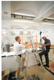
P062107ED-0237 [2018-0227-F_M1Hi_j0101_7.JPG] 6/21/2007 Press Briefing Room Renovations. West Wing.
