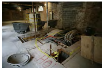
F101906PM-012 [2018-0227-F_M1Hi_j0246_1.JPG] 10/19/2006 Renovations to the Press Briefing room
