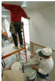
F061907CG-0009 [2018-0227-F_M2Hi_j0195_1.JPG] 6/19/2007 Work continues on the Brady Briefing Room
