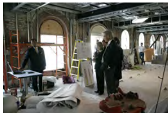
P040207SC-0015 [2018-0227-F_M1Hi_j0238_3.JPG] 4/2/2007 LB. The Brady Press Room During Renovations.
