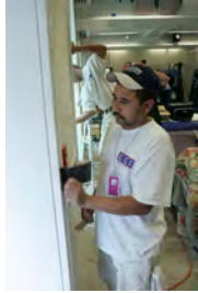
F062807CG-0019 [2018-0227-F_M1Hi_j0115_3.JPG] 6/28/2007 Work continues on the press briefing room
