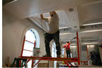
P061907DG-0233 [2018-0227-F_M1Hi_j0225_3.JPG] 6/19/2007 James S. Brady Press Briefing Room renovation
