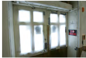
F061907CG-0035 [2018-0227-F_M2Hi_j0247_1.JPG] 6/19/2007 Work continues on the Brady Briefing Room
