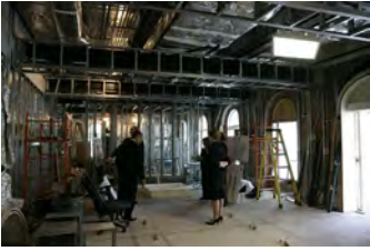
P040207SC-0038 [2018-0227-F_M1Hi_j0120_2.JPG] 4/2/2007 LB. The Brady Press Room During Renovations.
