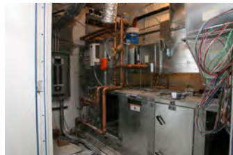
F051607SC-0143 [2018-0227-F_M1Hi_j0116_3.JPG] 5/16/2007 Press Briefing Room Renovations
