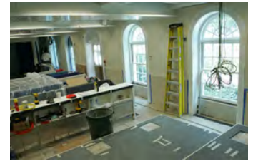
F062707CG-0016 [2018-0227-F_M1Hi_j0163_3.JPG] 6/27/2007 Work continues on the press briefing room
