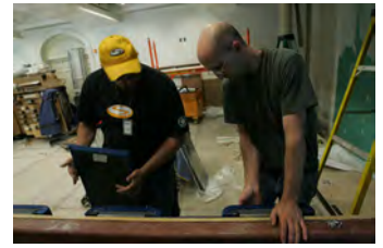
F062007CG-0081 [2018-0227-F_M2Hi_j0077.JPG] 6/20/2007 Work continues on the press briefing room
