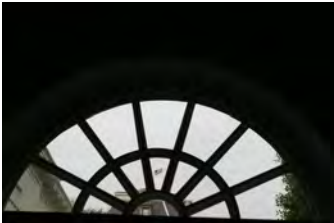
F051607SC-0062 [2018-0227-F_M1Hi_j0209_1.JPG] 5/16/2007 Press Briefing Room Renovations
