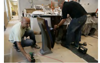
P062107ED-0316 [2018-0227-F_M1Hi_j0004_7.JPG] 6/21/2007 Press Briefing Room Renovations. West Wing.
