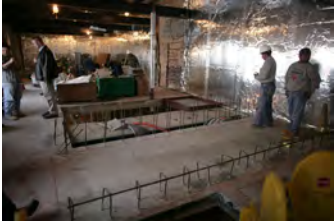
F010907PM-0007 [2018-0227-F_M1Hi_j0128_1.JPG] 1/9/2007 Press Briefing Room Renovations
