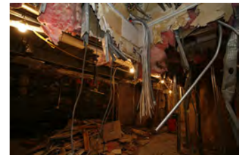
F081506PM-0031 [2018-0227-F_M1Hi_j0194_2.JPG] 8/15/2006 Press Briefing Room Renovations
