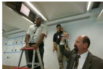
F061507CG-0063 [2018-0227-F_M2Hi_j0026.JPG] 6/15/2007 The Press Briefing Room nears completion
