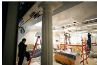
P062107ED-0226 [2018-0227-F_M1Hi_j0079_4.JPG] 6/21/2007 Press Briefing Room Renovations. West Wing.
