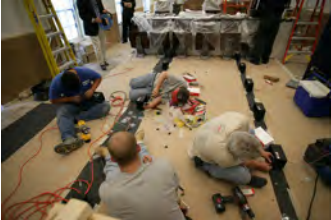
P062107ED-0293 [2018-0227-F_M1Hi_j0213_8.JPG] 6/21/2007 Press Briefing Room Renovations. West Wing.
