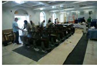
F062207CG-0074 [2018-0227-F_M1Hi_j0188_6.JPG] 6/22/2007 Work continues on the press briefing room
