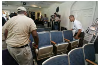
F080306PM-0110 [2018-0227-F_M1Hi_j0042.JPG] 8/3/2006 Clearing out Press Briefing room for renovations.
