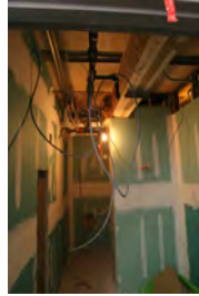
F051607SC-0115 [2018-0227-F_M1Hi_j0060_2.JPG] 5/16/2007 Press Briefing Room Renovations
