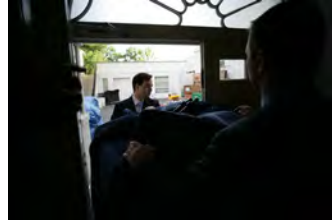
P062207ED-0022 [2018-0227-F_M1Hi_j0154_6.JPG] 6/22/2007 Press Briefing Room rennovations
