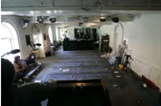
F080306PM-0184 [2018-0227-F_M1Hi_j0190.JPG] 8/3/2006 Clearing out Press Briefing room for renovations.
