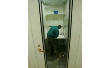
F062007CG-0053 [2018-0227-F_M2Hi_j0021.JPG] 6/20/2007 Work continues on the press briefing room
