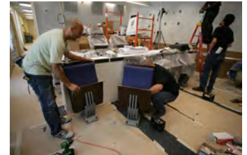
P062107ED-0324 [2018-0227-F_M1Hi_j0020_5.JPG] 6/21/2007 Press Briefing Room Renovations. West Wing.
