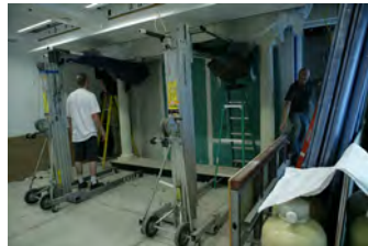
F062007CG-0047 [2018-0227-F_M2Hi_j0009.JPG] 6/20/2007 Work continues on the press briefing room
