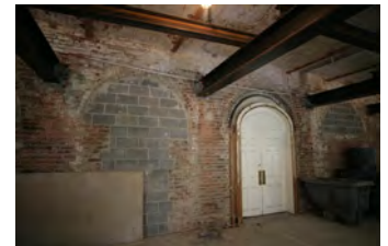
F101906PM-030 [2018-0227-F_M1Hi_j0028_1.JPG] 10/19/2006 Renovations to the Press Briefing room
