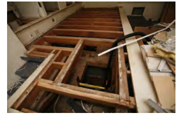
F081506PM-0019 [2018-0227-F_M1Hi_j0170_2.JPG] 8/15/2006 Press Briefing Room Renovations
