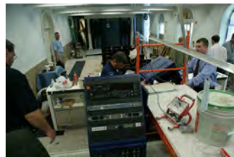
F062207CG-0051 [2018-0227-F_M1Hi_j0142_8.JPG] 6/22/2007 Work continues on the press briefing room
