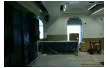
F062207CG-0076 [2018-0227-F_M1Hi_j0192_7.JPG] 6/22/2007 Work continues on the press briefing room
