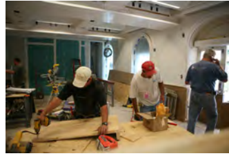
P061907DG-0210 [2018-0227-F_M1Hi_j0179_2.JPG] 6/19/2007 James S. Brady Press Briefing Room renovation
