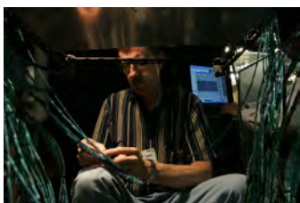
F062807CG-0039 [2018-0227-F_M1Hi_j0155_5.JPG] 6/28/2007 Work continues on the press briefing room
