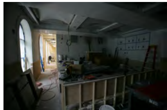
F061207DB-0053 [2018-0227-F_M1Hi_j0094_3.JPG] 6/12/2007 Brady Press Briefing Room Renovations
