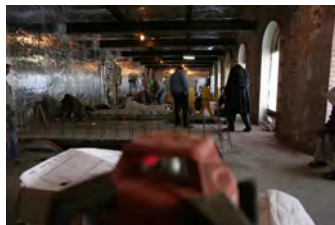
F010907PM-0020 [2018-0227-F_M1Hi_j0154_5.JPG] 1/9/2007 Press Briefing Room Renovations
