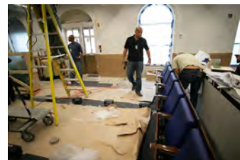
P062107ED-0336 [2018-0227-F_M1Hi_j0044_5.JPG] 6/21/2007 Press Briefing Room Renovations. West Wing.
