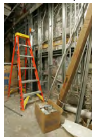
F061507CG-0019 [2018-0227-F_M2Hi_j0193.JPG] 6/15/2007 The Press Briefing Room nears completion
