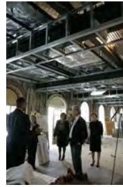
P040207SC-0020 [2018-0227-F_M1Hi_j0013_1.JPG] 4/2/2007 LB. The Brady Press Room During Renovations.
