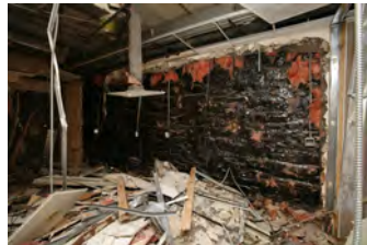
F081506PM-0025 [2018-0227-F_M1Hi_j0182_2.JPG] 8/15/2006 Press Briefing Room Renovations
