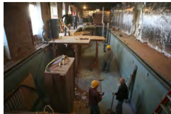
F120206PM-0022 [2018-0227-F_M1Hi_j0186_4.JPG] 12/2/2006 Press Briefing room renovations.
