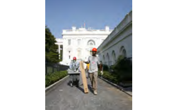
F081506PM-0051 [2018-0227-F_M1Hi_j0234_1.JPG] 8/15/2006 Press Briefing Room Renovations
