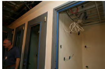
F051607SC-0139 [2018-0227-F_M1Hi_j0108_2.JPG] 5/16/2007 Press Briefing Room Renovations
