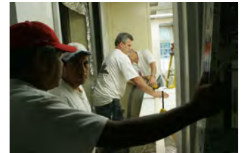
F062907CG-0040 [2018-0227-F_M1Hi_j0171_5.JPG] 6/29/2007 Work nears completion on the press briefing room, Friday June 29, 2007.
