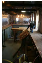
F120206PM-0015 [2018-0227-F_M1Hi_j0172_4.JPG] 12/2/2006 Press Briefing room renovations.
