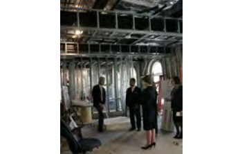
P040207SC-0044 [2018-0227-F_M1Hi_j0150_6.JPG] 4/2/2007 LB. The Brady Press Room During Renovations.
