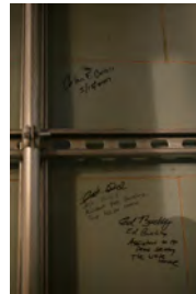
F051607SC-0016 [2018-0227-F_M1Hi_j0066_2.JPG] 5/16/2007 Press Briefing Room Renovations
