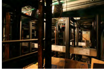
F051607SC-0035 [2018-0227-F_M1Hi_j0151_2.JPG] 5/16/2007 Press Briefing Room Renovations
