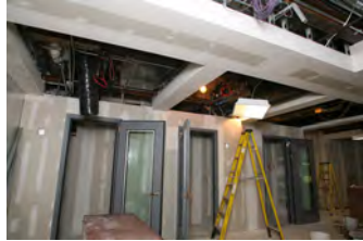
F051607SC-0095 [2018-0227-F_M1Hi_j0020_2.JPG] 5/16/2007 Press Briefing Room Renovations
