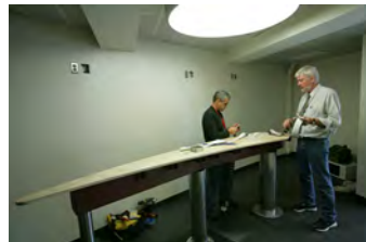
F070207CG-0030 [2018-0227-F_M1Hi_j0093_1.JPG] 7/2/2007 Work nears completion on the press briefing room
