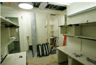
F062007CG-0054 [2018-0227-F_M2Hi_j0023.JPG] 6/20/2007 Work continues on the press briefing room
