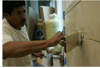
F061507CG-0004 [2018-0227-F_M2Hi_j0163.JPG] 6/15/2007 The Press Briefing Room nears completion
