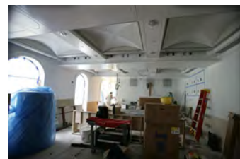
F061207DB-0019 [2018-0227-F_M1Hi_j0131_3.JPG] 6/12/2007 Brady Press Briefing Room Renovations
