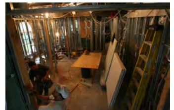
F051607SC-0069 [2018-0227-F_M1Hi_j0223_1.JPG] 5/16/2007 Press Briefing Room Renovations
