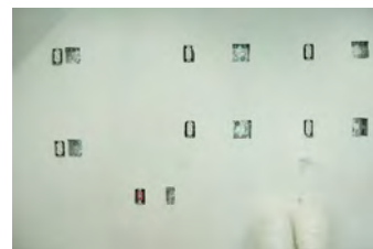
F062207CG-0016 [2018-0227-F_M1Hi_j0072_4.JPG] 6/22/2007 Work continues on the press briefing room
