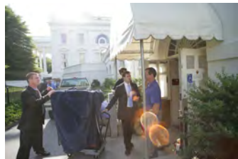
P062207ED-0029 [2018-0227-F_M1Hi_j0015_2.JPG] 6/22/2007 Press Briefing Room rennovations
