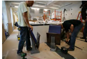
P062107ED-0323 [2018-0227-F_M1Hi_j0018_7.JPG] 6/21/2007 Press Briefing Room Renovations. West Wing.
