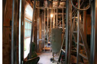
F051607SC-0076 [2018-0227-F_M1Hi_j0237_1.JPG] 5/16/2007 Press Briefing Room Renovations
