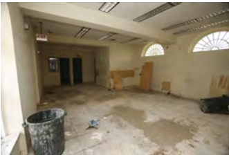
F081506PM-0024 [2018-0227-F_M1Hi_j0180_2.JPG] 8/15/2006 Press Briefing Room Renovations
