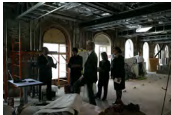
P040207SC-0011 [2018-0227-F_M1Hi_j0221_1.JPG] 4/2/2007 LB. The Brady Press Room During Renovations.
