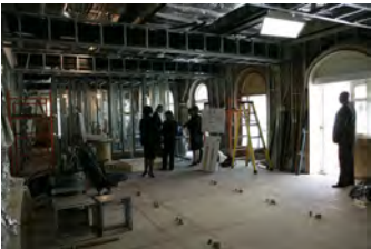
P040207SC-0006 [2018-0227-F_M1Hi_j0196_5.JPG] 4/2/2007 LB. The Brady Press Room During Renovations.
