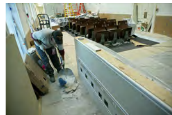
F062207CG-0008 [2018-0227-F_M1Hi_j0056_3.JPG] 6/22/2007 Work continues on the press briefing room
