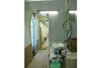
F062207CG-0031 [2018-0227-F_M1Hi_j0102_7.JPG] 6/22/2007 Work continues on the press briefing room
