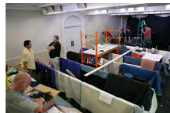
F070507CG-0043 [2018-0227-F_M1Hi_j0187_6.JPG] 7/5/2007 Work nears completion on the press briefing room and the Lower Press office.
