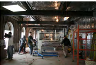
F012507PM-0030 [2018-0227-F_M1Hi_j0073.JPG] 1/25/2007 Press Briefing room renovations.
