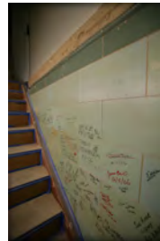
F061207DB-0030 [2018-0227-F_M1Hi_j0204_6.JPG] 6/12/2007 Brady Press Briefing Room Renovations
