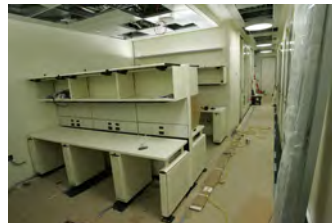
F062007CG-0052 [2018-0227-F_M2Hi_j0019.JPG] 6/20/2007 Work continues on the press briefing room
