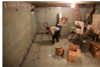
F012507PM-0008 [2018-0227-F_M1Hi_j0029.JPG] 1/25/2007 Press Briefing room renovations.
