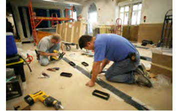
P062107ED-0256 [2018-0227-F_M1Hi_j0139_5.JPG] 6/21/2007 Press Briefing Room Renovations. West Wing.
