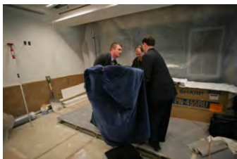
P062207ED-0040 [2018-0227-F_M1Hi_j0196_8.JPG] 6/22/2007 Press Briefing Room rennovations
