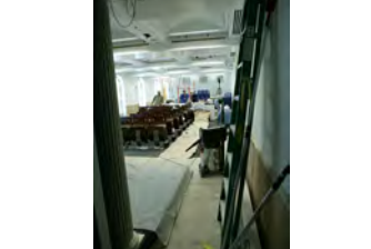
F062207CG-0063 [2018-0227-F_M1Hi_j0166_9.JPG] 6/22/2007 Work continues on the press briefing room
