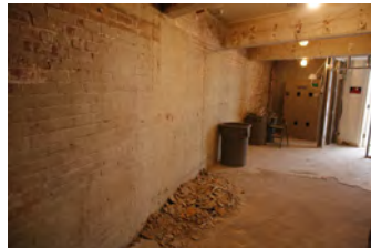
F110106PM-0004 [2018-0227-F_M1Hi_j0101_1.JPG] 11/1/2006 Press Briefing room renovations
