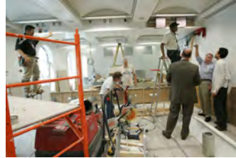
F061507CG-0071 [2018-0227-F_M2Hi_j0042.JPG] 6/15/2007 The Press Briefing Room nears completion
