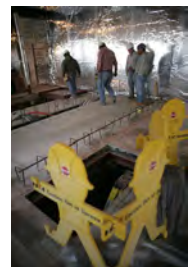
F010907PM-0002 [2018-0227-F_M1Hi_j0118_2.JPG] 1/9/2007 Press Briefing Room Renovations
