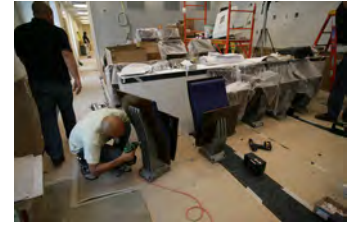
P062107ED-0312 [2018-0227-F_M1Hi_j0251_6.JPG] 6/21/2007 Press Briefing Room Renovations. West Wing.
