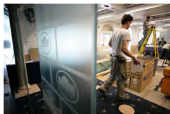
P062107ED-0359 [2018-0227-F_M1Hi_j0090_5.JPG] 6/21/2007 Press Briefing Room Renovations. West Wing.
