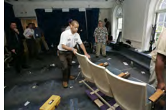
F080306PM-0146 [2018-0227-F_M1Hi_j0114.JPG] 8/3/2006 Clearing out Press Briefing room for renovations.
