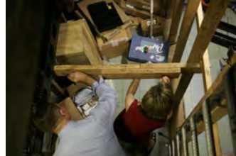
F080306PM-0046 [2018-0227-F_M1Hi_j0169.JPG] 8/3/2006 Clearing out Press Briefing room for renovations.
