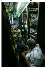
F062807CG-0044 [2018-0227-F_M1Hi_j0165_3.JPG] 6/28/2007 Work continues on the press briefing room
