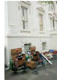
F062907CG-0056 [2018-0227-F_M1Hi_j0203_6.JPG] 6/29/2007 Work nears completion on the press briefing room, Friday June 29, 2007.
