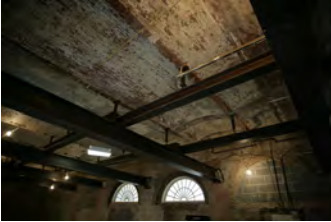
F101906PM-019 [2018-0227-F_M1Hi_j0006_1.JPG] 10/19/2006 Renovations to the Press Briefing room
