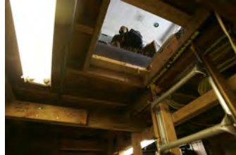
F080306PM-0085 [2018-0227-F_M1Hi_j0247.JPG] 8/3/2006 Clearing out Press Briefing room for renovations.
