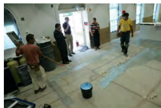
F062007CG-0096 [2018-0227-F_M2Hi_j0107.JPG] 6/20/2007 Work continues on the press briefing room
