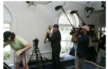
F080306PM-0028 [2018-0227-F_M1Hi_j0133.JPG] 8/3/2006 Clearing out Press Briefing room for renovations.
