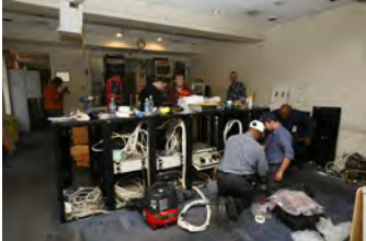
F080406PM-0013 [2018-0227-F_M1Hi_j0162_1.JPG] 8/4/2006 Clearing out Press Briefing room for renovations.
