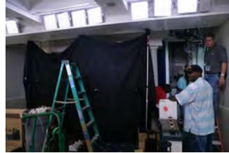
F070507CG-0054 [2018-0227-F_M1Hi_J0209_7.JPG] 7/5/2007 Work nears completion on the press briefing room and the Lower Press office.
