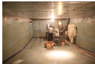
F012507PM-0012 [2018-0227-F_M1Hi_j0037.JPG] 1/25/2007 Press Briefing room renovations.
