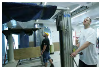
F062007CG-0024 [2018-0227-F_M2Hi_j0218.JPG] 6/20/2007 Work continues on the press briefing room
