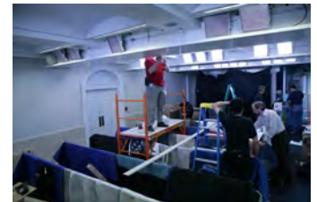
F070507CG-0063 [2018-0227-F_M1Hi_J0227_7.JPG] 7/5/2007 Work nears completion on the press briefing room and the Lower Press office.
