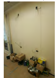
F061507CG-0040 [2018-0227-F_M2Hi_j0235.JPG] 6/15/2007 The Press Briefing Room nears completion
