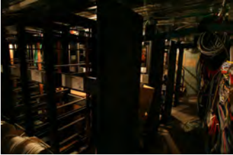
F051607SC-0034 [2018-0227-F_M1Hi_j0149_2.JPG] 5/16/2007 Press Briefing Room Renovations
