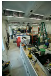
F062907CG-0034 [2018-0227-F_M1Hi_j0038_4.JPG] 6/29/2007 Work nears completion on the press briefing room, Friday June 29, 2007.
