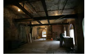
F101906PM-002 [2018-0227-F_M1Hi_j0199_1.JPG] 10/19/2006 Renovations to the Press Briefing room
