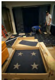
P062107ED-0345 [2018-0227-F_M1Hi_j0062_4.JPG] 6/21/2007 Press Briefing Room Renovations. West Wing.
