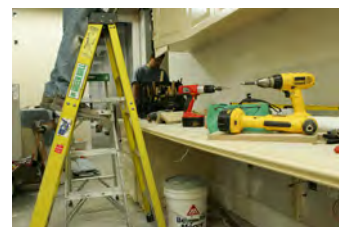
F062807CG-0050 [2018-0227-F_M1Hi_j0177_3.JPG] 6/28/2007 Work continues on the press briefing room
