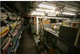
F061207DB-0032 [2018-0227-F_M1Hi_j0216_4.JPG] 6/12/2007 Brady Press Briefing Room Renovations
