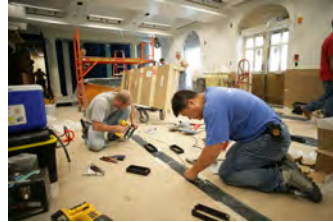
P062107ED-0255 [2018-0227-F_M1Hi_j0137_6.JPG] 6/21/2007 Press Briefing Room Renovations. West Wing.
