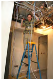
F051607SC-0118 [2018-0227-F_M1Hi_j0066_3.JPG] 5/16/2007 Press Briefing Room Renovations
