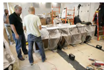
P062107ED-0276 [2018-0227-F_M1Hi_j0179_9.JPG] 6/21/2007 Press Briefing Room Renovations. West Wing.
