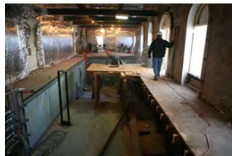
F120206PM-0006 [2018-0227-F_M1Hi_j0154_4.JPG] 12/2/2006 Press Briefing room renovations.
