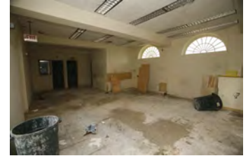
F081506PM-0023 [2018-0227-F_M1Hi_j0178_2.JPG] 8/15/2006 Press Briefing Room Renovations
