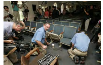
F080306PM-0012 [2018-0227-F_M1Hi_j0101.JPG] 8/3/2006 Clearing out Press Briefing room for renovations.
