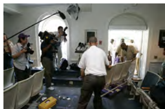
F080306PM-0117 [2018-0227-F_M1Hi_j0056.JPG] 8/3/2006 Clearing out Press Briefing room for renovations.
