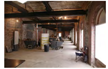
F110106PM-0001 [2018-0227-F_M1Hi_j0095_1.JPG] 11/1/2006 Press Briefing room renovations
