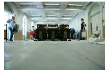
F062207CG-0072 [2018-0227-F_M1Hi_j0184_6.JPG] 6/22/2007 Work continues on the press briefing room
