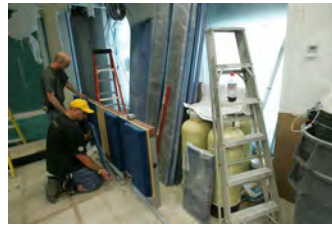
F062007CG-0100 [2018-0227-F_M2Hi_j0115.JPG] 6/20/2007 Work continues on the press briefing room
