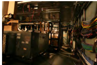
F051607SC-0023 [2018-0227-F_M1Hi_j0106_2.JPG] 5/16/2007 Press Briefing Room Renovations
