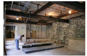
F091806PM-002 [2018-0227-F_M1Hi_j0106_1.JPG] 9/18/2006 Renovations of the Press Briefing Room
