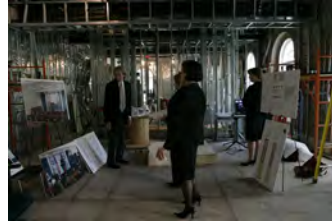
P040207SC-0004 [2018-0227-F_M1Hi_j0188_5.JPG] 4/2/2007 LB. The Brady Press Room During Renovations.
