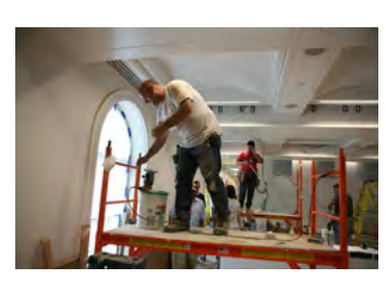
P061907DG-0223 [2018-0227-F_M1Hi_j0205_2.JPG] 6/19/2007 James S. Brady Press Briefing Room renovation
