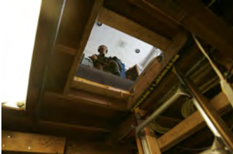
F080306PM-0084 [2018-0227-F_M1Hi_j0245.JPG] 8/3/2006 Clearing out Press Briefing room for renovations.
