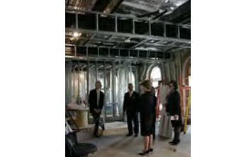
P040207SC-0045 [2018-0227-F_M1Hi_j0190_5.JPG] 4/2/2007 LB. The Brady Press Room During Renovations.
