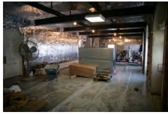
F010907PM-0004 [2018-0227-F_M1Hi_j0122_2.JPG] 1/9/2007 Press Briefing Room Renovations
