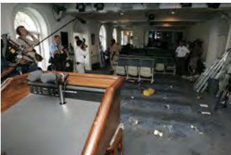
F080306PM-0152 [2018-0227-F_M1Hi_j0126.JPG] 8/3/2006 Clearing out Press Briefing room for renovations.
