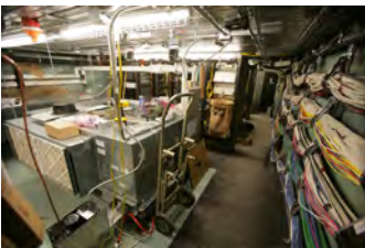
F061207DB-0036 [2018-0227-F_M1Hi_j0247_2.JPG] 6/12/2007 Brady Press Briefing Room Renovations
