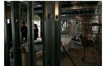
P040207SC-0009 [2018-0227-F_M1Hi_j0213_1.JPG] 4/2/2007 LB. The Brady Press Room During Renovations.
