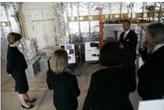
P040207SC-0050 [2018-0227-F_M1Hi_j0220_3.JPG] 4/2/2007 LB. The Brady Press Room During Renovations.
