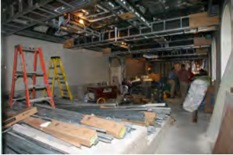
F051607SC-0154 [2018-0227-F_M1Hi_j0138_5.JPG] 5/16/2007 Press Briefing Room Renovations
