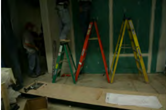
F062007CG-0002 [2018-0227-F_M2Hi_j0174.JPG] 6/20/2007 Work continues on the press briefing room
