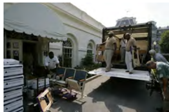
F080306PM-0137 [2018-0227-F_M1Hi_j0096.JPG] 8/3/2006 Clearing out Press Briefing room for renovations.
