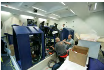
F062907CG-0061 [2018-0227-F_M1Hi_j0213_5.JPG] 6/29/2007 Work nears completion on the press briefing room, Friday June 29, 2007.
