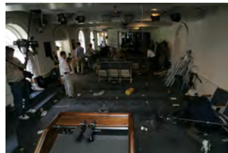
F080306PM-0154 [2018-0227-F_M1Hi_j0130.JPG] 8/3/2006 Clearing out Press Briefing room for renovations.
