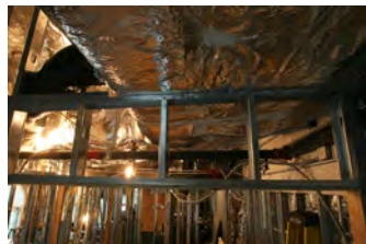
F051607SC-0068 [2018-0227-F_M1Hi_j0221_2.JPG] 5/16/2007 Press Briefing Room Renovations
