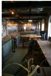
F120206PM-0018 [2018-0227-F_M1Hi_j0178_4.JPG] 12/2/2006 Press Briefing room renovations.
