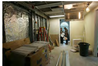
F061507CG-0016 [2018-0227-F_M2Hi_j0187.JPG] 6/15/2007 The Press Briefing Room nears completion
