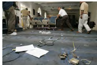
F080306PM-0178 [2018-0227-F_M1Hi_j0178.JPG] 8/3/2006 Clearing out Press Briefing room for renovations.
