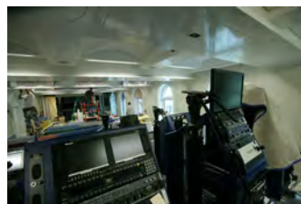
F062907CG-0027 [2018-0227-F_M1Hi_j0024_4.JPG] 6/29/2007 Work nears completion on the press briefing room, Friday June 29, 2007.
