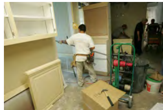
F061907CG-0007 [2018-0227-F_M2Hi_j0191_1.JPG] 6/19/2007 Work continues on the Brady Briefing Room
