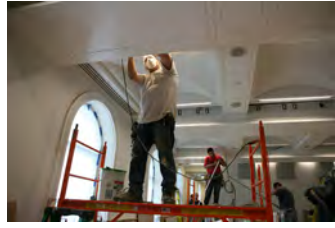
P061907DG-0229 [2018-0227-F_M1Hi_j0217_3.JPG] 6/19/2007 James S. Brady Press Briefing Room renovation
