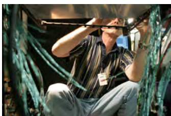
F062807CG-0040 [2018-0227-F_M1Hi_j0157_3.JPG] 6/28/2007 Work continues on the press briefing room
