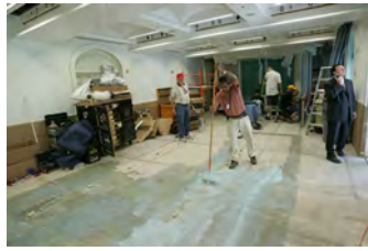
F062007CG-0099 [2018-0227-F_M2Hi_j0113.JPG] 6/20/2007 Work continues on the press briefing room
