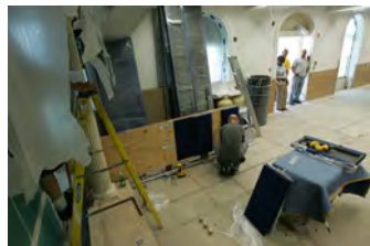
F062007CG-0075 [2018-0227-F_M2Hi_j0065.JPG] 6/20/2007 Work continues on the press briefing room
