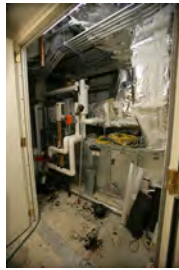
F061207DB-0045 [2018-0227-F_M1Hi_j0046_3.JPG] 6/12/2007 Brady Press Briefing Room Renovations
