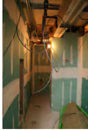
F051607SC-0114 [2018-0227-F_M1Hi_j0058_2.JPG] 5/16/2007 Press Briefing Room Renovations
