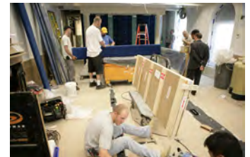
P062107ED-0204 [2018-0227-F_M1Hi_j0035_2.JPG] 6/21/2007 Press Briefing Room Renovations. West Wing.
