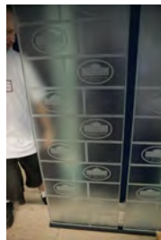
P062107ED-0302 [2018-0227-F_M1Hi_j0231_7.JPG] 6/21/2007 Press Briefing Room Renovations. West Wing.
