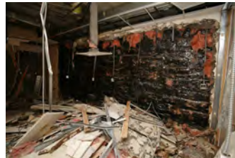
F081506PM-0026 [2018-0227-F_M1Hi_j0184_2.JPG] 8/15/2006 Press Briefing Room Renovations
