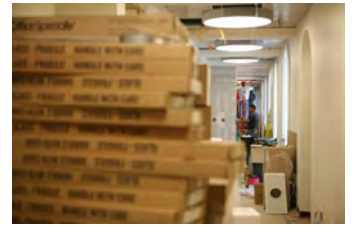
P061907DG-0251 [2018-0227-F_M1Hi_j0006_3.JPG] 6/19/2007 James S. Brady Press Briefing Room renovation
