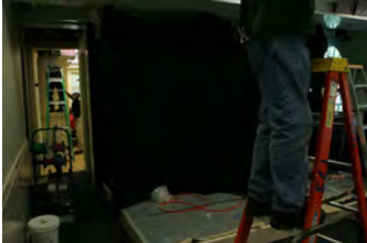
F070207CG-0012 [2018-0227-F_M1Hi_j0091_1.JPG] 7/2/2007 Work nears completion on the press briefing room
