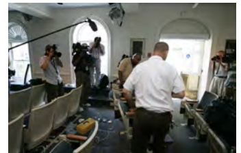
F080306PM-0115 [2018-0227-F_M1Hi_j0052.JPG] 8/3/2006 Clearing out Press Briefing room for renovations.
