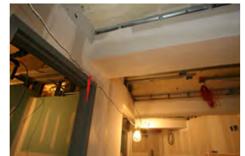
F051607SC-0109 [2018-0227-F_M1Hi_j0048_2.JPG] 5/16/2007 Press Briefing Room Renovations
