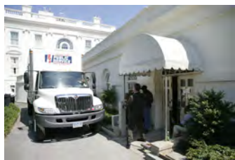
P062107ED-0330 [2018-0227-F_M1Hi_j0032_6.JPG] 6/21/2007 Press Briefing Room Renovations. West Wing.
