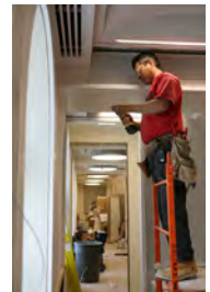
P061907DG-0247 [2018-0227-F_M1Hi_j0253_4.JPG] 6/19/2007 James S. Brady Press Briefing Room renovation
