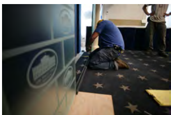
P062107ED-0353 [2018-0227-F_M1Hi_j0078_5.JPG] 6/21/2007 Press Briefing Room Renovations. West Wing.
