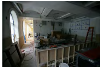
F061207DB-0054 [2018-0227-F_M1Hi_j0100_3.JPG] 6/12/2007 Brady Press Briefing Room Renovations
