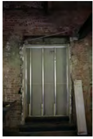
F101806KH-0031 [2018-0227-F_M1Hi_j0206_2.JPG] 10/18/2006 Press Room Renovations
