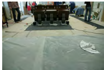
F062207CG-0071 [2018-0227-F_M1Hi_j0182_5.JPG] 6/22/2007 Work continues on the press briefing room
