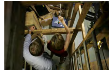
F080306PM-0043 [2018-0227-F_M1Hi_j0163.JPG] 8/3/2006 Clearing out Press Briefing room for renovations.
