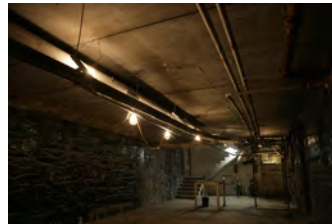
F101806KH-0021 [2018-0227-F_M1Hi_j0186_3.JPG] 10/18/2006 Press Room Renovations
