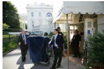
P062207ED-0030 [2018-0227-F_M1Hi_j0013_4.JPG] 6/22/2007 Press Briefing Room rennovations
