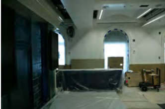
F062207CG-0077 [2018-0227-F_M1Hi_j0194_5.JPG] 6/22/2007 Work continues on the press briefing room
