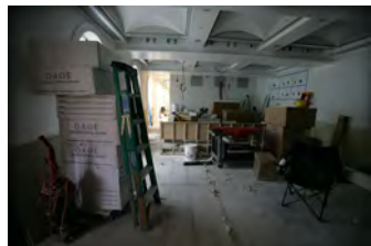
F061207DB-0057 [2018-0227-F_M1Hi_j0118_4.JPG] 6/12/2007 Brady Press Briefing Room Renovations
