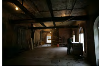
F101906PM-001 [2018-0227-F_M1Hi_j0195_1.JPG] 10/19/2006 Renovations to the Press Briefing room
