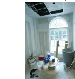
F061507CG-0020 [2018-0227-F_M2Hi_j0195.JPG] 6/15/2007 The Press Briefing Room nears completion
