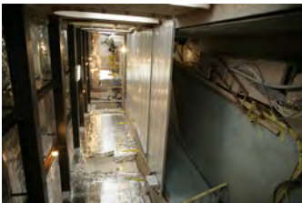
F121506PM-0002 [2018-0227-F_M1Hi_j0107_1.JPG] 12/15/2006 Press Briefing room renovations
