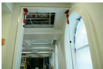
F062207CG-0019 [2018-0227-F_M1Hi_j0078_6.JPG] 6/22/2007 Work continues on the press briefing room
