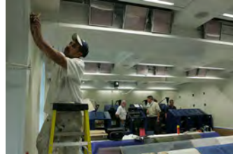
F062807CG-0061 [2018-0227-F_M1Hi_j0199_5.JPG] 6/28/2007 Work continues on the press briefing room
