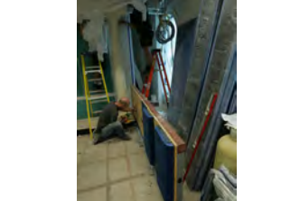
F062007CG-0076 [2018-0227-F_M2Hi_j0067.JPG] 6/20/2007 Work continues on the press briefing room
