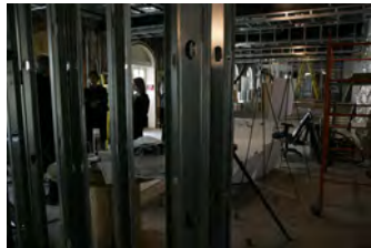
P040207SC-0007 [2018-0227-F_M1Hi_j0200_5.JPG] 4/2/2007 LB. The Brady Press Room During Renovations.
