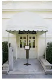
F101806KH-0033 [2018-0227-F_M1Hi_j0210_2.JPG] 10/18/2006 Press Room Renovations
