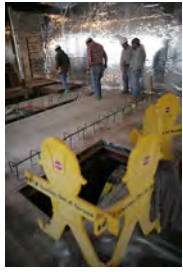
F010907PM-0003 [2018-0227-F_M1Hi_j0120_1.JPG] 1/9/2007 Press Briefing Room Renovations
