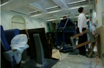
F062207CG-0037 [2018-0227-F_M1Hi_j0114_5.JPG] 6/22/2007 Work continues on the press briefing room
