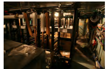
F051607SC-0029 [2018-0227-F_M1Hi_j0132_3.JPG] 5/16/2007 Press Briefing Room Renovations
