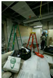
F062707CG-0049 [2018-0227-F_M1Hi_j0053_1.JPG] 6/27/2007 Work continues on the press briefing room
