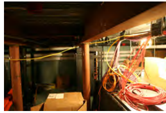
F051607SC-0012 [2018-0227-F_M1Hi_j0050_1.JPG] 5/16/2007 Press Briefing Room Renovations
