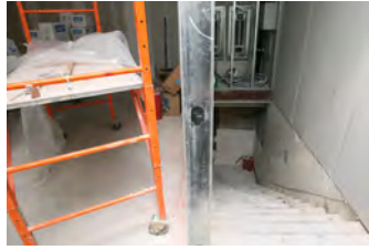
F051607SC-0151 [2018-0227-F_M1Hi_j0132_4.JPG] 5/16/2007 Press Briefing Room Renovations
