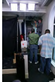
F070507CG-0053 [2018-0227-F_M1Hi_J0207_9.JPG] 7/5/2007 Work nears completion on the press briefing room and the Lower Press office.
