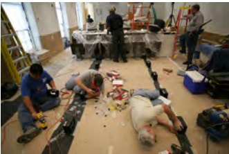
P062107ED-0297 [2018-0227-F_M1Hi_j0221_6.JPG] 6/21/2007 Press Briefing Room Renovations. West Wing.
