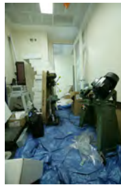
F062707CG-0035 [2018-0227-F_M1Hi_j0239_4.JPG] 6/27/2007 Work continues on the press briefing room
