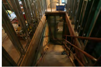
F051607SC-0055 [2018-0227-F_M1Hi_j0195_2.JPG] 5/16/2007 Press Briefing Room Renovations
