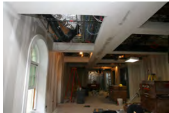
F051607SC-0099 [2018-0227-F_M1Hi_j0028_2.JPG] 5/16/2007 Press Briefing Room Renovations
