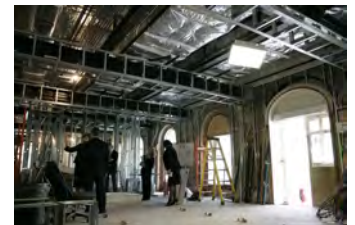
P040207SC-0037 [2018-0227-F_M1Hi_j0114_2.JPG] 4/2/2007 LB. The Brady Press Room During Renovations.
