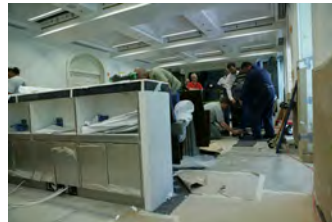
F062207CG-0043 [2018-0227-F_M1Hi_j0126_6.JPG] 6/22/2007 Work continues on the press briefing room
