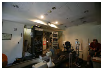
F080406PM-0043 [2018-0227-F_M1Hi_j0222.JPG] 8/4/2006 Clearing out Press Briefing room for renovations.
