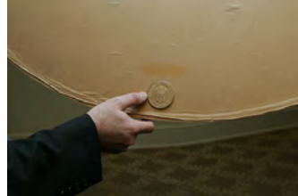
F080306PM-0066 [2018-0227-F_M1Hi_j0209.JPG] 8/3/2006 Clearing out Press Briefing room for renovations.
