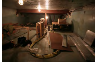
F012507PM-0020 [2018-0227-F_M1Hi_j0053.JPG] 1/25/2007 Press Briefing room renovations.
