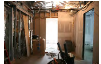
F053107LS-0011 [2018-0227-F_M1Hi_j0078_3.JPG] 5/31/2007 renovation progress of James S. Brady Press Briefing Room
