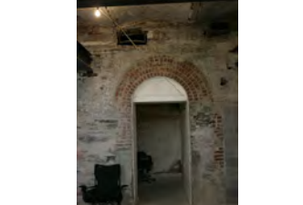
F101806KH-0005 [2018-0227-F_M1Hi_j0154_3.JPG] 10/18/2006 Press Room Renovations
