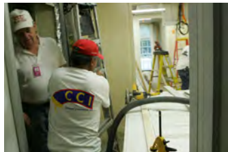
F062907CG-0042 [2018-0227-F_M1Hi_j0175_6.JPG] 6/29/2007 Work nears completion on the press briefing room, Friday June 29, 2007.
