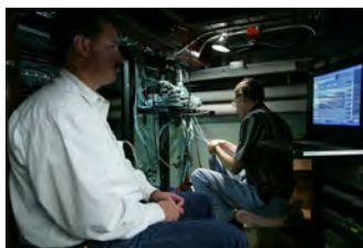
F062807CG-0045 [2018-0227-F_M1Hi_j0167_6.JPG] 6/28/2007 Work continues on the press briefing room
