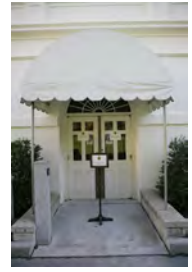
F101806KH-0034 [2018-0227-F_M1Hi_j0212_2.JPG] 10/18/2006 Press Room Renovations
