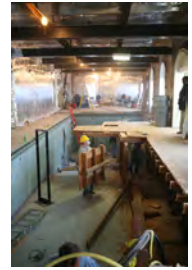
F120206PM-0012 [2018-0227-F_M1Hi_j0166_4.JPG] 12/2/2006 Press Briefing room renovations.
