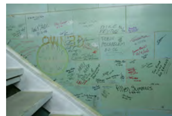
F062007CG-0021 [2018-0227-F_M2Hi_j0212.JPG] 6/20/2007 Work continues on the press briefing room
