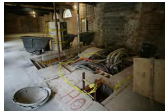
F101906PM-013 [2018-0227-F_M1Hi_j0249_1.JPG] 10/19/2006 Renovations to the Press Briefing room
