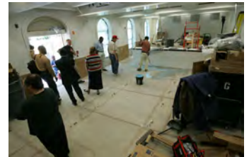
F062007CG-0089 [2018-0227-F_M2Hi_j0093.JPG] 6/20/2007 Work continues on the press briefing room
