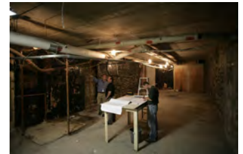
F101906PM-026 [2018-0227-F_M1Hi_j0020_1.JPG] 10/19/2006 Renovations to the Press Briefing room
