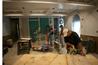
P061907DG-0214 [2018-0227-F_M1Hi_j0187_2.JPG] 6/19/2007 James S. Brady Press Briefing Room renovation
