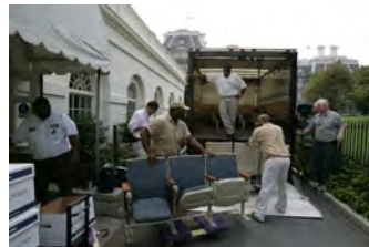
F080306PM-0134 [2018-0227-F_M1Hi_j0090.JPG] 8/3/2006 Clearing out Press Briefing room for renovations.
