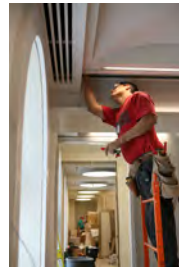
P061907DG-0242 [2018-0227-F_M1Hi_j0243_2.JPG] 6/19/2007 James S. Brady Press Briefing Room renovation
