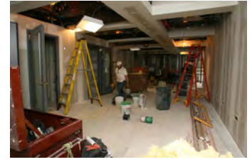
F051607SC-0093 [2018-0227-F_M1Hi_j0016_2.JPG] 5/16/2007 Press Briefing Room Renovations
