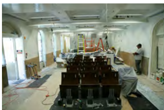
F062207CG-0014 [2018-0227-F_M1Hi_j0068_4.JPG] 6/22/2007 Work continues on the press briefing room
