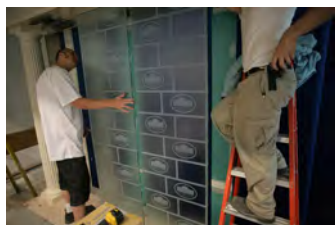
P062107ED-0286 [2018-0227-F_M1Hi_j0199_9.JPG] 6/21/2007 Press Briefing Room Renovations. West Wing.
