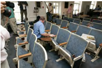
F080306PM-0052 [2018-0227-F_M1Hi_j0181.JPG] 8/3/2006 Clearing out Press Briefing room for renovations.
