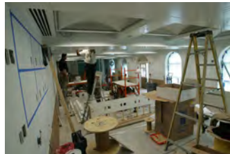
F061507CG-0055 [2018-0227-F_M2Hi_j0010.JPG] 6/15/2007 The Press Briefing Room nears completion
