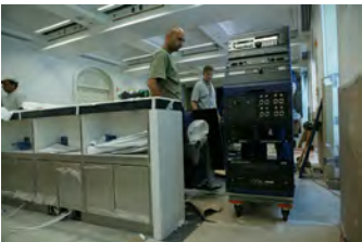
F062207CG-0045 [2018-0227-F_M1Hi_j0130_5.JPG] 6/22/2007 Work continues on the press briefing room
