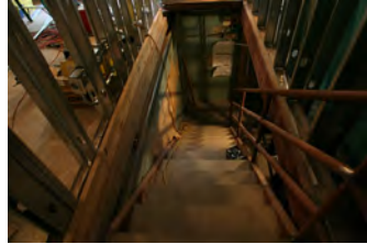
F051607SC-0056 [2018-0227-F_M1Hi_j0197_1.JPG] 5/16/2007 Press Briefing Room Renovations
