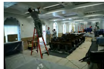
F062207CG-0060 [2018-0227-F_M1Hi_j0160_8.JPG] 6/22/2007 Work continues on the press briefing room
