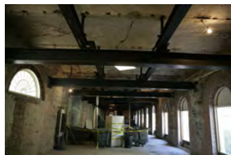
F101806KH-0004 [2018-0227-F_M1Hi_j0152_3.JPG] 10/18/2006 Press Room Renovations
