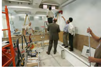
F061507CG-0070 [2018-0227-F_M2Hi_j0040.JPG] 6/15/2007 The Press Briefing Room nears completion
