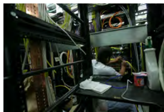
F062007CG-0020 [2018-0227-F_M2Hi_j0210.JPG] 6/20/2007 Work continues on the press briefing room
