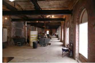
F110106PM-0003 [2018-0227-F_M1Hi_j0019.JPG] 11/1/2006 Press Briefing room renovations
