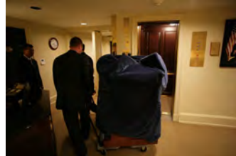
P062207ED-0002 [2018-0227-F_M1Hi_j0108_5.JPG] 6/22/2007 Press Briefing Room rennovations
