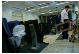
F062207CG-0035 [2018-0227-F_M1Hi_j0110_4.JPG] 6/22/2007 Work continues on the press briefing room
