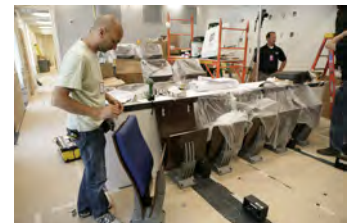
P062107ED-0308 [2018-0227-F_M1Hi_j0243_6.JPG] 6/21/2007 Press Briefing Room Renovations. West Wing.
