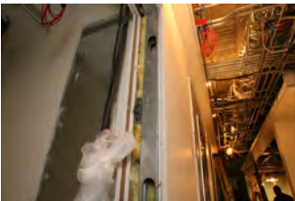
F051607SC-0122 [2018-0227-F_M1Hi_j0074_1.JPG] 5/16/2007 Press Briefing Room Renovations
