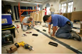
P062107ED-0254 [2018-0227-F_M1Hi_j0135_5.JPG] 6/21/2007 Press Briefing Room Renovations. West Wing.
