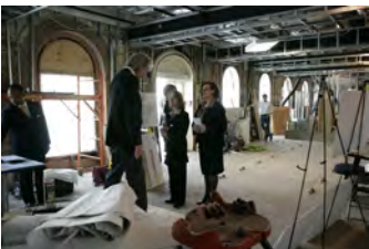
P040207SC-0014 [2018-0227-F_M1Hi_j0233_1.JPG] 4/2/2007 LB. The Brady Press Room During Renovations.
