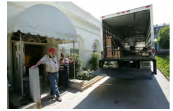
F062007CG-0101 [2018-0227-F_M2Hi_j0117.JPG] 6/20/2007 Work continues on the press briefing room
