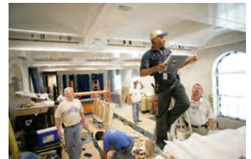
P062107ED-0244 [2018-0227-F_M1Hi_j0115_7.JPG] 6/21/2007 Press Briefing Room Renovations. West Wing.
