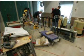
F061907CG-0001 [2018-0227-F_M2Hi_j0179_1.JPG] 6/19/2007 Work continues on the Brady Briefing Room
