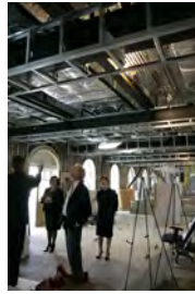
P040207SC-0019 [2018-0227-F_M1Hi_j0007.JPG] 4/2/2007 LB. The Brady Press Room During Renovations.
