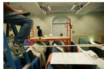
F070507CG-0047 [2018-0227-F_M1Hi_j0195_8.JPG] 7/5/2007 Work nears completion on the press briefing room and the Lower Press office.
