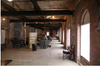
F110106PM-0002 [2018-0227-F_M1Hi_j0017.JPG] 11/1/2006 Press Briefing room renovations
