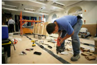
P062107ED-0250 [2018-0227-F_M1Hi_j0127_5.JPG] 6/21/2007 Press Briefing Room Renovations. West Wing.
