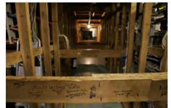
F080306PM-0071 [2018-0227-F_M1Hi_j0219.JPG] 8/3/2006 Clearing out Press Briefing room for renovations.
