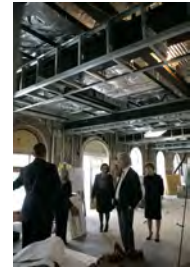
P040207SC-0021 [2018-0227-F_M1Hi_j0018_2.JPG] 4/2/2007 LB. The Brady Press Room During Renovations.
