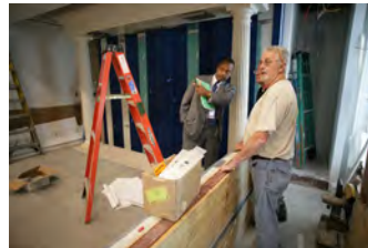
P062107ED-0219 [2018-0227-F_M1Hi_j0065_5.JPG] 6/21/2007 Press Briefing Room Renovations. West Wing.
