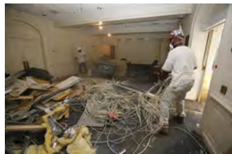
F081506PM-0012 [2018-0227-F_M1Hi_j0156_2.JPG] 8/15/2006 Press Briefing Room Renovations
