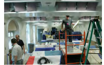
F062907CG-0036 [2018-0227-F_M1Hi_j0042_3.JPG] 6/29/2007 Work nears completion on the press briefing room, Friday June 29, 2007.
