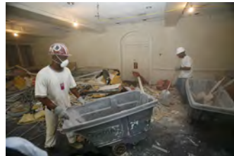
F081506PM-0005 [2018-0227-F_M1Hi_j0142_2.JPG] 8/15/2006 Press Briefing Room Renovations
