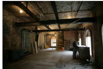
F101906PM-005 [2018-0227-F_M1Hi_j0211_1.JPG] 10/19/2006 Renovations to the Press Briefing room
