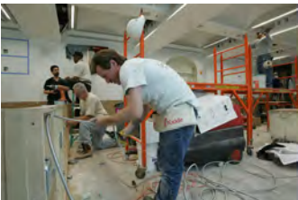
F061507CG-0014 [2018-0227-F_M2Hi_j0183.JPG] 6/15/2007 The Press Briefing Room nears completion
