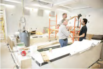
P062107ED-0213 [2018-0227-F_M1Hi_j0053_5.JPG] 6/21/2007 Press Briefing Room Renovations. West Wing.
