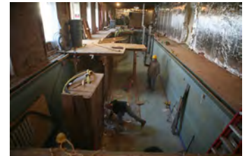
F120206PM-0020 [2018-0227-F_M1Hi_j0182_4.JPG] 12/2/2006 Press Briefing room renovations.
