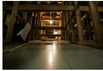
F080306PM-0082 [2018-0227-F_M1Hi_j0241.JPG] 8/3/2006 Clearing out Press Briefing room for renovations.
