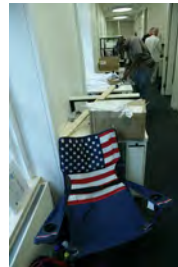
F070507CG-0062 [2018-0227-F_M1Hi_J0225_5.JPG] 7/5/2007 Work nears completion on the press briefing room and the Lower Press office.
