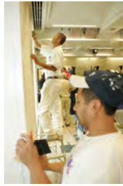
F062807CG-0016 [2018-0227-F_M1Hi_j0109_4.JPG] 6/28/2007 Work continues on the press briefing room
