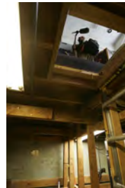
F080306PM-0086 [2018-0227-F_M1Hi_j0249.JPG] 8/3/2006 Clearing out Press Briefing room for renovations.
