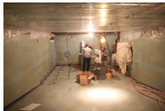
F012507PM-0011 [2018-0227-F_M1Hi_j0035.JPG] 1/25/2007 Press Briefing room renovations.
