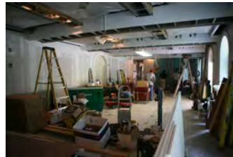
F053107LS-0006 [2018-0227-F_M1Hi_j0068_2.JPG] 5/31/2007 renovation progress of James S. Brady Press Briefing Room
