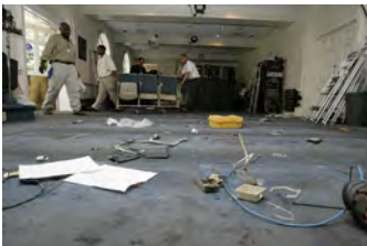
F080306PM-0172 [2018-0227-F_M1Hi_j0166.JPG] 8/3/2006 Clearing out Press Briefing room for renovations.
