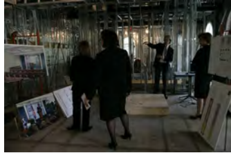
P040207SC-0003 [2018-0227-F_M1Hi_j0184_5.JPG] 4/2/2007 LB. The Brady Press Room During Renovations.
