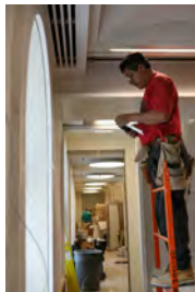
P061907DG-0244 [2018-0227-F_M1Hi_j0247_3.JPG] 6/19/2007 James S. Brady Press Briefing Room renovation
