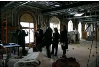
P040207SC-0010 [2018-0227-F_M1Hi_j0217_1.JPG] 4/2/2007 LB. The Brady Press Room During Renovations.
