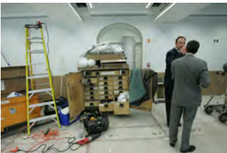
F062007CG-0050 [2018-0227-F_M2Hi_j0015.JPG] 6/20/2007 Work continues on the press briefing room
