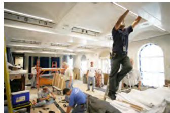
P062107ED-0242 [2018-0227-F_M1Hi_j0111_7.JPG] 6/21/2007 Press Briefing Room Renovations. West Wing.
