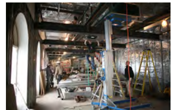
F012507PM-0033 [2018-0227-F_M1Hi_j0079_1.JPG] 1/25/2007 Press Briefing room renovations.
