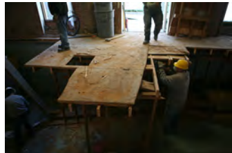
F120206PM-0038 [2018-0227-F_M1Hi_j0218_2.JPG] 12/2/2006 Press Briefing room renovations.
