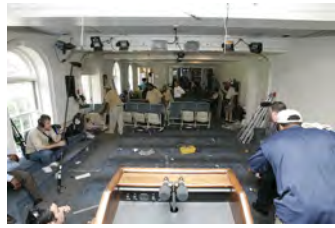
F080306PM-0161 [2018-0227-F_M1Hi_j0144.JPG] 8/3/2006 Clearing out Press Briefing room for renovations.
