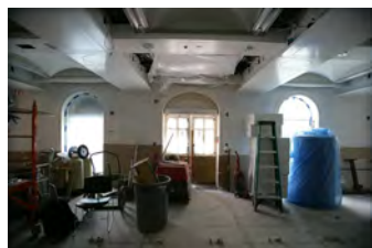
F061207DB-0018 [2018-0227-F_M1Hi_j0125_2.JPG] 6/12/2007 Brady Press Briefing Room Renovations
