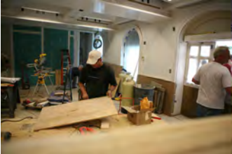
P061907DG-0212 [2018-0227-F_M1Hi_j0183_2.JPG] 6/19/2007 James S. Brady Press Briefing Room renovation
