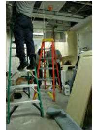
F062707CG-0040 [2018-0227-F_M1Hi_j0017_4.JPG] 6/27/2007 Work continues on the press briefing room
