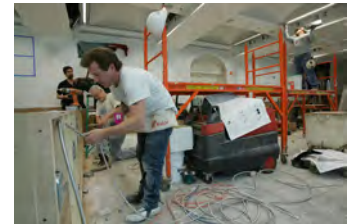
F061507CG-0013 [2018-0227-F_M2Hi_j0181.JPG] 6/15/2007 The Press Briefing Room nears completion
