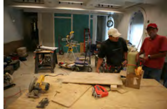
P061907DG-0213 [2018-0227-F_M1Hi_j0185_2.JPG] 6/19/2007 James S. Brady Press Briefing Room renovation
