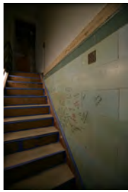
F061207DB-0040 [2018-0227-F_M1Hi_j0016_3.JPG] 6/12/2007 Brady Press Briefing Room Renovations
