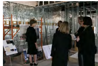
P040207SC-0052 [2018-0227-F_M1Hi_j0232_2.JPG] 4/2/2007 LB. The Brady Press Room During Renovations.
