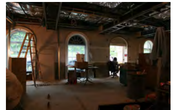
F051607SC-0085 [2018-0227-F_M1Hi_j0255_2.JPG] 5/16/2007 Press Briefing Room Renovations
