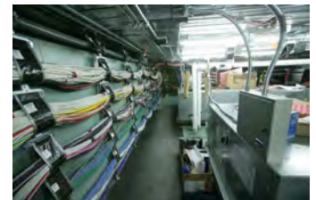
F062007CG-0009 [2018-0227-F_M2Hi_j0188.JPG] 6/20/2007 Work continues on the press briefing room
