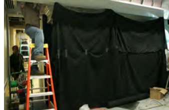
F070207CG-0014 [2018-0227-F_M1Hi_j0099_2.JPG] 7/2/2007 Work nears completion on the press briefing room
