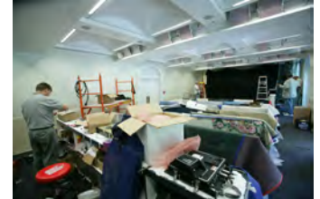
F070207CG-0023 [2018-0227-F_M1Hi_j0079_2.JPG] 7/2/2007 Work nears completion on the press briefing room
