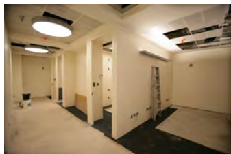
F061207DB-0005 [2018-0227-F_M1Hi_j0038_3.JPG] 6/12/2007 Brady Press Briefing Room Renovations
