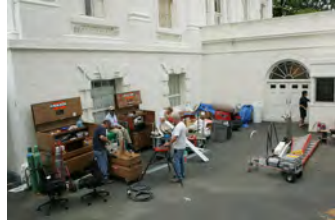
F062907CG-0054 [2018-0227-F_M1Hi_j0199_6.JPG] 6/29/2007 Work nears completion on the press briefing room, Friday June 29, 2007.
