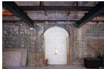
F091806PM-004 [2018-0227-F_M1Hi_j0114_1.JPG] 9/18/2006 Renovations of the Press Briefing Room
