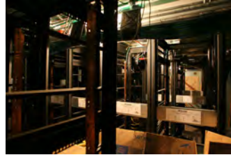
F051607SC-0036 [2018-0227-F_M1Hi_j0153_2.JPG] 5/16/2007 Press Briefing Room Renovations
