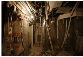
F081506PM-0037 [2018-0227-F_M1Hi_j0206_1.JPG] 8/15/2006 Press Briefing Room Renovations
