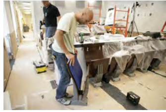
P062107ED-0310 [2018-0227-F_M1Hi_j0247_8.JPG] 6/21/2007 Press Briefing Room Renovations. West Wing.
