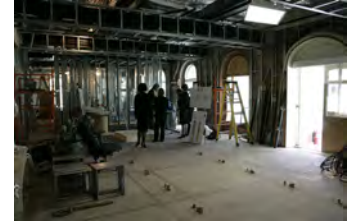
P040207SC-0005 [2018-0227-F_M1Hi_j0192_5.JPG] 4/2/2007 LB. The Brady Press Room During Renovations.
