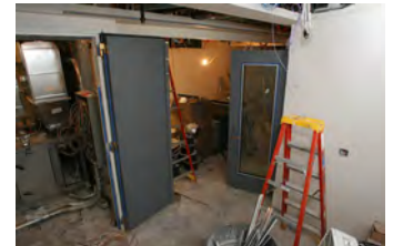
F051607SC-0141 [2018-0227-F_M1Hi_j0112_2.JPG] 5/16/2007 Press Briefing Room Renovations
