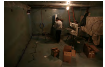
F012507PM-0005 [2018-0227-F_M1Hi_j0023_1.JPG] 1/25/2007 Press Briefing room renovations.
