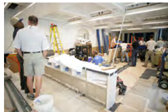
P062107ED-0207 [2018-0227-F_M1Hi_j0041_3.JPG] 6/21/2007 Press Briefing Room Renovations. West Wing.
