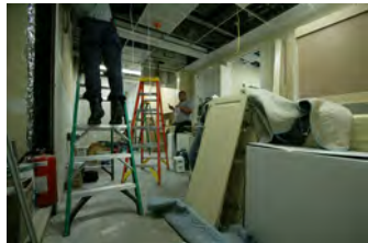
F062707CG-0042 [2018-0227-F_M1Hi_j0025_3.JPG] 6/27/2007 Work continues on the press briefing room
