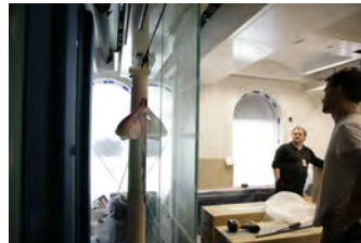
P062107ED-0259 [2018-0227-F_M1Hi_j0145_5.JPG] 6/21/2007 Press Briefing Room Renovations. West Wing.
