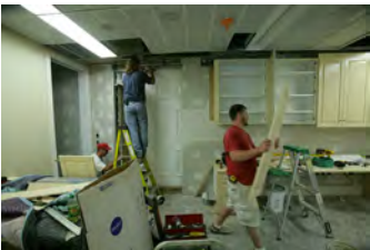
F062807CG-0027 [2018-0227-F_M1Hi_j0131_5.JPG] 6/28/2007 Work continues on the press briefing room
