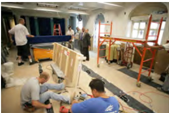
P062107ED-0201 [2018-0227-F_M1Hi_j0029_1.JPG] 6/21/2007 Press Briefing Room Renovations. West Wing.
