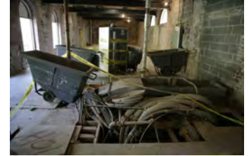
F101806KH-0018 [2018-0227-F_M1Hi_j0180_3.JPG] 10/18/2006 Press Room Renovations
