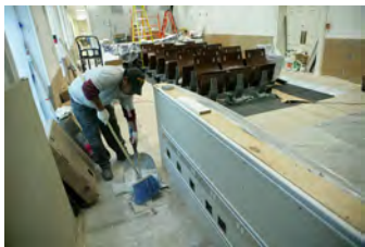
F062207CG-0009 [2018-0227-F_M1Hi_j0058_6.JPG] 6/22/2007 Work continues on the press briefing room
