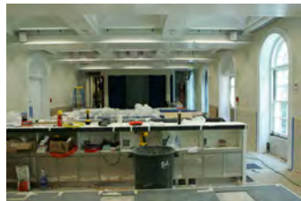
F062707CG-0018 [2018-0227-F_M1Hi_j0171_3.JPG] 6/27/2007 Work continues on the press briefing room
