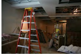
F053107LS-0001 [2018-0227-F_M1Hi_j0058_3.JPG] 5/31/2007 renovation progress of James S. Brady Press Briefing Room
