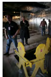
F010907PM-0001 [2018-0227-F_M1Hi_j0116_1.JPG] 1/9/2007 Press Briefing Room Renovations
