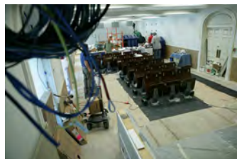
F062207CG-0067 [2018-0227-F_M1Hi_j0174_7.JPG] 6/22/2007 Work continues on the press briefing room
