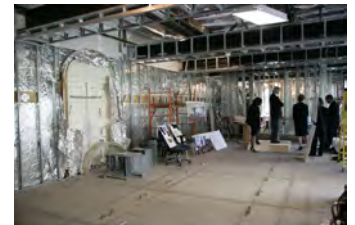
P040207SC-0033 [2018-0227-F_M1Hi_j0090_1.JPG] 4/2/2007 LB. The Brady Press Room During Renovations.
