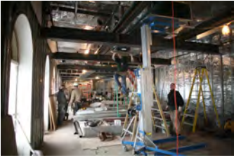
F012507PM-0034 [2018-0227-F_M1Hi_j0081_1.JPG] 1/25/2007 Press Briefing room renovations.
