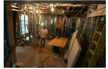
F051607SC-0073 [2018-0227-F_M1Hi_j0231_1.JPG] 5/16/2007 Press Briefing Room Renovations
