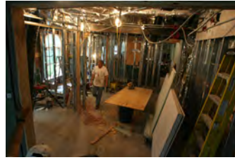
F051607SC-0072 [2018-0227-F_M1Hi_j0229_2.JPG] 5/16/2007 Press Briefing Room Renovations
