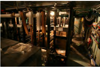
F051607SC-0030 [2018-0227-F_M1Hi_j0136_3.JPG] 5/16/2007 Press Briefing Room Renovations
