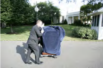
P062207ED-0020 [2018-0227-F_M1Hi_j0156_8.JPG] 6/22/2007 Press Briefing Room rennovations
