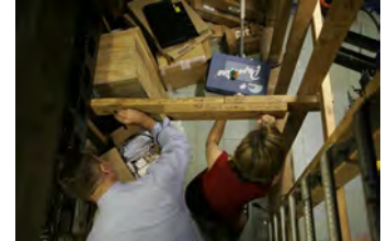
F080306PM-0047 [2018-0227-F_M1Hi_j0171.JPG] 8/3/2006 Clearing out Press Briefing room for renovations.
