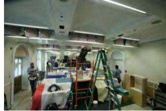
F062907CG-0035 [2018-0227-F_M1Hi_j0040_6.JPG] 6/29/2007 Work nears completion on the press briefing room, Friday June 29, 2007.
