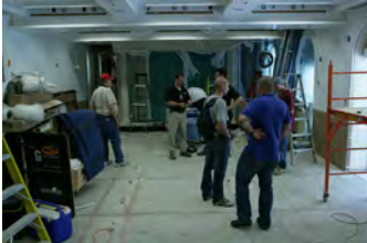
F062007CG-0062 [2018-0227-F_M2Hi_j0039.JPG] 6/20/2007 Work continues on the press briefing room
