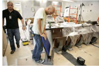
P062107ED-0311 [2018-0227-F_M1Hi_j0249_6.JPG] 6/21/2007 Press Briefing Room Renovations. West Wing.
