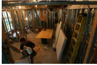
F051607SC-0071 [2018-0227-F_M1Hi_j0227_1.JPG] 5/16/2007 Press Briefing Room Renovations
