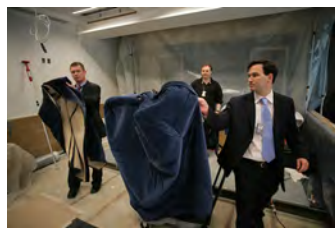
P062207ED-0038 [2018-0227-F_M1Hi_j0005_2.JPG] 6/22/2007 Press Briefing Room rennovations
