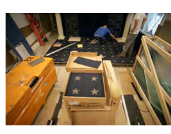
P062107ED-0348 [2018-0227-F_M1Hi_j0068_3.JPG] 6/21/2007 Press Briefing Room Renovations. West Wing.
