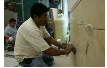
F061507CG-0005 [2018-0227-F_M2Hi_j0165.JPG] 6/15/2007 The Press Briefing Room nears completion
