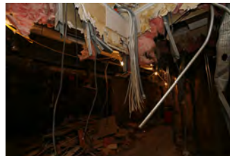
F081506PM-0030 [2018-0227-F_M1Hi_j0192_2.JPG] 8/15/2006 Press Briefing Room Renovations
