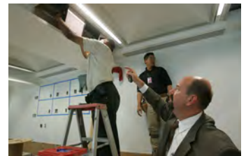
F061507CG-0064 [2018-0227-F_M2Hi_j0028.JPG] 6/15/2007 The Press Briefing Room nears completion
