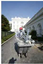
F081506PM-0056 [2018-0227-F_M1Hi_j0244_1.JPG] 8/15/2006 Press Briefing Room Renovations
