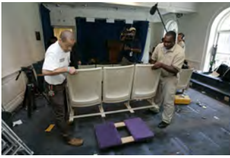
F080306PM-0120 [2018-0227-F_M1Hi_j0062.JPG] 8/3/2006 Clearing out Press Briefing room for renovations.
