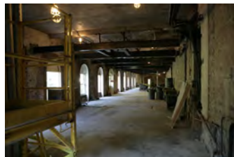
F101806KH-0028 [2018-0227-F_M1Hi_j0200_3.JPG] 10/18/2006 Press Room Renovations
