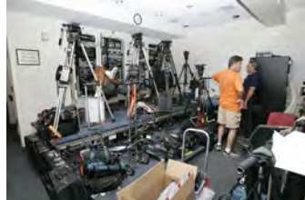
F080306PM-0006 [2018-0227-F_M1Hi_j0089.JPG] 8/3/2006 Clearing out Press Briefing room for renovations.
