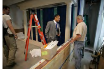
P062107ED-0215 [2018-0227-F_M1Hi_j0057_5.JPG] 6/21/2007 Press Briefing Room Renovations. West Wing.
