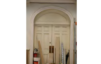
P061907DG-0219 [2018-0227-F_M1Hi_j0197_2.JPG] 6/19/2007 James S. Brady Press Briefing Room renovation
