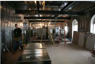
F012507PM-0002 [2018-0227-F_M1Hi_j0017_1.JPG] 1/25/2007 Press Briefing room renovations.
