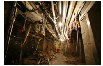
F081506PM-0039 [2018-0227-F_M1Hi_j0210_1.JPG] 8/15/2006 Press Briefing Room Renovations
