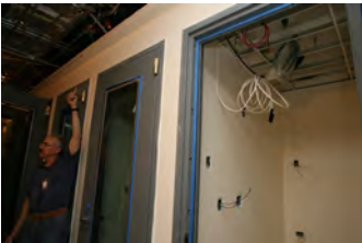
F051607SC-0138 [2018-0227-F_M1Hi_j0106_3.JPG] 5/16/2007 Press Briefing Room Renovations
