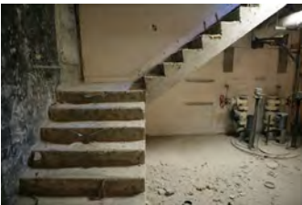
F101806KH-0023 [2018-0227-F_M1Hi_j0190_3.JPG] 10/18/2006 Press Room Renovations
