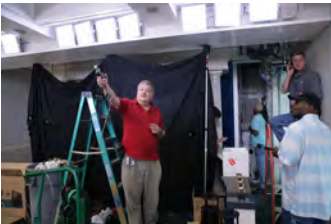
F070507CG-0056 [2018-0227-F_M1Hi_J0213_7.JPG] 7/5/2007 Work nears completion on the press briefing room and the Lower Press office.
