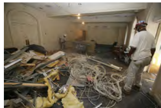
F081506PM-0013 [2018-0227-F_M1Hi_j0158_2.JPG] 8/15/2006 Press Briefing Room Renovations
