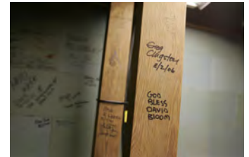
F080306PM-0091 [2018-0227-F_M1Hi_j0004.JPG] 8/3/2006 Clearing out Press Briefing room for renovations.
