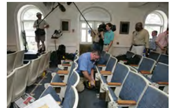
F080306PM-0055 [2018-0227-F_M1Hi_j0187.JPG] 8/3/2006 Clearing out Press Briefing room for renovations.
