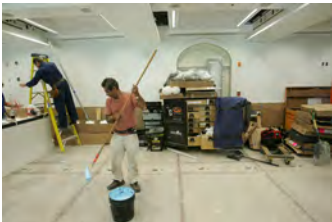
F062007CG-0086 [2018-0227-F_M2Hi_j0087.JPG] 6/20/2007 Work continues on the press briefing room
