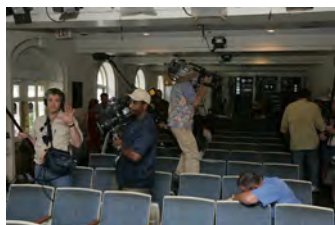
F080306PM-0037 [2018-0227-F_M1Hi_j0151.JPG] 8/3/2006 Clearing out Press Briefing room for renovations.
