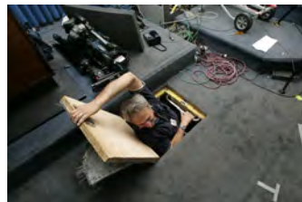
F080306PM-0019 [2018-0227-F_M1Hi_j0115.JPG] 8/3/2006 Clearing out Press Briefing room for renovations.
