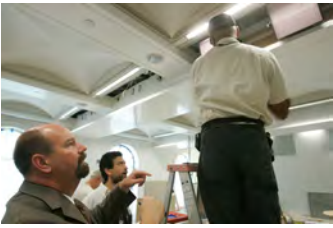
F061507CG-0065 [2018-0227-F_M2Hi_j0030.JPG] 6/15/2007 The Press Briefing Room nears completion
