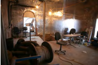
F120206PM-0033 [2018-0227-F_M1Hi_j0208_3.JPG] 12/2/2006 Press Briefing room renovations.
