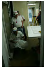
F062907CG-0050 [2018-0227-F_M1Hi_j0191_5.JPG] 6/29/2007 Work nears completion on the press briefing room, Friday June 29, 2007.
