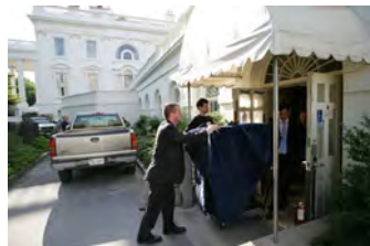
P062207ED-0033 [2018-0227-F_M1Hi_j0194_6.JPG] 6/22/2007 Press Briefing Room rennovations
