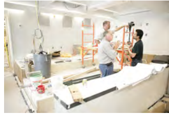
P062107ED-0211 [2018-0227-F_M1Hi_j0049_7.JPG] 6/21/2007 Press Briefing Room Renovations. West Wing.
