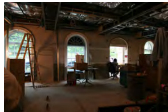
F051607SC-0084 [2018-0227-F_M1Hi_j0253_2.JPG] 5/16/2007 Press Briefing Room Renovations
