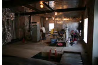
F010907PM-0009 [2018-0227-F_M1Hi_j0132_1.JPG] 1/9/2007 Press Briefing Room Renovations
