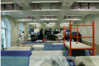
F062807CG-0059 [2018-0227-F_M1Hi_j0195_6.JPG] 6/28/2007 Work continues on the press briefing room
