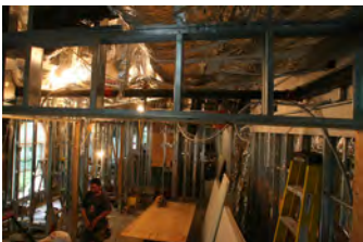
F051607SC-0066 [2018-0227-F_M1Hi_j0217_2.JPG] 5/16/2007 Press Briefing Room Renovations
