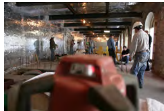
F010907PM-0017 [2018-0227-F_M1Hi_j0148_5.JPG] 1/9/2007 Press Briefing Room Renovations
