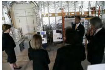
P040207SC-0051 [2018-0227-F_M1Hi_j0226_3.JPG] 4/2/2007 LB. The Brady Press Room During Renovations.
