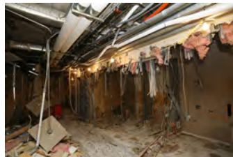
F081506PM-0029 [2018-0227-F_M1Hi_j0190_2.JPG] 8/15/2006 Press Briefing Room Renovations
