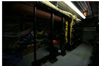
F061207DB-0033 [2018-0227-F_M1Hi_j0222_4.JPG] 6/12/2007 Brady Press Briefing Room Renovations
