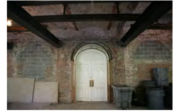
F101806KH-0014 [2018-0227-F_M1Hi_j0172_3.JPG] 10/18/2006 Press Room Renovations
