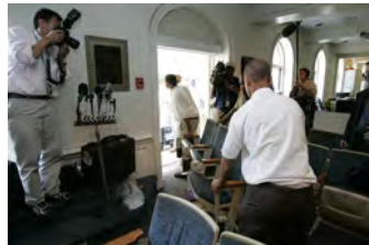
F080306PM-0109 [2018-0227-F_M1Hi_j0040.JPG] 8/3/2006 Clearing out Press Briefing room for renovations.
