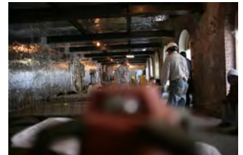
F010907PM-0014 [2018-0227-F_M1Hi_j0142_3.JPG] 1/9/2007 Press Briefing Room Renovations
