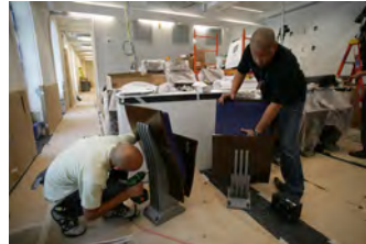
P062107ED-0319 [2018-0227-F_M1Hi_j0010_7.JPG] 6/21/2007 Press Briefing Room Renovations. West Wing.
