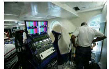
F062907CG-0060 [2018-0227-F_M1Hi_j0211_5.JPG] 6/29/2007 Work nears completion on the press briefing room, Friday June 29, 2007.
