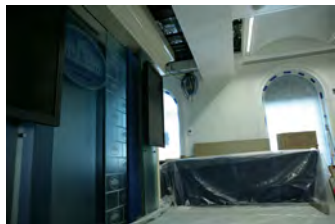
F062207CG-0062 [2018-0227-F_M1Hi_j0164_9.JPG] 6/22/2007 Work continues on the press briefing room
