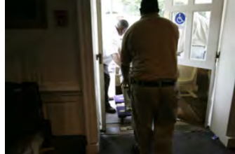
F080306PM-0125 [2018-0227-F_M1Hi_j0072.JPG] 8/3/2006 Clearing out Press Briefing room for renovations.
