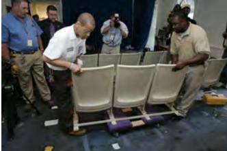
F080306PM-0124 [2018-0227-F_M1Hi_j0070.JPG] 8/3/2006 Clearing out Press Briefing room for renovations.
