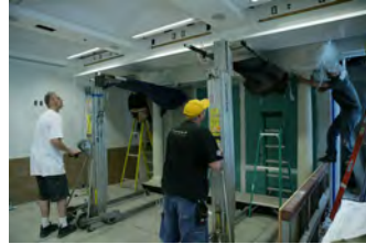
F062007CG-0044 [2018-0227-F_M2Hi_j0003.JPG] 6/20/2007 Work continues on the press briefing room
