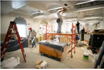
P062107ED-0229 [2018-0227-F_M1Hi_j0085_4.JPG] 6/21/2007 Press Briefing Room Renovations. West Wing.
