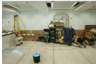
F062007CG-0087 [2018-0227-F_M2Hi_j0089.JPG] 6/20/2007 Work continues on the press briefing room
