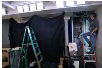
F070507CG-0057 [2018-0227-F_M1Hi_J0215_3.JPG] 7/5/2007 Work nears completion on the press briefing room and the Lower Press office.
