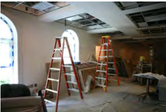
F053107LS-0004 [2018-0227-F_M1Hi_j0064_2.JPG] 5/31/2007 renovation progress of James S. Brady Press Briefing Room
