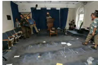
F080306PM-0150 [2018-0227-F_M1Hi_j0122.JPG] 8/3/2006 Clearing out Press Briefing room for renovations.
