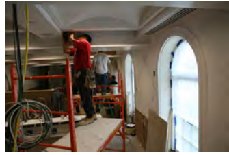
P061907DG-0209 [2018-0227-F_M1Hi_j0177_2.JPG] 6/19/2007 James S. Brady Press Briefing Room renovation
