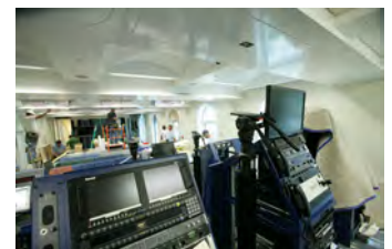
F062907CG-0028 [2018-0227-F_M1Hi_j0026_5.JPG] 6/29/2007 Work nears completion on the press briefing room, Friday June 29, 2007.
