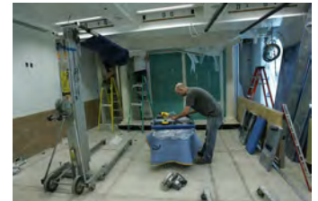
F062007CG-0049 [2018-0227-F_M2Hi_j0013.JPG] 6/20/2007 Work continues on the press briefing room
