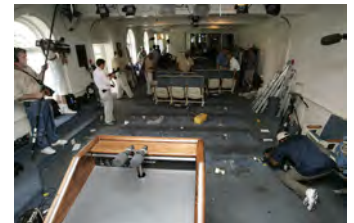
F080306PM-0155 [2018-0227-F_M1Hi_j0132.JPG] 8/3/2006 Clearing out Press Briefing room for renovations.
