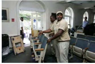
F080306PM-0141 [2018-0227-F_M1Hi_j0104.JPG] 8/3/2006 Clearing out Press Briefing room for renovations.
