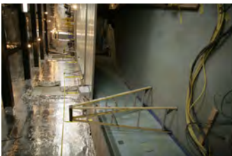
F121506PM-0006 [2018-0227-F_M1Hi_j0115_1.JPG] 12/15/2006 Press Briefing room renovations
