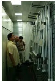
F070507CG-0060 [2018-0227-F_M1Hi_J0221_5.JPG] 7/5/2007 Work nears completion on the press briefing room and the Lower Press office.
