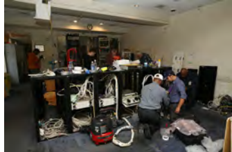
F080406PM-0014 [2018-0227-F_M1Hi_j0164_1.JPG] 8/4/2006 Clearing out Press Briefing room for renovations.
