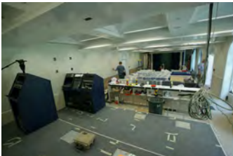
F062707CG-0021 [2018-0227-F_M1Hi_j0183_3.JPG] 6/27/2007 Work continues on the press briefing room
