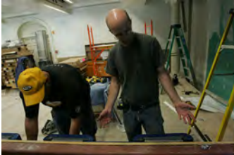
F062007CG-0082 [2018-0227-F_M2Hi_j0079.JPG] 6/20/2007 Work continues on the press briefing room
