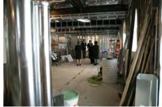
P040207SC-0043 [2018-0227-F_M1Hi_j0146_6.JPG] 4/2/2007 LB. The Brady Press Room During Renovations.
