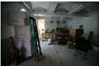
F061207DB-0056 [2018-0227-F_M1Hi_j0112_3.JPG] 6/12/2007 Brady Press Briefing Room Renovations
