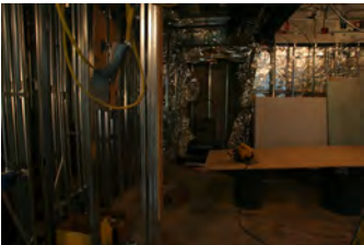
F051607SC-0078 [2018-0227-F_M1Hi_j0241_1.JPG] 5/16/2007 Press Briefing Room Renovations
