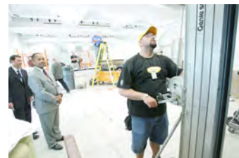
F062007CG-0033 [2018-0227-F_M2Hi_j0236.JPG] 6/20/2007 Work continues on the press briefing room
