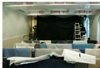
F070207CG-0002 [2018-0227-F_M1Hi_j0025_4.JPG] 7/2/2007 Work nears completion on the press briefing room
