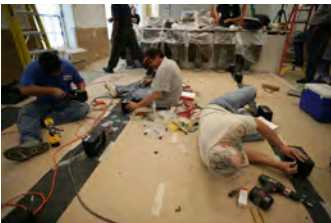
P062107ED-0301 [2018-0227-F_M1Hi_j0229_6.JPG] 6/21/2007 Press Briefing Room Renovations. West Wing.
