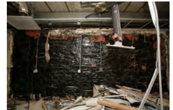
F081506PM-0027 [2018-0227-F_M1Hi_j0186_2.JPG] 8/15/2006 Press Briefing Room Renovations
