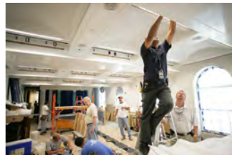
P062107ED-0243 [2018-0227-F_M1Hi_j0113_9.JPG] 6/21/2007 Press Briefing Room Renovations. West Wing.
