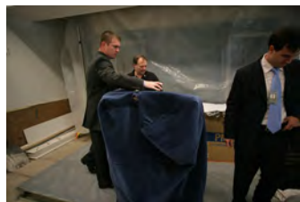
P062207ED-0042 [2018-0227-F_M1Hi_j0178_6.JPG] 6/22/2007 Press Briefing Room rennovations
