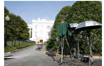
F081506PM-0047 [2018-0227-F_M1Hi_j0226_1.JPG] 8/15/2006 Press Briefing Room Renovations
