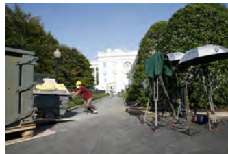
F081506PM-0050 [2018-0227-F_M1Hi_j0232_1.JPG] 8/15/2006 Press Briefing Room Renovations
