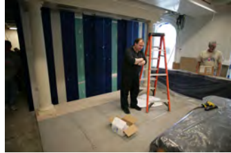
P062107ED-0234 [2018-0227-F_M1Hi_j0095_6.JPG] 6/21/2007 Press Briefing Room Renovations. West Wing.
