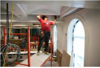
P061907DG-0208 [2018-0227-F_M1Hi_j0175_2.JPG] 6/19/2007 James S. Brady Press Briefing Room renovation
