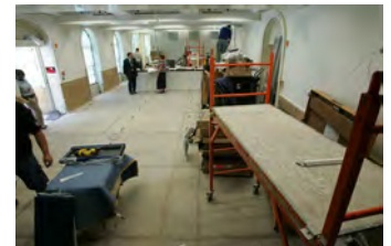
F062007CG-0073 [2018-0227-F_M2Hi_j0061.JPG] 6/20/2007 Work continues on the press briefing room
