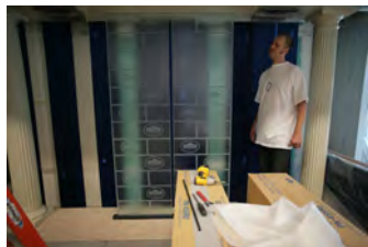
P062107ED-0266 [2018-0227-F_M1Hi_j0159_7.JPG] 6/21/2007 Press Briefing Room Renovations. West Wing.
