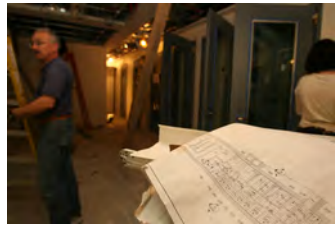
F051607SC-0131 [2018-0227-F_M1Hi_j0092_1.JPG] 5/16/2007 Press Briefing Room Renovations
