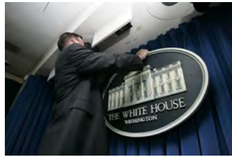
F080306PM-0061 [2018-0227-F_M1Hi_j0199.JPG] 8/3/2006 Clearing out Press Briefing room for renovations.
