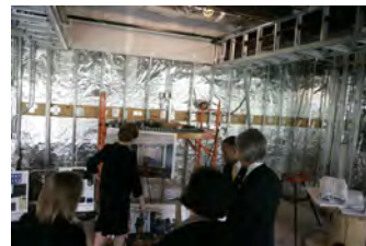
P040207SC-0056 [2018-0227-F_M1Hi_j0001_1.JPG] 4/2/2007 LB. The Brady Press Room During Renovations.
