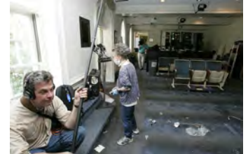
F080306PM-0167 [2018-0227-F_M1Hi_j0156.JPG] 8/3/2006 Clearing out Press Briefing room for renovations.
