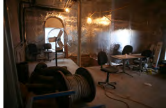
F120206PM-0034 [2018-0227-F_M1Hi_j0210_3.JPG] 12/2/2006 Press Briefing room renovations.
