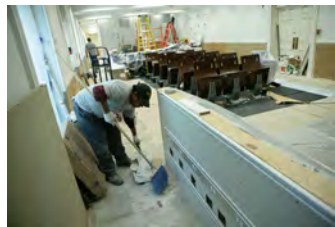
F062207CG-0011 [2018-0227-F_M1Hi_j0062_5.JPG] 6/22/2007 Work continues on the press briefing room
