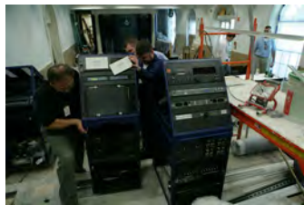
F062207CG-0054 [2018-0227-F_M1Hi_j0148_8.JPG] 6/22/2007 Work continues on the press briefing room
