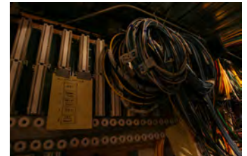
F051607SC-0041 [2018-0227-F_M1Hi_j0167_1.JPG] 5/16/2007 Press Briefing Room Renovations
