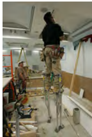
F061507CG-0033 [2018-0227-F_M2Hi_j0221.JPG] 6/15/2007 The Press Briefing Room nears completion
