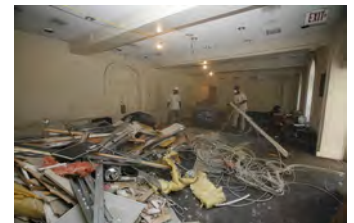
F081506PM-0014 [2018-0227-F_M1Hi_j0160_2.JPG] 8/15/2006 Press Briefing Room Renovations
