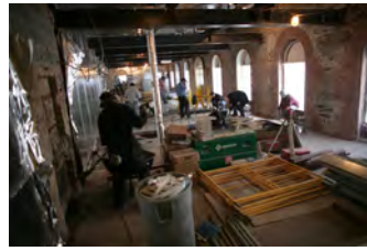
F010907PM-0025 [2018-0227-F_M1Hi_j0164_5.JPG] 1/9/2007 Press Briefing Room Renovations
