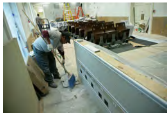
F062207CG-0010 [2018-0227-F_M1Hi_j0060_6.JPG] 6/22/2007 Work continues on the press briefing room
