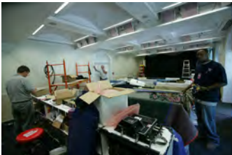
F070207CG-0024 [2018-0227-F_M1Hi_j0081_2.JPG] 7/2/2007 Work nears completion on the press briefing room
