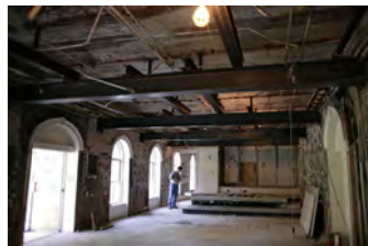
F091806PM-008 [2018-0227-F_M1Hi_j0133_1.JPG] 9/18/2006 Renovations of the Press Briefing Room
