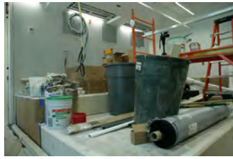
F062207CG-0034 [2018-0227-F_M1Hi_j0108_7.JPG] 6/22/2007 Work continues on the press briefing room
