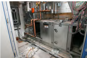
F051607SC-0146 [2018-0227-F_M1Hi_j0122_3.JPG] 5/16/2007 Press Briefing Room Renovations
