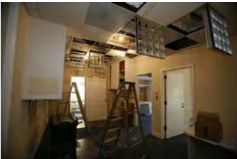
F081506PM-0044 [2018-0227-F_M1Hi_j0220_1.JPG] 8/15/2006 Press Briefing Room Renovations
