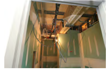
F051607SC-0113 [2018-0227-F_M1Hi_j0056_1.JPG] 5/16/2007 Press Briefing Room Renovations
