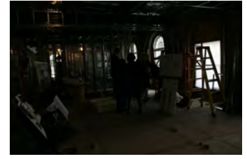
P040207SC-0001 [2018-0227-F_M1Hi_j0176_5.JPG] 4/2/2007 LB. The Brady Press Room During Renovations.
