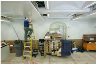
F062007CG-0070 [2018-0227-F_M2Hi_j0055.JPG] 6/20/2007 Work continues on the press briefing room
