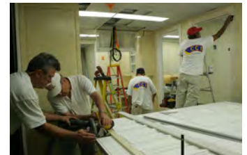
F062907CG-0044 [2018-0227-F_M1Hi_j0179_5.JPG] 6/29/2007 Work nears completion on the press briefing room, Friday June 29, 2007.
