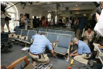
F080306PM-0017 [2018-0227-F_M1Hi_j0111.JPG] 8/3/2006 Clearing out Press Briefing room for renovations.
