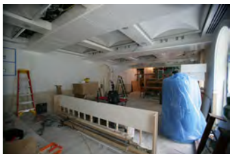
F061207DB-0012 [2018-0227-F_M1Hi_j0089_1.JPG] 6/12/2007 Brady Press Briefing Room Renovations
