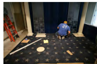
P062107ED-0352 [2018-0227-F_M1Hi_j0076_6.JPG] 6/21/2007 Press Briefing Room Renovations. West Wing.
