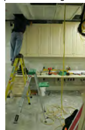
F062807CG-0054 [2018-0227-F_M1Hi_j0185_3.JPG] 6/28/2007 Work continues on the press briefing room
