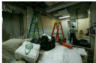
F062707CG-0051 [2018-0227-F_M1Hi_j0061_3.JPG] 6/27/2007 Work continues on the press briefing room
