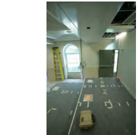
F062707CG-0020 [2018-0227-F_M1Hi_j0179_3.JPG] 6/27/2007 Work continues on the press briefing room
