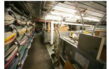
F061207DB-0031 [2018-0227-F_M1Hi_j0210_4.JPG] 6/12/2007 Brady Press Briefing Room Renovations
