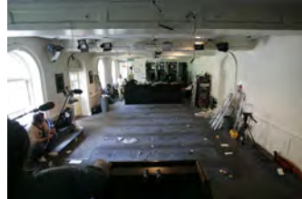
F080306PM-0186 [2018-0227-F_M1Hi_j0194.JPG] 8/3/2006 Clearing out Press Briefing room for renovations.
