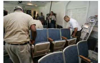
F080306PM-0111 [2018-0227-F_M1Hi_j0044.JPG] 8/3/2006 Clearing out Press Briefing room for renovations.
