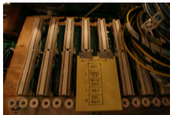
F051607SC-0047 [2018-0227-F_M1Hi_j0179_1.JPG] 5/16/2007 Press Briefing Room Renovations
