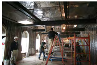
F012507PM-0032 [2018-0227-F_M1Hi_j0077.JPG] 1/25/2007 Press Briefing room renovations.
