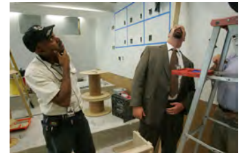
F061507CG-0076 [2018-0227-F_M2Hi_j0052.JPG] 6/15/2007 The Press Briefing Room nears completion
