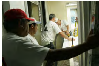
F062907CG-0039 [2018-0227-F_M1Hi_j0169_4.JPG] 6/29/2007 Work nears completion on the press briefing room, Friday June 29, 2007.
