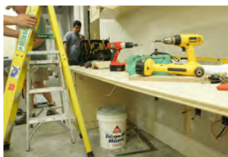
F062807CG-0049 [2018-0227-F_M1Hi_j0175_5.JPG] 6/28/2007 Work continues on the press briefing room
