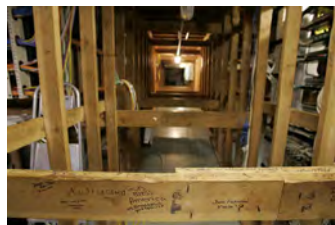
F080306PM-0073 [2018-0227-F_M1Hi_j0223.JPG] 8/3/2006 Clearing out Press Briefing room for renovations.
