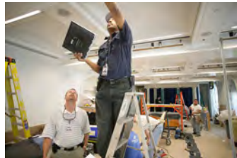
P062107ED-0238 [2018-0227-F_M1Hi_j0103_8.JPG] 6/21/2007 Press Briefing Room Renovations. West Wing.
