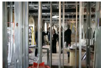
P040207SC-0016 [2018-0227-F_M1Hi_j0244_2.JPG] 4/2/2007 LB. The Brady Press Room During Renovations.
