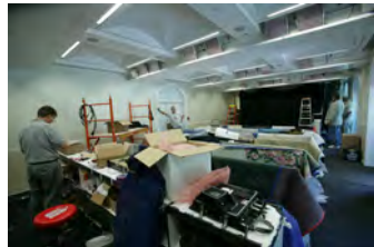
F070207CG-0025 [2018-0227-F_M1Hi_j0083_3.JPG] 7/2/2007 Work nears completion on the press briefing room
