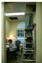
F070507CG-0001 [2018-0227-F_M1Hi_j0103_6.JPG] 7/5/2007 Work nears completion on the press briefing room and Lower Press office.
