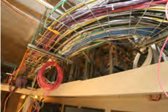
F051607SC-0134 [2018-0227-F_M1Hi_j0098_1.JPG] 5/16/2007 Press Briefing Room Renovations
