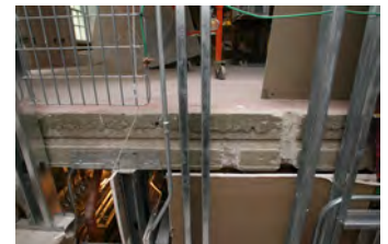
F051607SC-0149 [2018-0227-F_M1Hi_j0128_3.JPG] 5/16/2007 Press Briefing Room Renovations
