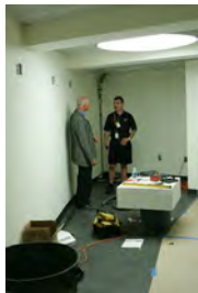
F062707CG-0029 [2018-0227-F_M1Hi_j0215_4.JPG] 6/27/2007 Work continues on the press briefing room
