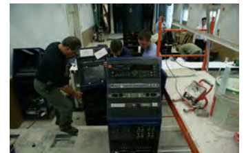
F062207CG-0052 [2018-0227-F_M1Hi_j0144_8.JPG] 6/22/2007 Work continues on the press briefing room
