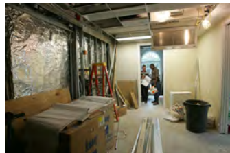
F061507CG-0015 [2018-0227-F_M2Hi_j0185.JPG] 6/15/2007 The Press Briefing Room nears completion
