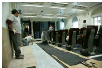
F062207CG-0003 [2018-0227-F_M1Hi_j0046_7.JPG] 6/22/2007 Work continues on the press briefing room
