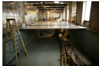
F121506PM-0004 [2018-0227-F_M1Hi_j0111_1.JPG] 12/15/2006 Press Briefing room renovations
