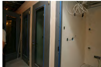
F051607SC-0140 [2018-0227-F_M1Hi_j0110_2.JPG] 5/16/2007 Press Briefing Room Renovations
