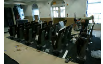
F062207CG-0080 [2018-0227-F_M1Hi_j0200_7.JPG] 6/22/2007 Work continues on the press briefing room
