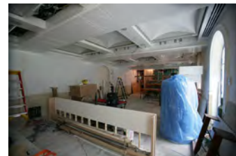
F061207DB-0011 [2018-0227-F_M1Hi_j0083_1.JPG] 6/12/2007 Brady Press Briefing Room Renovations
