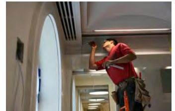
P061907DG-0239 [2018-0227-F_M1Hi_j0237_2.JPG] 6/19/2007 James S. Brady Press Briefing Room renovation
