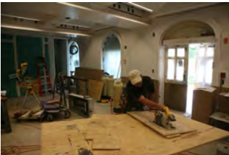
P061907DG-0216 [2018-0227-F_M1Hi_j0191_2.JPG] 6/19/2007 James S. Brady Press Briefing Room renovation
