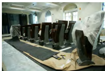
F062207CG-0002 [2018-0227-F_M1Hi_j0044_6.JPG] 6/22/2007 Work continues on the press briefing room
