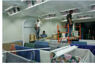
F062907CG-0031 [2018-0227-F_M1Hi_j0032_4.JPG] 6/29/2007 Work nears completion on the press briefing room, Friday June 29, 2007.
