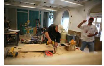
P061907DG-0211 [2018-0227-F_M1Hi_j0181_2.JPG] 6/19/2007 James S. Brady Press Briefing Room renovation
