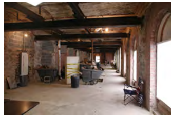
F110106PM-0001 [2018-0227-F_M1Hi_j0015.JPG] 11/1/2006 Press Briefing room renovations
