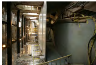
F121506PM-0008 [2018-0227-F_M1Hi_j0119_1.JPG] 12/15/2006 Press Briefing room renovations
