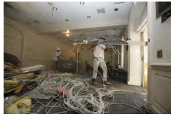
F081506PM-0017 [2018-0227-F_M1Hi_j0166_2.JPG] 8/15/2006 Press Briefing Room Renovations
