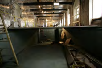
F121506PM-0010 [2018-0227-F_M1Hi_j0123_1.JPG] 12/15/2006 Press Briefing room renovations
