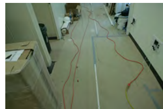
F062207CG-0028 [2018-0227-F_M1Hi_j0096_6.JPG] 6/22/2007 Work continues on the press briefing room
