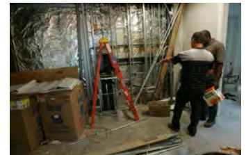
F061507CG-0017 [2018-0227-F_M2Hi_j0189.JPG] 6/15/2007 The Press Briefing Room nears completion
