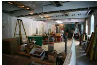
F053107LS-0005 [2018-0227-F_M1Hi_j0066_4.JPG] 5/31/2007 renovation progress of James S. Brady Press Briefing Room
