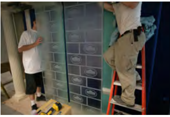
P062107ED-0289 [2018-0227-F_M1Hi_j0205_6.JPG] 6/21/2007 Press Briefing Room Renovations. West Wing.
