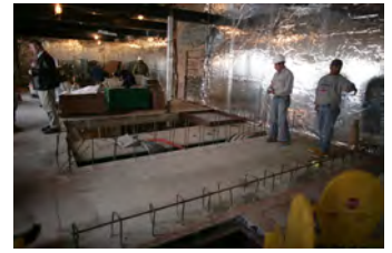
F010907PM-0006 [2018-0227-F_M1Hi_j0126_1.JPG] 1/9/2007 Press Briefing Room Renovations
