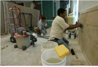
F061507CG-0002 [2018-0227-F_M2Hi_j0159.JPG] 6/15/2007 The Press Briefing Room nears completion
