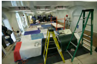
F062807CG-0024 [2018-0227-F_M1Hi_j0125_6.JPG] 6/28/2007 Work continues on the press briefing room
