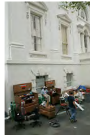
F062907CG-0055 [2018-0227-F_M1Hi_j0201_3.JPG] 6/29/2007 Work nears completion on the press briefing room, Friday June 29, 2007.
