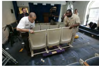
F080306PM-0121 [2018-0227-F_M1Hi_j0064.JPG] 8/3/2006 Clearing out Press Briefing room for renovations.
