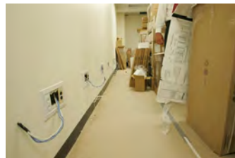
F061907CG-0011 [2018-0227-F_M2Hi_j0199_1.JPG] 6/19/2007 Work continues on the Brady Briefing Room
