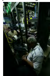
F062807CG-0046 [2018-0227-F_M1Hi_j0169_3.JPG] 6/28/2007 Work continues on the press briefing room
