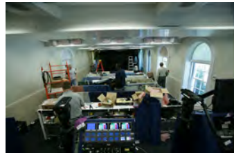
F070207CG-0026 [2018-0227-F_M1Hi_j0085_1.JPG] 7/2/2007 Work nears completion on the press briefing room
