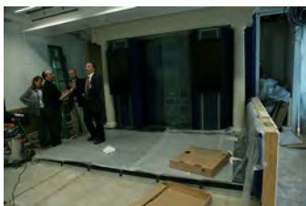
F062207CG-0001 [2018-0227-F_M1Hi_j0042_5.JPG] 6/22/2007 Work continues on the press briefing room
