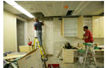
F062807CG-0026 [2018-0227-F_M1Hi_j0129_3.JPG] 6/28/2007 Work continues on the press briefing room
