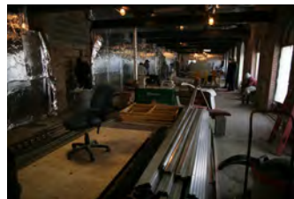
F010907PM-0021 [2018-0227-F_M1Hi_j0156_5.JPG] 1/9/2007 Press Briefing Room Renovations
