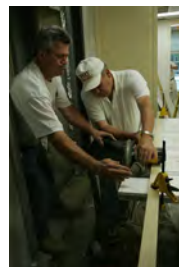
F062907CG-0047 [2018-0227-F_M1Hi_j0185_4.JPG] 6/29/2007 Work nears completion on the press briefing room, Friday June 29, 2007.
