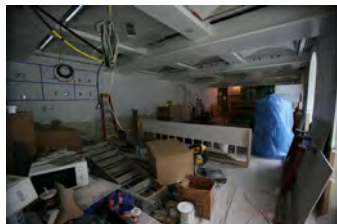
F061207DB-0009 [2018-0227-F_M1Hi_j0071_1.JPG] 6/12/2007 Brady Press Briefing Room Renovations
