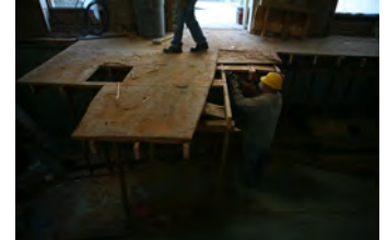
F120206PM-0036 [2018-0227-F_M1Hi_j0214_3.JPG] 12/2/2006 Press Briefing room renovations.
