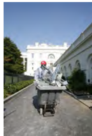
F081506PM-0054 [2018-0227-F_M1Hi_j0240_1.JPG] 8/15/2006 Press Briefing Room Renovations
