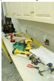
F062807CG-0051 [2018-0227-F_M1Hi_j0179_4.JPG] 6/28/2007 Work continues on the press briefing room
