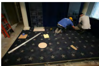
P062107ED-0349 [2018-0227-F_M1Hi_j0070_6.JPG] 6/21/2007 Press Briefing Room Renovations. West Wing.
