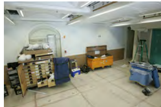
F062007CG-0068 [2018-0227-F_M2Hi_j0051.JPG] 6/20/2007 Work continues on the press briefing room
