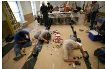
P062107ED-0298 [2018-0227-F_M1Hi_j0223_5.JPG] 6/21/2007 Press Briefing Room Renovations. West Wing.
