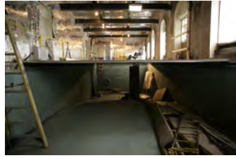
F121506PM-0011 [2018-0227-F_M1Hi_j0125_1.JPG] 12/15/2006 Press Briefing room renovations
