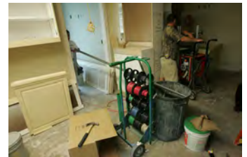
F061907CG-0008 [2018-0227-F_M2Hi_j0193_1.JPG] 6/19/2007 Work continues on the Brady Briefing Room
