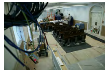
F062207CG-0068 [2018-0227-F_M1Hi_j0176_6.JPG] 6/22/2007 Work continues on the press briefing room
