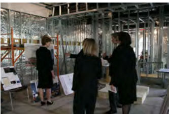
P040207SC-0054 [2018-0227-F_M1Hi_j0244_3.JPG] 4/2/2007 LB. The Brady Press Room During Renovations.
