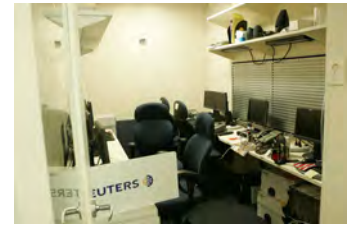
F070207CG-0017 [2018-0227-F_M1Hi_j0111_4.JPG] 7/2/2007 Work nears completion on the press briefing room
