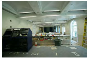
F062707CG-0014 [2018-0227-F_M1Hi_j0155_4.JPG] 6/27/2007 Work continues on the press briefing room
