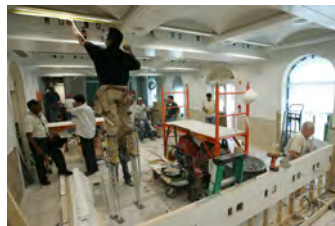
F061507CG-0034 [2018-0227-F_M2Hi_j0223.JPG] 6/15/2007 The Press Briefing Room nears completion
