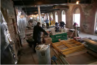
F010907PM-0027 [2018-0227-F_M1Hi_j0168_5.JPG] 1/9/2007 Press Briefing Room Renovations
