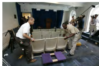
F080306PM-0118 [2018-0227-F_M1Hi_j0058.JPG] 8/3/2006 Clearing out Press Briefing room for renovations.
