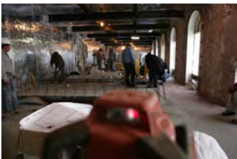
F010907PM-0019 [2018-0227-F_M1Hi_j0152_5.JPG] 1/9/2007 Press Briefing Room Renovations
