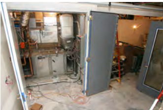
F051607SC-0142 [2018-0227-F_M1Hi_j0114_3.JPG] 5/16/2007 Press Briefing Room Renovations
