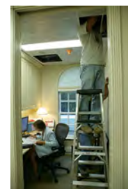
F070507CG-0003 [2018-0227-F_M1Hi_j0107_5.JPG] 7/5/2007 Work nears completion on the press briefing room and Lower Press office.
