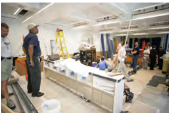
P062107ED-0205 [2018-0227-F_M1Hi_j0037_2.JPG] 6/21/2007 Press Briefing Room Renovations. West Wing.
