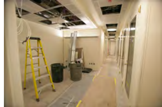
F061207DB-0046 [2018-0227-F_M1Hi_j0052_2.JPG] 6/12/2007 Brady Press Briefing Room Renovations
