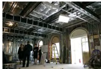
P040207SC-0036 [2018-0227-F_M1Hi_j0108_1.JPG] 4/2/2007 LB. The Brady Press Room During Renovations.
