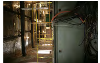
F121506PM-0021 [2018-0227-F_M1Hi_j0145_1.JPG] 12/15/2006 Press Briefing room renovations
