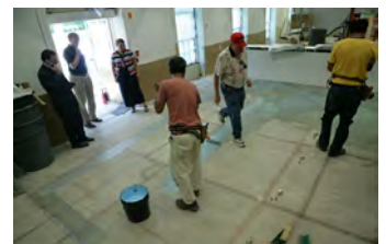
F062007CG-0097 [2018-0227-F_M2Hi_j0109.JPG] 6/20/2007 Work continues on the press briefing room
