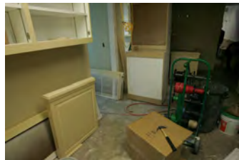
F061907CG-0006 [2018-0227-F_M2Hi_j0189_1.JPG] 6/19/2007 Work continues on the Brady Briefing Room
