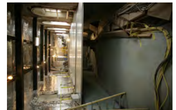
F121506PM-0009 [2018-0227-F_M1Hi_j0121_1.JPG] 12/15/2006 Press Briefing room renovations
