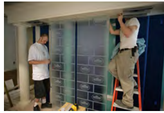
P062107ED-0291 [2018-0227-F_M1Hi_j0209_4.JPG] 6/21/2007 Press Briefing Room Renovations. West Wing.
