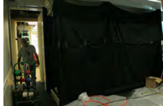
F070207CG-0013 [2018-0227-F_M1Hi_j0095_3.JPG] 7/2/2007 Work nears completion on the press briefing room
