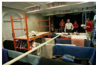
F070507CG-0042 [2018-0227-F_M1Hi_j0185_5.JPG] 7/5/2007 Work nears completion on the press briefing room and the Lower Press office.
