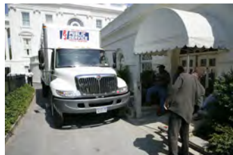
P062107ED-0326 [2018-0227-F_M1Hi_j0024_5.JPG] 6/21/2007 Press Briefing Room Renovations. West Wing.
