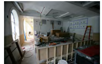
F061207DB-0055 [2018-0227-F_M1Hi_j0106_4.JPG] 6/12/2007 Brady Press Briefing Room Renovations
