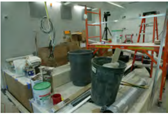
F062207CG-0033 [2018-0227-F_M1Hi_j0106_6.JPG] 6/22/2007 Work continues on the press briefing room
