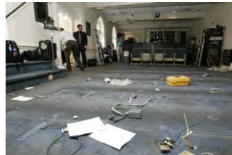
F080306PM-0170 [2018-0227-F_M1Hi_j0162.JPG] 8/3/2006 Clearing out Press Briefing room for renovations.
