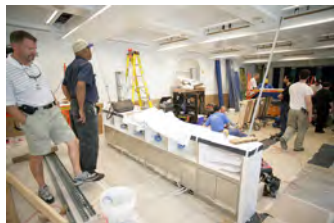
P062107ED-0206 [2018-0227-F_M1Hi_j0039_2.JPG] 6/21/2007 Press Briefing Room Renovations. West Wing.
