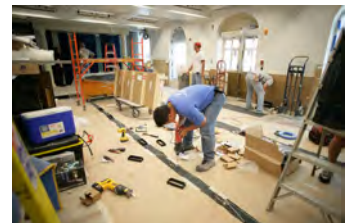
P062107ED-0248 [2018-0227-F_M1Hi_j0123_6.JPG] 6/21/2007 Press Briefing Room Renovations. West Wing.
