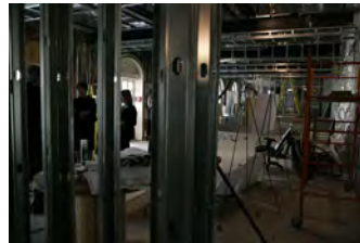
P040207SC-0008 [2018-0227-F_M1Hi_j0204_5.JPG] 4/2/2007 LB. The Brady Press Room During Renovations.
