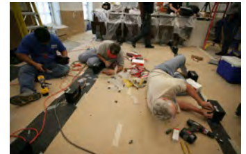
P062107ED-0300 [2018-0227-F_M1Hi_j0227_8.JPG] 6/21/2007 Press Briefing Room Renovations. West Wing.
