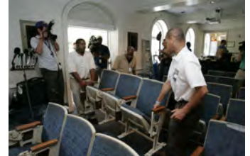
F080306PM-0107 [2018-0227-F_M1Hi_j0036.JPG] 8/3/2006 Clearing out Press Briefing room for renovations.
