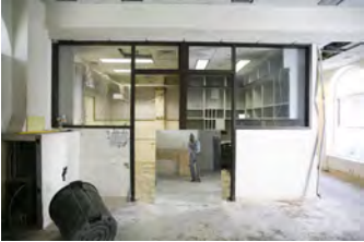
F081506PM-0040 [2018-0227-F_M1Hi_j0212_1.JPG] 8/15/2006 Press Briefing Room Renovations
