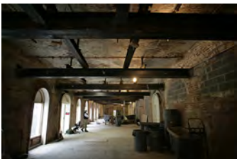
F101906PM-011 [2018-0227-F_M1Hi_j0242_2.JPG] 10/19/2006 Renovations to the Press Briefing room
