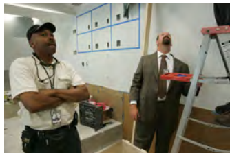
F061507CG-0078 [2018-0227-F_M2Hi_j0056.JPG] 6/15/2007 The Press Briefing Room nears completion
