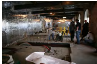
F010907PM-0012 [2018-0227-F_M1Hi_j0138_3.JPG] 1/9/2007 Press Briefing Room Renovations
