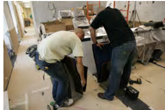
P062107ED-0322 [2018-0227-F_M1Hi_j0016_5.JPG] 6/21/2007 Press Briefing Room Renovations. West Wing.
