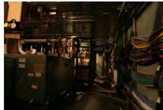
F051607SC-0020 [2018-0227-F_M1Hi_j0088_1.JPG] 5/16/2007 Press Briefing Room Renovations
