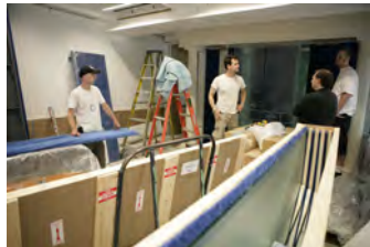
P062107ED-0258 [2018-0227-F_M1Hi_j0143_5.JPG] 6/21/2007 Press Briefing Room Renovations. West Wing.
