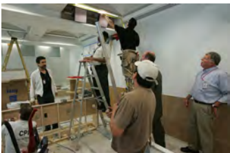
F061507CG-0061 [2018-0227-F_M2Hi_j0022.JPG] 6/15/2007 The Press Briefing Room nears completion
