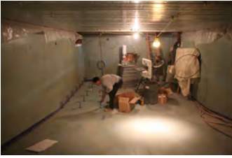
F012507PM-0014 [2018-0227-F_M1Hi_j0041.JPG] 1/25/2007 Press Briefing room renovations.
