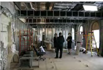
P040207SC-0034 [2018-0227-F_M1Hi_j0096_1.JPG] 4/2/2007 LB. The Brady Press Room During Renovations.
