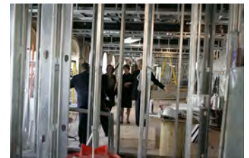
P040207SC-0017 [2018-0227-F_M1Hi_j0250.JPG] 4/2/2007 LB. The Brady Press Room During Renovations.
