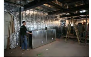
F012507PM-0001 [2018-0227-F_M1Hi_j0015_1.JPG] 1/25/2007 Press Briefing room renovations.
