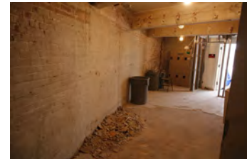
F110106PM-0005 [2018-0227-F_M1Hi_j0103_1.JPG] 11/1/2006 Press Briefing room renovations
