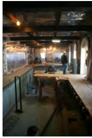
F120206PM-0009 [2018-0227-F_M1Hi_j0160_4.JPG] 12/2/2006 Press Briefing room renovations.
