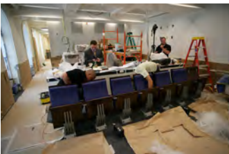
P062107ED-0325 [2018-0227-F_M1Hi_j0022_8.JPG] 6/21/2007 Press Briefing Room Renovations. West Wing.
