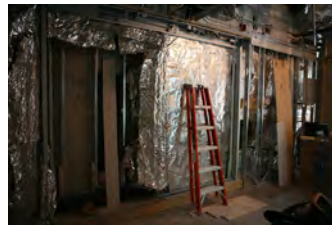
F053107LS-0010 [2018-0227-F_M1Hi_j0076_3.JPG] 5/31/2007 renovation progress of James S. Brady Press Briefing Room
