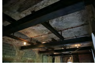
F101806KH-0017 [2018-0227-F_M1Hi_j0178_3.JPG] 10/18/2006 Press Room Renovations
