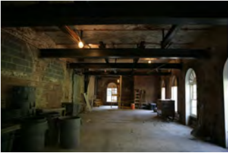
F101806KH-0011 [2018-0227-F_M1Hi_j0166_3.JPG] 10/18/2006 Press Room Renovations
