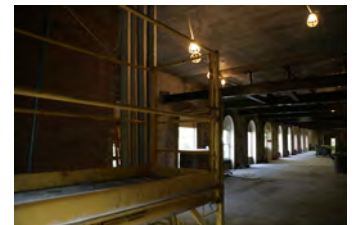
F101806KH-0030 [2018-0227-F_M1Hi_j0204_3.JPG] 10/18/2006 Press Room Renovations
