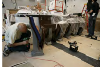
P062107ED-0315 [2018-0227-F_M1Hi_j0002_5.JPG] 6/21/2007 Press Briefing Room Renovations. West Wing.
