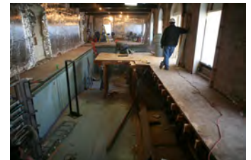
F120206PM-0004 [2018-0227-F_M1Hi_j0150_4.JPG] 12/2/2006 Press Briefing room renovations.
