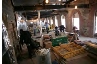
F010907PM-0029 [2018-0227-F_M1Hi_j0172_5.JPG] 1/9/2007 Press Briefing Room Renovations
