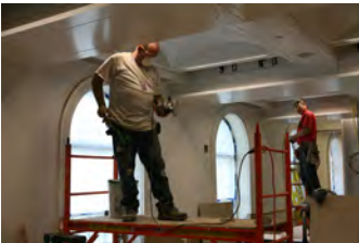
P061907DG-0236 [2018-0227-F_M1Hi_j0231_2.JPG] 6/19/2007 James S. Brady Press Briefing Room renovation
