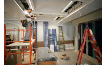
P062107ED-0212 [2018-0227-F_M1Hi_j0051_3.JPG] 6/21/2007 Press Briefing Room Renovations. West Wing.
