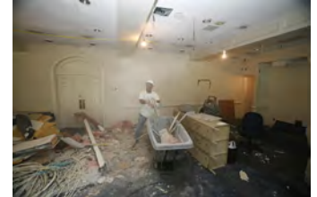
F081506PM-0002 [2018-0227-F_M1Hi_j0136_1.JPG] 8/15/2006 Press Briefing Room Renovations
