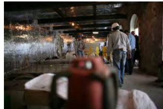
F010907PM-0013 [2018-0227-F_M1Hi_j0140_3.JPG] 1/9/2007 Press Briefing Room Renovations
