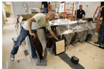
P062107ED-0306 [2018-0227-F_M1Hi_j0239_7.JPG] 6/21/2007 Press Briefing Room Renovations. West Wing.
