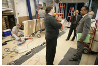
P062107ED-0210 [2018-0227-F_M1Hi_j0047_1.JPG] 6/21/2007 Press Briefing Room Renovations. West Wing.
