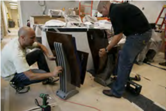
P062107ED-0317 [2018-0227-F_M1Hi_j0006_6.JPG] 6/21/2007 Press Briefing Room Renovations. West Wing.
