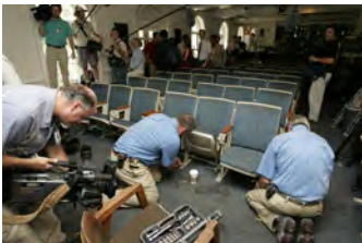
F080306PM-0013 [2018-0227-F_M1Hi_j0103.JPG] 8/3/2006 Clearing out Press Briefing room for renovations.
