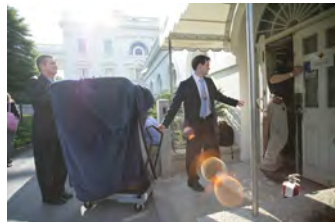
P062207ED-0025 [2018-0227-F_M1Hi_j0164_6.JPG] 6/22/2007 Press Briefing Room rennovations
