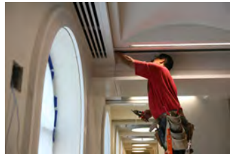
P061907DG-0237 [2018-0227-F_M1Hi_j0233_3.JPG] 6/19/2007 James S. Brady Press Briefing Room renovation
