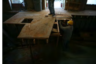
F120206PM-0035 [2018-0227-F_M1Hi_j0212_3.JPG] 12/2/2006 Press Briefing room renovations.
