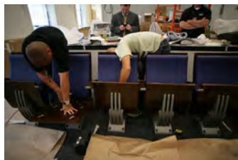
P062107ED-0334 [2018-0227-F_M1Hi_j0040_5.JPG] 6/21/2007 Press Briefing Room Renovations. West Wing.
