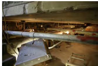
F101806KH-0024 [2018-0227-F_M1Hi_j0192_3.JPG] 10/18/2006 Press Room Renovations
