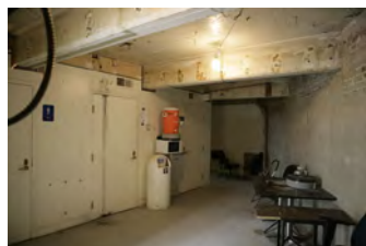
F101806KH-0008 [2018-0227-F_M1Hi_j0160_3.JPG] 10/18/2006 Press Room Renovations
