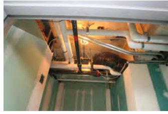
F051607SC-0111 [2018-0227-F_M1Hi_j0052_1.JPG] 5/16/2007 Press Briefing Room Renovations
