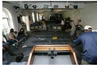
F080306PM-0162 [2018-0227-F_M1Hi_j0146.JPG] 8/3/2006 Clearing out Press Briefing room for renovations.
