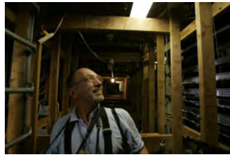
F080306PM-0101 [2018-0227-F_M1Hi_j0024.JPG] 8/3/2006 Clearing out Press Briefing room for renovations.
