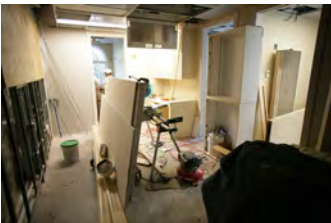
P062107ED-0221 [2018-0227-F_M1Hi_j0069_5.JPG] 6/21/2007 Press Briefing Room Renovations. West Wing.
