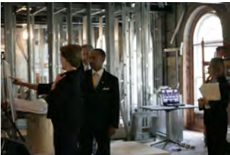
P040207SC-0046 [2018-0227-F_M1Hi_j0196_6.JPG] 4/2/2007 LB. The Brady Press Room During Renovations.
