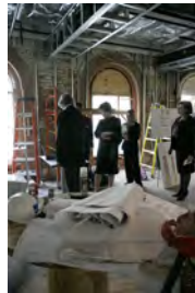
P040207SC-0023 [2018-0227-F_M1Hi_j0030_2.JPG] 4/2/2007 LB. The Brady Press Room During Renovations.
