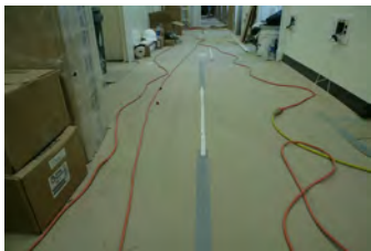
F062207CG-0029 [2018-0227-F_M1Hi_j0098_3.JPG] 6/22/2007 Work continues on the press briefing room
