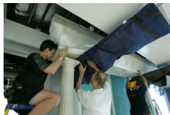
F062007CG-0032 [2018-0227-F_M2Hi_j0234.JPG] 6/20/2007 Work continues on the press briefing room
