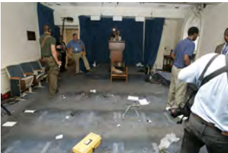
F080306PM-0148 [2018-0227-F_M1Hi_j0118.JPG] 8/3/2006 Clearing out Press Briefing room for renovations.
