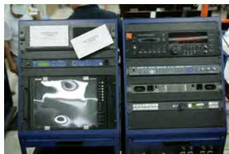
F062207CG-0058 [2018-0227-F_M1Hi_j0156_7.JPG] 6/22/2007 Work continues on the press briefing room
