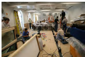
P062107ED-0278 [2018-0227-F_M1Hi_j0183_9.JPG] 6/21/2007 Press Briefing Room Renovations. West Wing.
