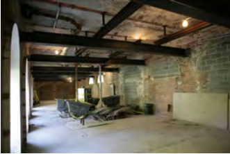
F101806KH-0015 [2018-0227-F_M1Hi_j0174_3.JPG] 10/18/2006 Press Room Renovations
