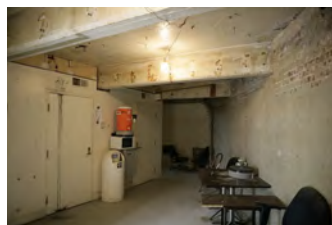
F101806KH-0009 [2018-0227-F_M1Hi_j0162_2.JPG] 10/18/2006 Press Room Renovations
