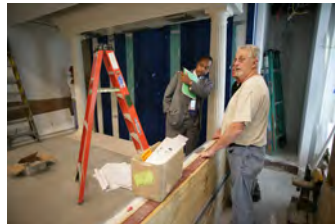
P062107ED-0218 [2018-0227-F_M1Hi_j0063_4.JPG] 6/21/2007 Press Briefing Room Renovations. West Wing.
