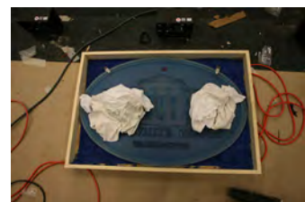
F062107DG-0025 [2018-0227-F_M1Hi_j0125_3.JPG] 6/21/2007 White House Press Briefing Room renovations Thursday, June 21, 2007. White House photo by Debra Gulbas
