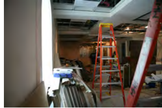
F053107LS-0002 [2018-0227-F_M1Hi_j0060_3.JPG] 5/31/2007 renovation progress of James S. Brady Press Briefing Room
