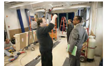
P062107ED-0208 [2018-0227-F_M1Hi_j0043_3.JPG] 6/21/2007 Press Briefing Room Renovations. West Wing.
