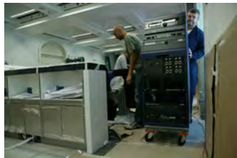
F062207CG-0046 [2018-0227-F_M1Hi_j0132_7.JPG] 6/22/2007 Work continues on the press briefing room
