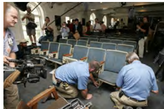
F080306PM-0014 [2018-0227-F_M1Hi_j0105.JPG] 8/3/2006 Clearing out Press Briefing room for renovations.
