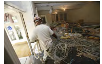
F081506PM-0010 [2018-0227-F_M1Hi_j0152_2.JPG] 8/15/2006 Press Briefing Room Renovations
