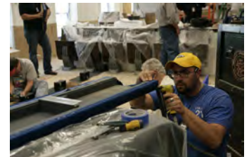
P062107ED-0304 [2018-0227-F_M1Hi_j0235_6.JPG] 6/21/2007 Press Briefing Room Renovations. West Wing.
