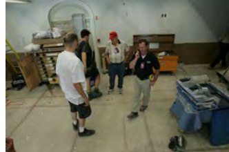
F062007CG-0064 [2018-0227-F_M2Hi_j0043.JPG] 6/20/2007 Work continues on the press briefing room
