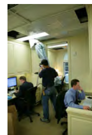
F070507CG-0007 [2018-0227-F_M1Hi_j0115_5.JPG] 7/5/2007 Work nears completion on the press briefing room and Lower Press office.
