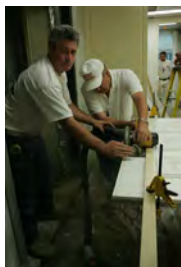
F062907CG-0045 [2018-0227-F_M1Hi_j0181_4.JPG] 6/29/2007 Work nears completion on the press briefing room, Friday June 29, 2007.
