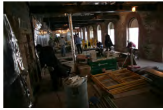
F010907PM-0024 [2018-0227-F_M1Hi_j0162_4.JPG] 1/9/2007 Press Briefing Room Renovations
