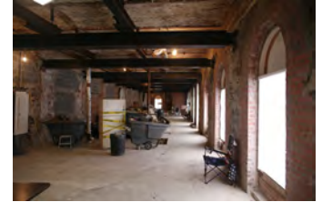
F110106PM-0003 [2018-0227-F_M1Hi_j0099_1.JPG] 11/1/2006 Press Briefing room renovations
