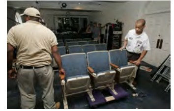
F080306PM-0143 [2018-0227-F_M1Hi_j0108.JPG] 8/3/2006 Clearing out Press Briefing room for renovations.
