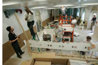
F061507CG-0008 [2018-0227-F_M2Hi_j0171.JPG] 6/15/2007 The Press Briefing Room nears completion
