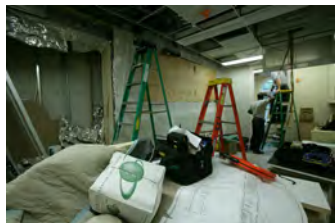
F062707CG-0050 [2018-0227-F_M1Hi_j0057_1.JPG] 6/27/2007 Work continues on the press briefing room
