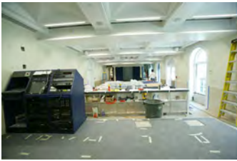
F062707CG-0013 [2018-0227-F_M1Hi_j0151_3.JPG] 6/27/2007 Work continues on the press briefing room
