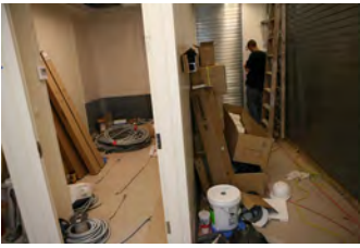
P061907DG-0248 [2018-0227-F_M1Hi_j0255_3.JPG] 6/19/2007 James S. Brady Press Briefing Room renovation
