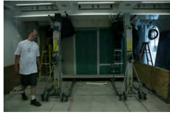
F062007CG-0039 [2018-0227-F_M2Hi_j0248.JPG] 6/20/2007 Work continues on the press briefing room
