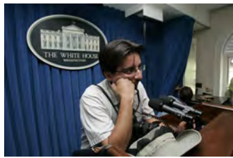
F080306PM-0022 [2018-0227-F_M1Hi_j0121.JPG] 8/3/2006 Clearing out Press Briefing room for renovations.
