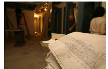
F051607SC-0129 [2018-0227-F_M1Hi_j0088_2.JPG] 5/16/2007 Press Briefing Room Renovations
