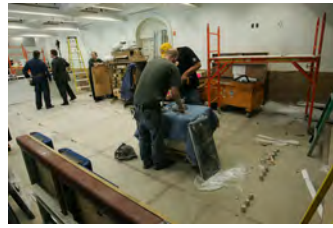
F062007CG-0080 [2018-0227-F_M2Hi_j0075.JPG] 6/20/2007 Work continues on the press briefing room
