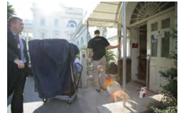
P062207ED-0027 [2018-0227-F_M1Hi_j0193_3.JPG] 6/22/2007 Press Briefing Room rennovations
