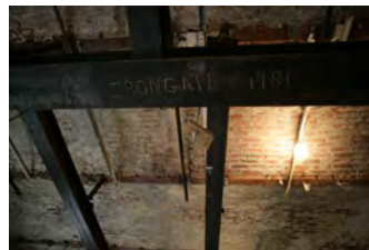
F101906PM-033 [2018-0227-F_M1Hi_j0034_1.JPG] 10/19/2006 Renovations to the Press Briefing room
