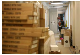
P061907DG-0250 [2018-0227-F_M1Hi_j0004_4.JPG] 6/19/2007 James S. Brady Press Briefing Room renovation
