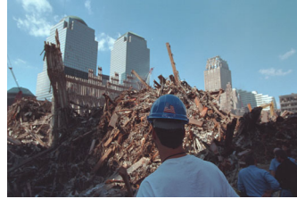
P8045-13 [Hi_j0057_1.JPG] 10/3/2001 VIEWS OF GROUND ZERO
