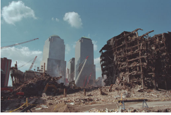
P8045-07 [Hi_j0063_1.JPG] 10/3/2001 VIEWS OF GROUND ZERO
