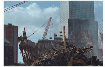
P8049-03 [Hi_j0049_1.JPG] 10/3/2001 VIEWS OF GROUND ZERO
