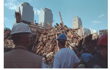
P8045-10 [Hi_j0060_1.JPG] 10/3/2001 VIEWS OF GROUND ZERO
