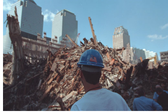
P8045-12 [Hi_j0058_1.JPG] 10/3/2001 VIEWS OF GROUND ZERO
