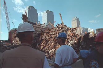
P8045-11 [Hi_j0059_1.JPG] 10/3/2001 VIEWS OF GROUND ZERO
