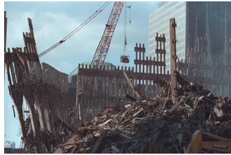
P8049-01 [Hi_j0051_2.JPG] 10/3/2001 VIEWS OF GROUND ZERO
