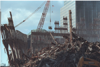
P8049-04 [Hi_j0048_1.JPG] 10/3/2001 VIEWS OF GROUND ZERO
