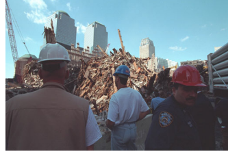
P8045-09 [Hi_j0061_1.JPG] 10/3/2001 VIEWS OF GROUND ZERO
