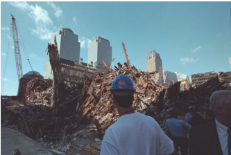
P8045-15 [Hi_j0055_1.JPG] 10/3/2001 VIEWS OF GROUND ZERO
