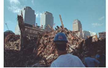
P8045-14 [Hi_j0056_1.JPG] 10/3/2001 VIEWS OF GROUND ZERO
