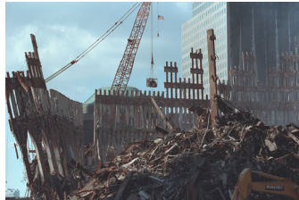
P8049-05 [Hi_j0047_1.JPG] 10/3/2001 VIEWS OF GROUND ZERO
