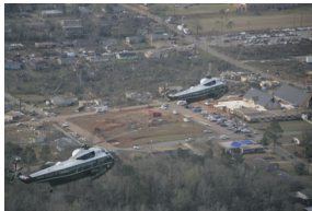
P030307PM-0102 [2025-0073-F_M1Hi_j0157.JPG] 3/3/2007 Aerial tour of tornado damage in Enterprise, Alabama.
