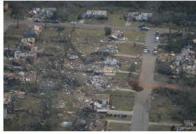
P030307PM-0123 [2025-0073-F_M1Hi_j0199.JPG] 3/3/2007 Aerial tour of tornado damage in Enterprise, Alabama.
