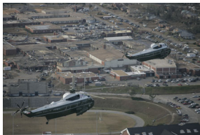
P030307PM-0106 [2025-0073-F_M1Hi_j0165.JPG] 3/3/2007 Aerial tour of tornado damage in Enterprise, Alabama.
