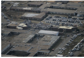
P030307PM-0118 [2025-0073-F_M1Hi_j0189.JPG] 3/3/2007 Aerial tour of tornado damage in Enterprise, Alabama.
