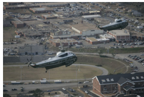
P030307PM-0107 [2025-0073-F_M1Hi_j0167.JPG] 3/3/2007 Aerial tour of tornado damage in Enterprise, Alabama.
