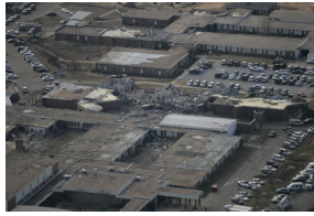
P030307PM-0119 [2025-0073-F_M1Hi_j0191.JPG] 3/3/2007 Aerial tour of tornado damage in Enterprise, Alabama.
