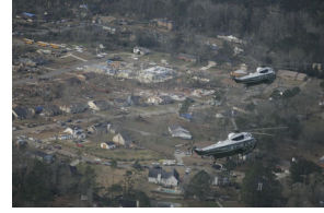
P030307PM-0093 [2025-0073-F_M1Hi_j0139.JPG] 3/3/2007 Aerial tour of tornado damage in Enterprise, Alabama.
