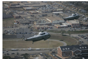
P030307PM-0108 [2025-0073-F_M1Hi_j0169.JPG] 3/3/2007 Aerial tour of tornado damage in Enterprise, Alabama.
