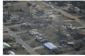
P030307PM-0121 [2025-0073-F_M1Hi_j0195.JPG] 3/3/2007 Aerial tour of tornado damage in Enterprise, Alabama.
