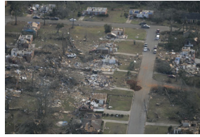
P030307PM-0124 [2025-0073-F_M1Hi_j0201.JPG] 3/3/2007 Aerial tour of tornado damage in Enterprise, Alabama.
