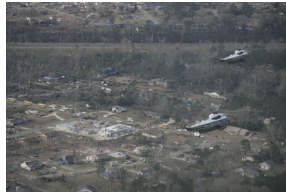
P030307PM-0099 [2025-0073-F_M1Hi_j0151.JPG] 3/3/2007 Aerial tour of tornado damage in Enterprise, Alabama.
