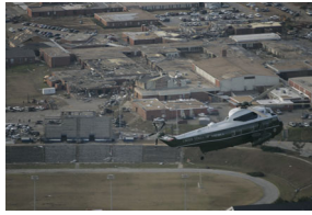
P030307PM-0115 [2025-0073-F_M1Hi_j0183.JPG] 3/3/2007 Aerial tour of tornado damage in Enterprise, Alabama.
