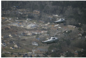
P030307PM-0094 [2025-0073-F_M1Hi_j0141.JPG] 3/3/2007 Aerial tour of tornado damage in Enterprise, Alabama.
