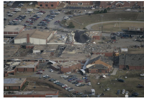
P030307PM-0128 [2025-0073-F_M1Hi_j0209.JPG] 3/3/2007 Aerial tour of tornado damage in Enterprise, Alabama.
