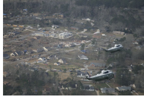
P030307PM-0091 [2025-0073-F_M1Hi_j0135.JPG] 3/3/2007 Aerial tour of tornado damage in Enterprise, Alabama.
