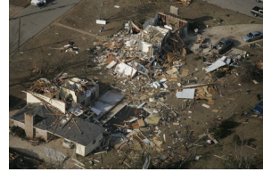
P030307PM-0133 [2025-0073-F_M1Hi_j0219.JPG] 3/3/2007 Aerial tour of tornado damage in Enterprise, Alabama.
