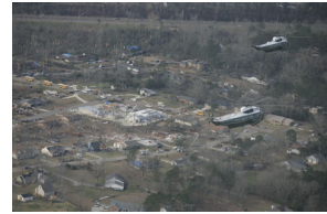
P030307PM-0097 [2025-0073-F_M1Hi_j0147.JPG] 3/3/2007 Aerial tour of tornado damage in Enterprise, Alabama.
