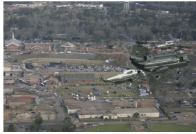
P030307PM-0127 [2025-0073-F_M1Hi_j0207.JPG] 3/3/2007 Aerial tour of tornado damage in Enterprise, Alabama.
