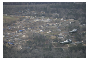
P030307PM-0089 [2025-0073-F_M1Hi_j0131.JPG] 3/3/2007 Aerial tour of tornado damage in Enterprise, Alabama.
