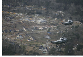
P030307PM-0092 [2025-0073-F_M1Hi_j0137.JPG] 3/3/2007 Aerial tour of tornado damage in Enterprise, Alabama.
