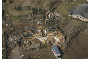
P030307PM-0132 [2025-0073-F_M1Hi_j0217.JPG] 3/3/2007 Aerial tour of tornado damage in Enterprise, Alabama.
