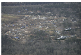
P030307PM-0087 [2025-0073-F_M1Hi_j0127.JPG] 3/3/2007 Aerial tour of tornado damage in Enterprise, Alabama.
